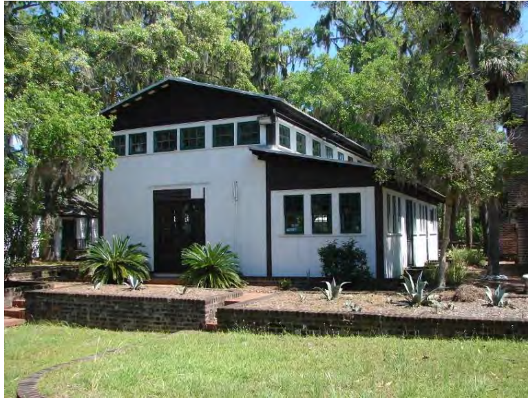
Figure 607. Principal facade of mechanical shop W-1.
