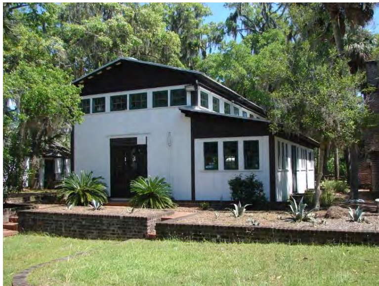
Figure 642. Roebling House precinct gardens.
