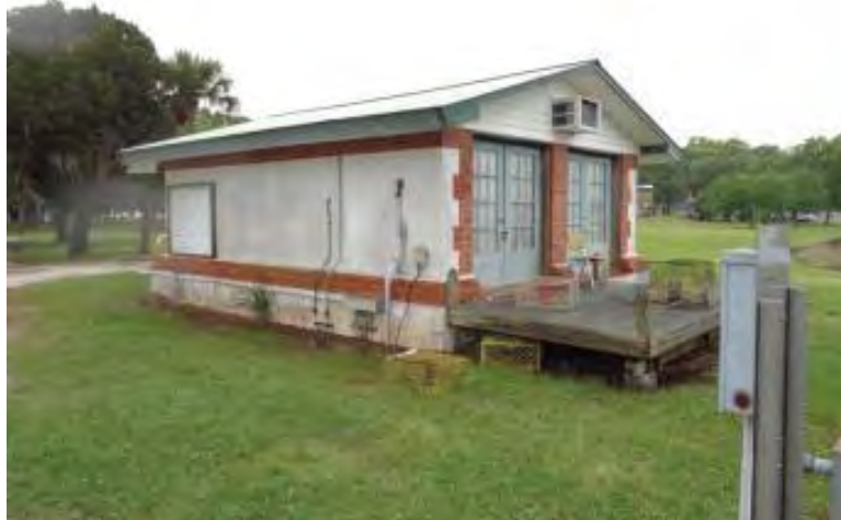
Figure 636. Fuel Oil Storage.
