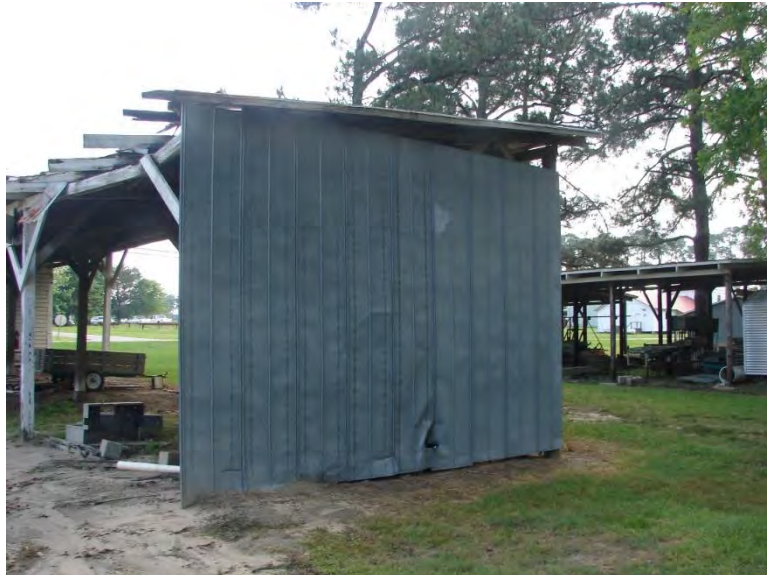
Figure 360. Ag Engineering Equipment Shed, seen far right.
