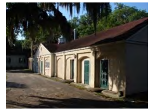
Figure 564. Maintenance and Lab Complex.
