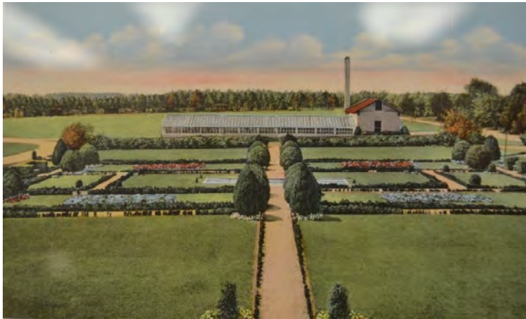
Figure 320. View of the formal garden, greenhouse, and experiment station grounds behind the Tift Building in the 1930s. (Source: University of Georgia Archives)
