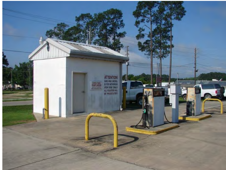
Figure 340. Fuel Monitoring Building.
