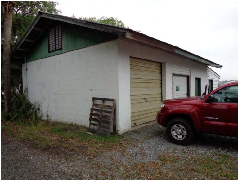
Figure 616. Marine OPS Storage Building.
