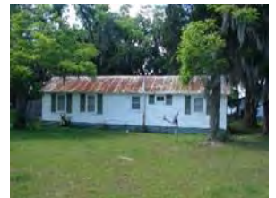
Figure 617. Maintenance Shop 5B.
