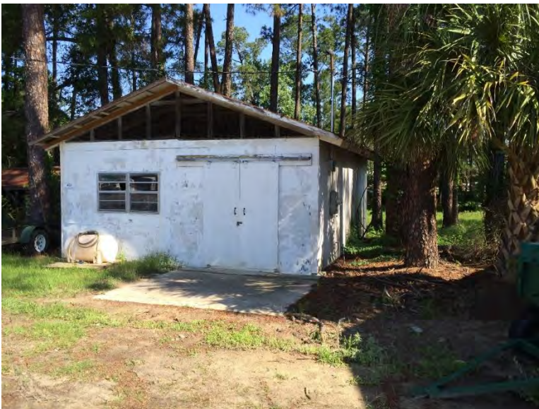
Figure 367. The Plant Pathology Growth Chamber.
