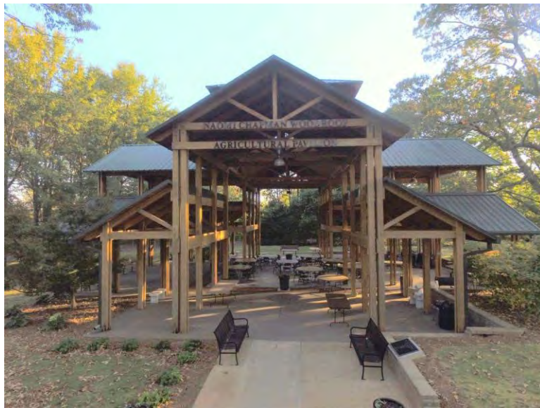
Figure 300. View toward the Woodroof Pavilion, 2015. (Source: University of Georgia)
