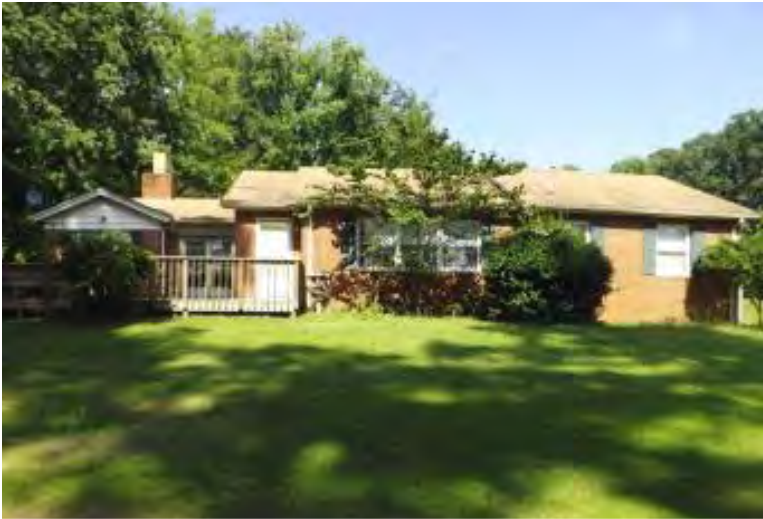
Figure 463. The Resident Jenkins building.
