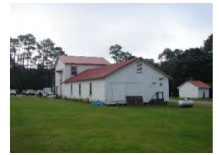
Figure 356. Rear view of the Gin and Seed House.
