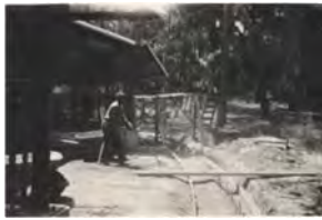
The Cattle Show Barn under construction.
