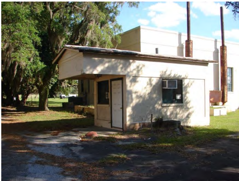
Figure 565. South End Filling Station.
