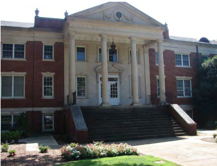
Figure 183. Hoke Smith Building, 2015.
