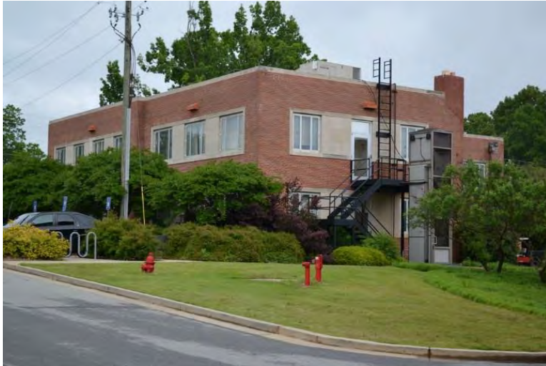
Figure 273. View northwest toward the Cowart Building, 2015.
