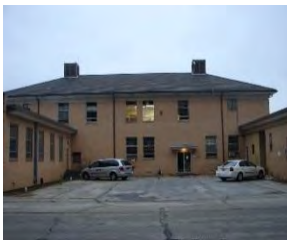
Figure 329. Rear view, Old Administration Building.
