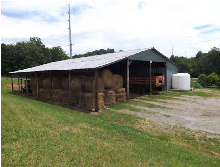
Figure 407. The feed barn.
