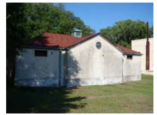
Figure 570. Fuel Storage Building.
