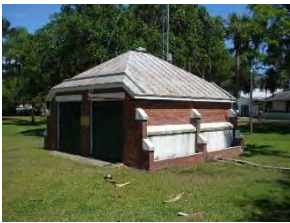
Figure 634. Chemical Storage Building.
