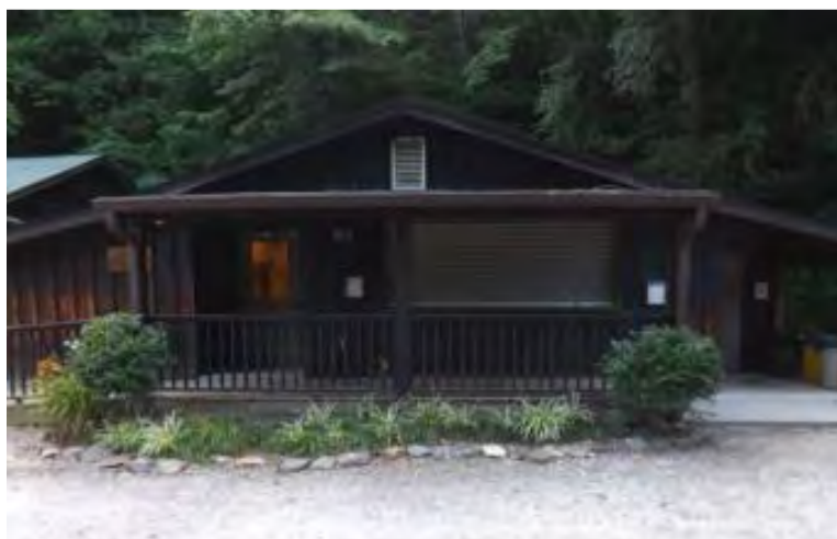
Figure 481. Camp Wahsega craft food storage building.
