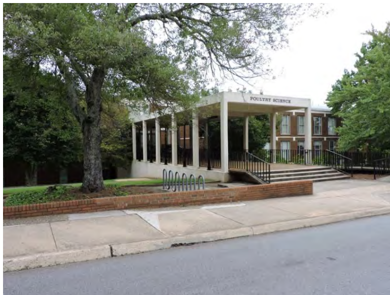
Figure 148. Poultry Science Building, 2015.
