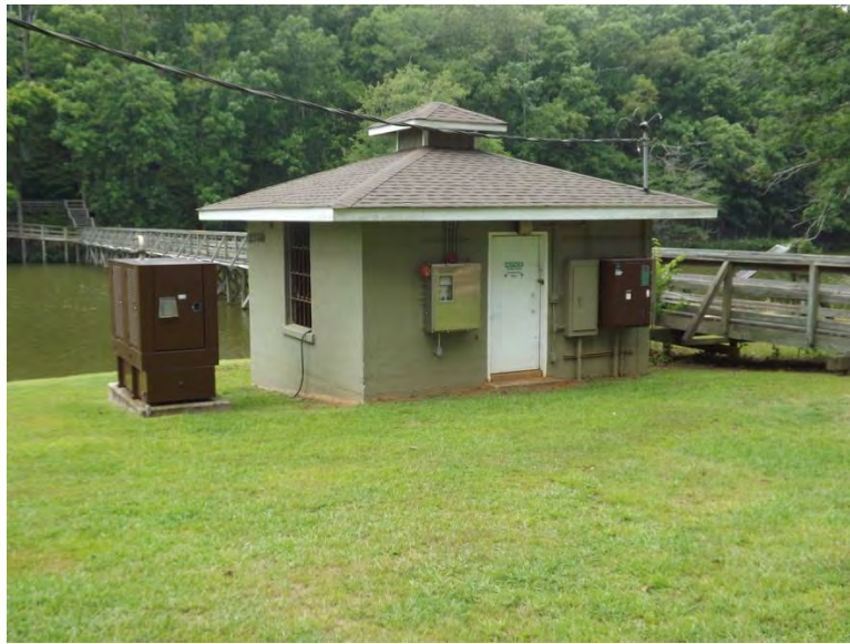
Figure 470. The Sewerage lift station.
