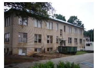
Figure 332. Rear facade, H. H. Tift Building.
