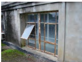
Figure 335. Steel windows at the front of the building.
