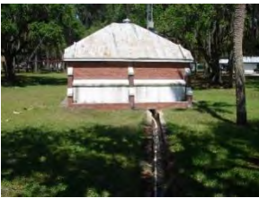
Figure 635. Chemical Storage Building.
