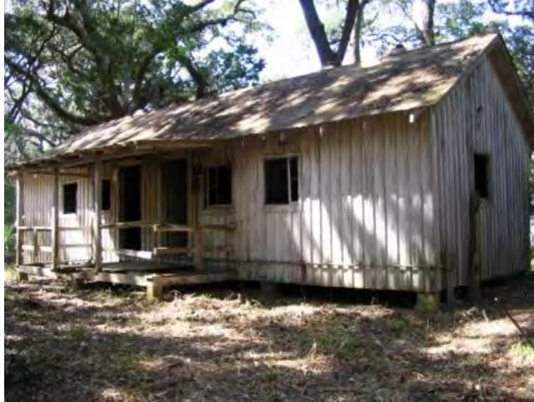
Figure 652. Skidaway Interpretive Cabin.
