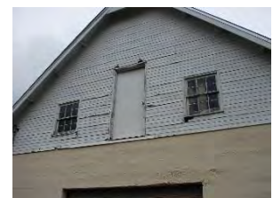
Figure 275. Detail of Mule Barn gable, 2015.
