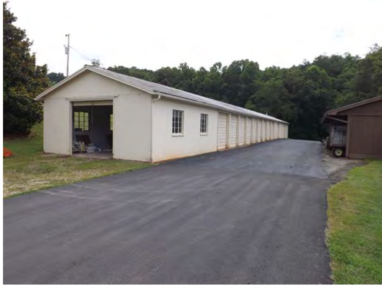
Figure 409. The utility warehouse.
