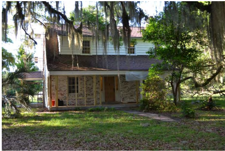
Figure 38. Sears house (UGA 6088) on Sapelo Island. (Source: University of Georgia)
