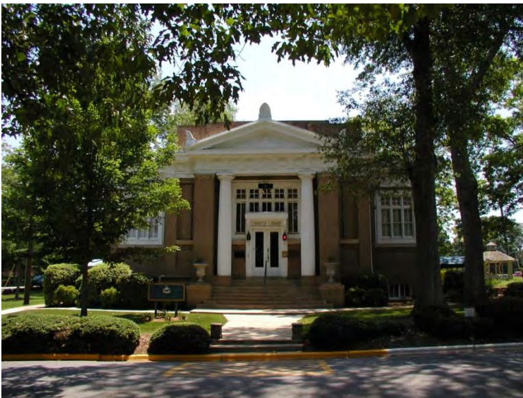
Figure 243. Carnegie Library. (Source: Historic Buildings Preservation Plan)
