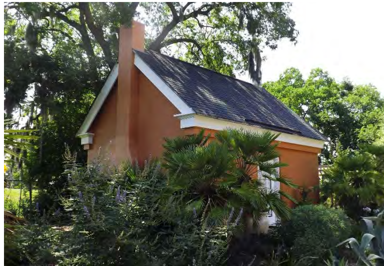
Figure 661. Superintendent's Office, built circa 1919, later Office 15, and now the Bridal Cottage at the Mediterranean Garden. (Source: Coastal Georgia Botanical Gardens, 2013)
