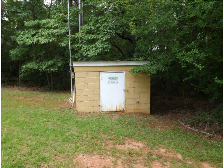
Figure 467. The pump house.
