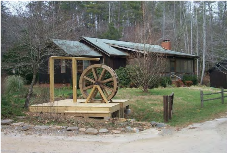
Figure 476. Manager's House/Director's House/Caretaker's House, with water wheel in foreground. (Source: University of Georgia Office of University Architects)
