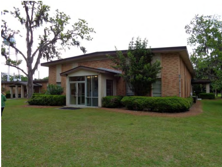
Figure 604. Principal facade of the Roebing Lab.
