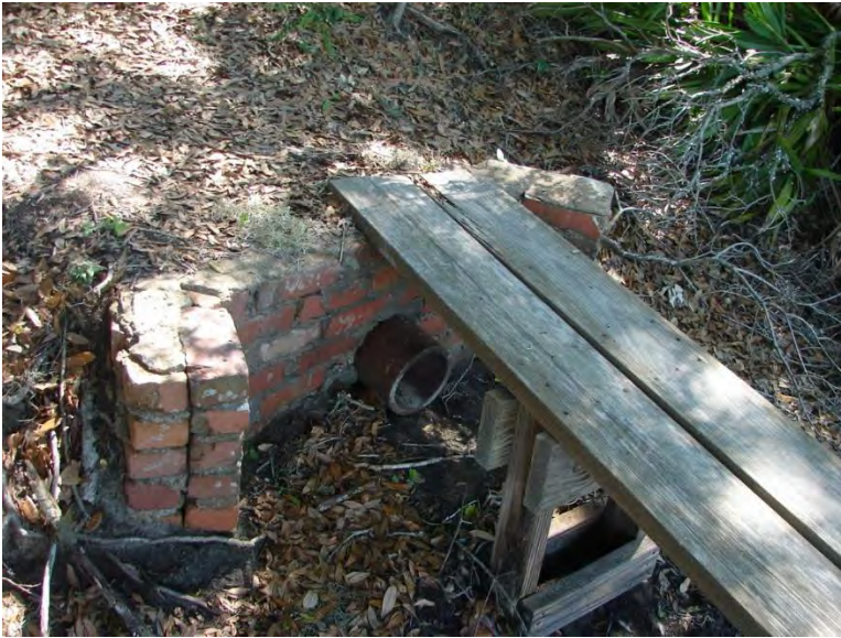
Figure 540. Brick wall and stormwater management system.
