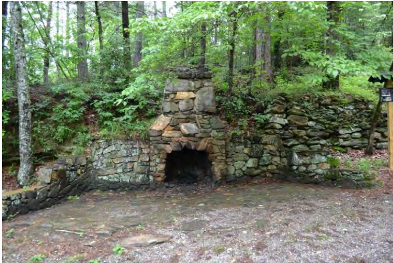
Figure 424. Stone fireplace west of the storage shed.
