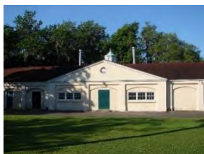
Figure 563. Maintenance and Lab Complex.
