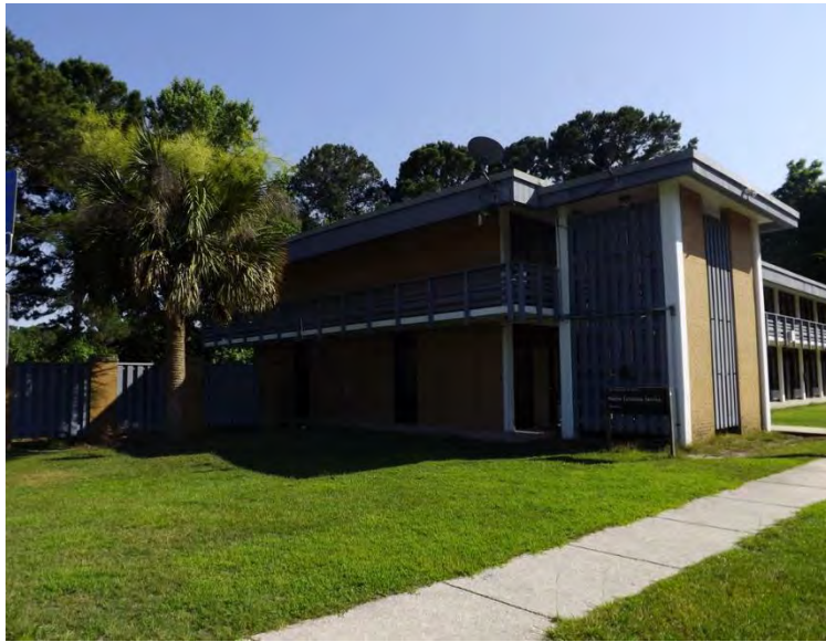
Figure 647. UGA MAREX Dormitory.
