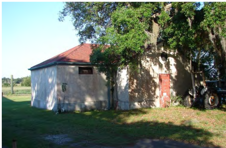
Figure 569. Fuel Storage Building.
