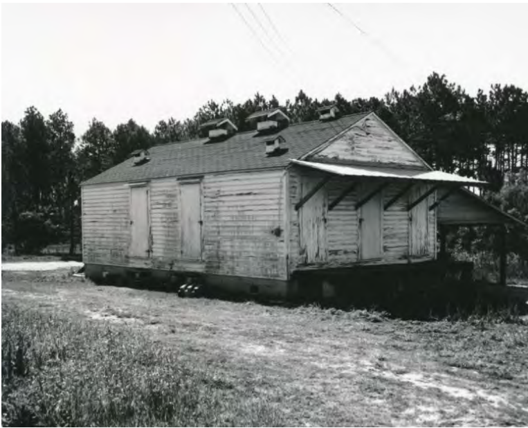
Figure 352. Undated historic photo of the Potato Curing House. (Source: b63)
