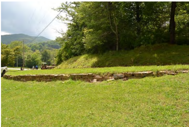
Figure 400. Entrance road retaining wall.
