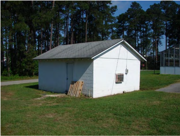
Figure 364. ARS Storage Building.
