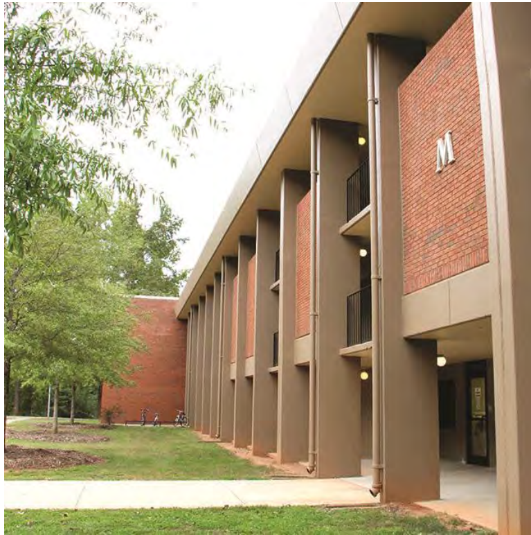
Figure 212. Rogers Road apartments. (Source: University of Georgia)
