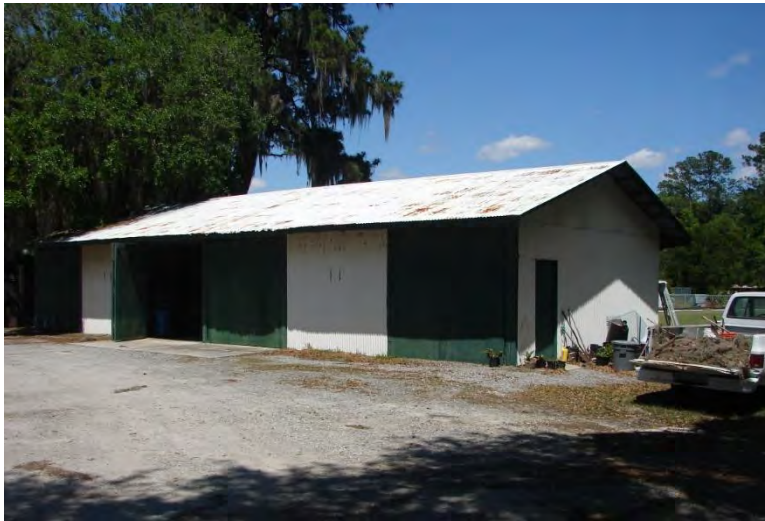
Figure 637. Maintenance Shop B.
