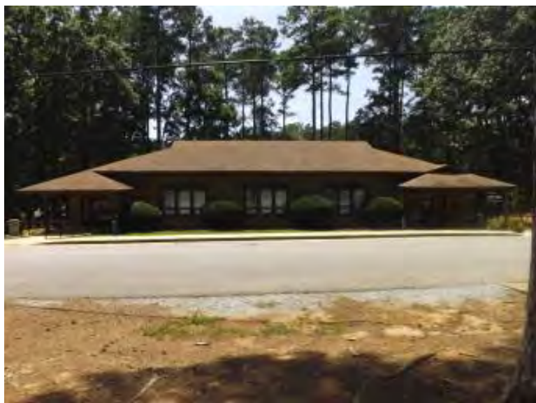
Figure 453. The Callaway Building.
