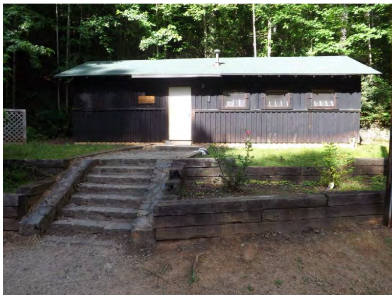
Figure 488. Camp Wahsega boys' bathhouse.
