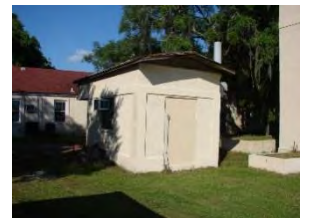
Figure 566. South End Filling Station.
