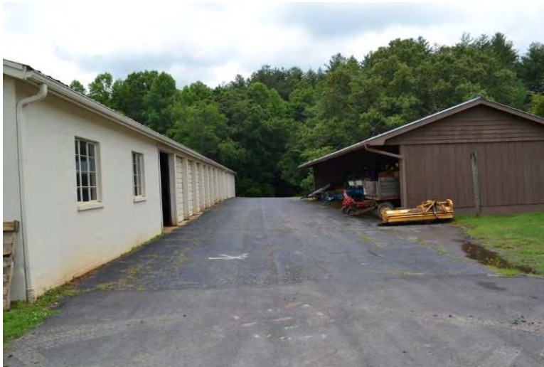
Figure 411. The maintenance vehicle shed.
