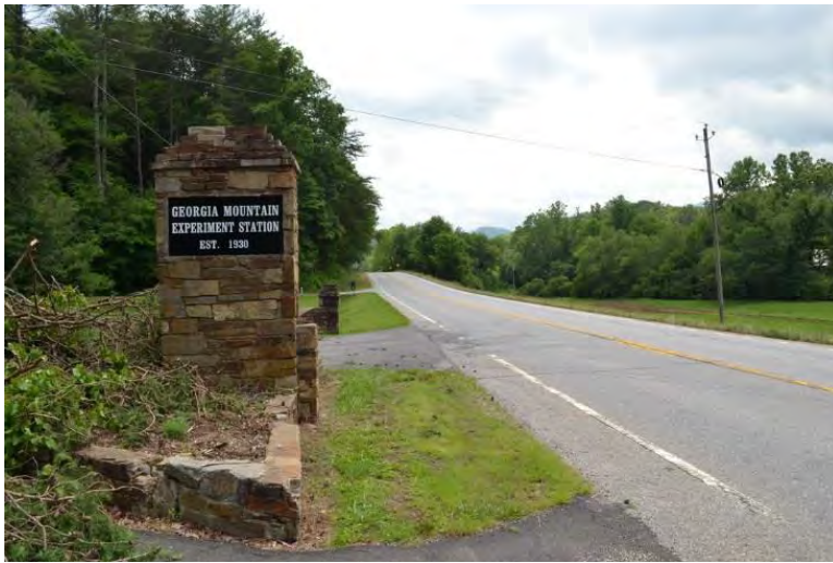
Figure 399. Stone walls and entry piers.
