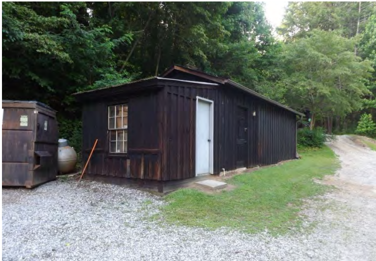
Figure 482. Camp Wahsega pump house.
