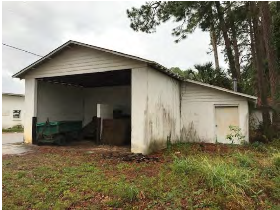
Figure 378. Soil Sterilizer Shed. (Source: University of Georgia)
