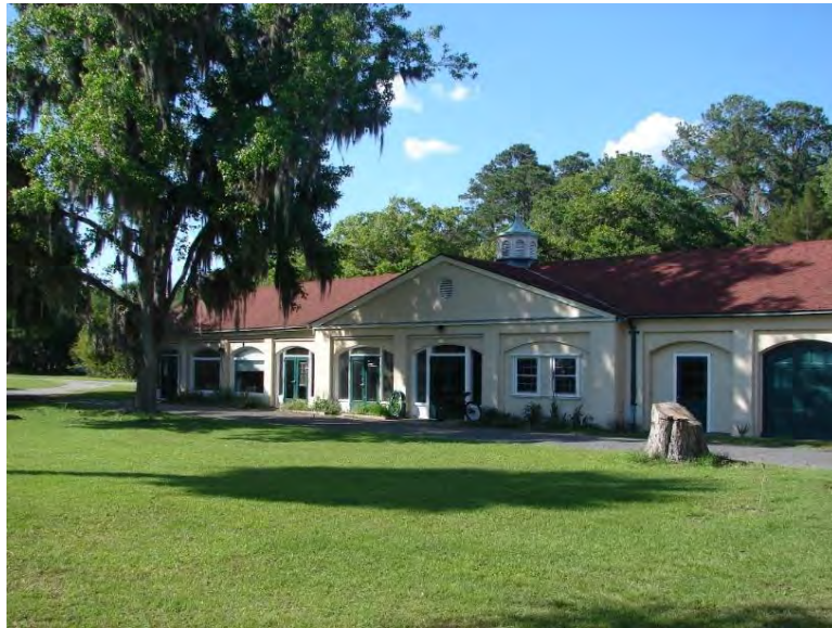
Figure 562. Maintenance and Lab Complex.
