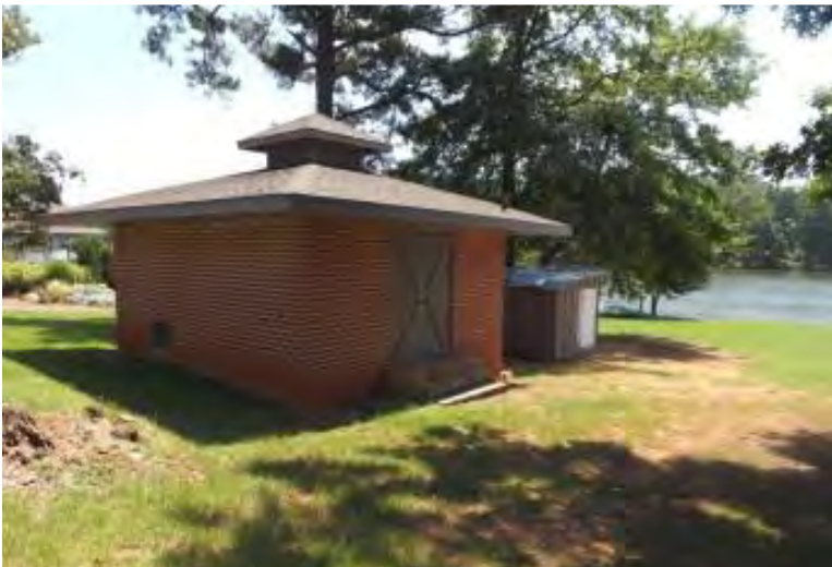
Figure 464. Pool 1 Filter House.
