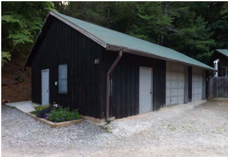
Figure 486. Camp Wahsega shop building.
