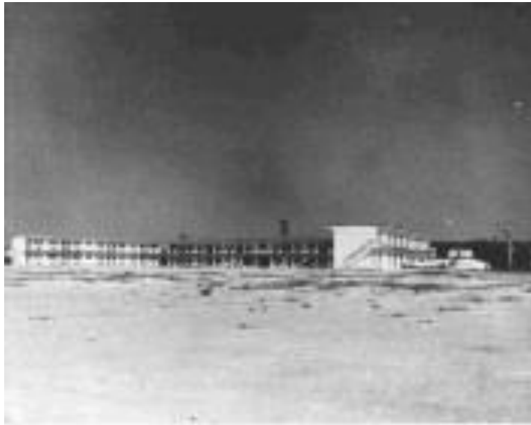
Figure 437. Dolphin Club and Hotel, 1959. (Source: University of Georgia 4-H)
