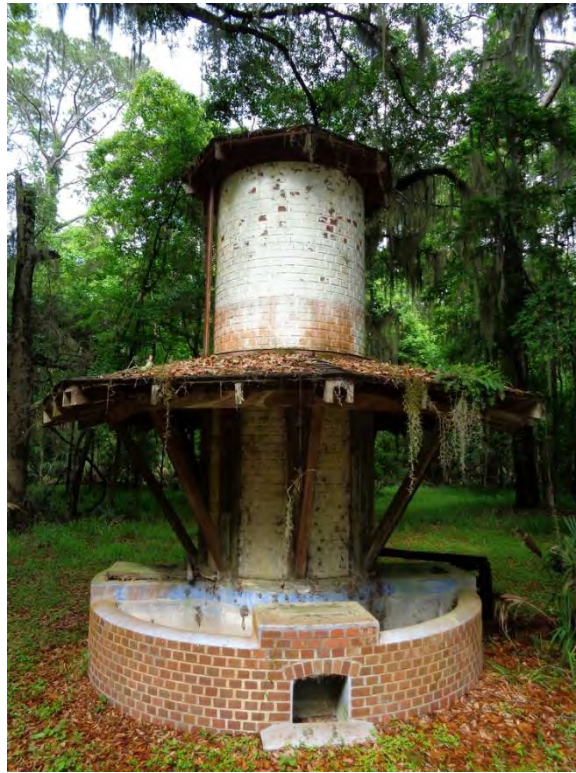
Figure 650. Livestock watering trough.
