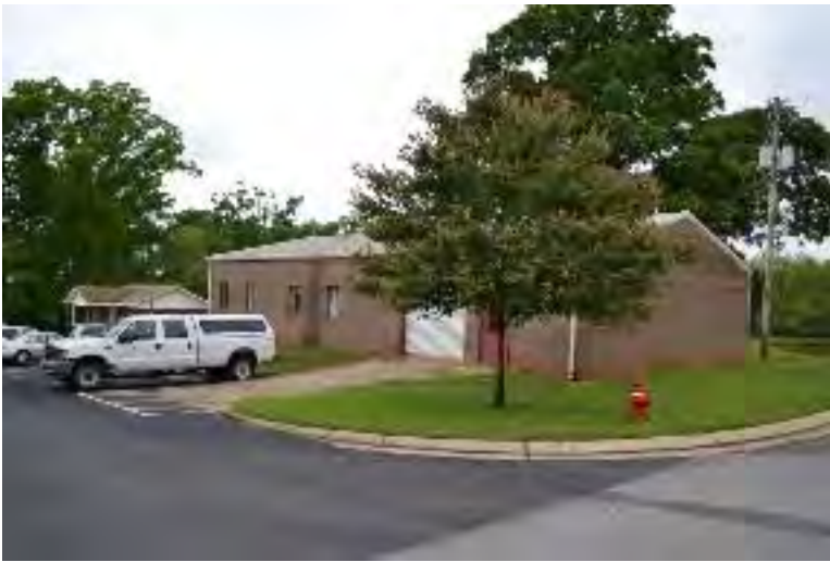
Figure 307. View northwest of the Redding Annex, 2015.
