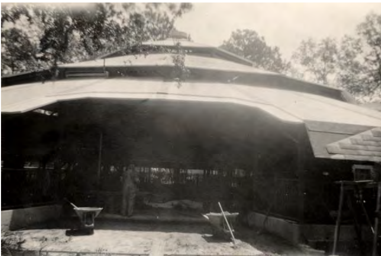
Figure 593. Cattle Show Barn under construction. (Source: Skidaway Oceanographic Institute)
