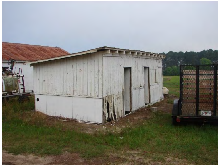
Figure 384. The Fuel House.
