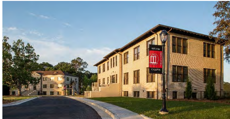
Figure 333. View of Animal and Dairy Science Building (left) and H. H. Tift Building (right). (Source: University of Georgia, Office of the University Architects)
