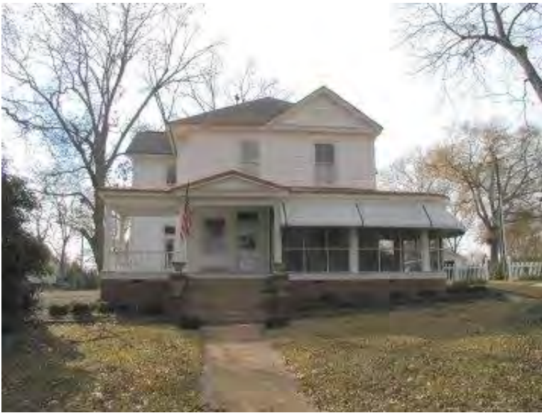
Figure 238. Former President's Cottage. (Source: Historic Buildings Preservation Plan)
