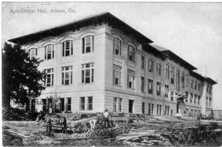
Figure 30. Conner Hall under construction. (Source: University of Georgia Extension.)
