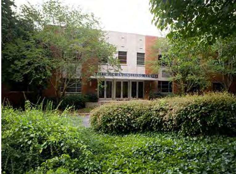
Figure 202. Driftmier Engineering Center. (Source: University of Georgia)
