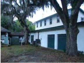
Figure 605 Mechanical Shop W-1.
