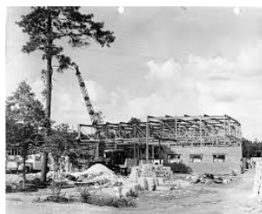
Construction of Rock Eagle 4-H Camp.
