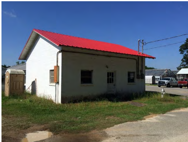
Figure 369. The Grass Br Headhouse and Greenhouse.
