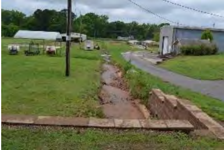
Figure 310. View south of one of the stormwater management channels, 2015.
