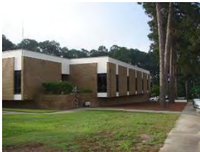
Figure 338. The General Research Building is located southwest of the H. H. Tift and Animal and Dairy Science Buildings.
