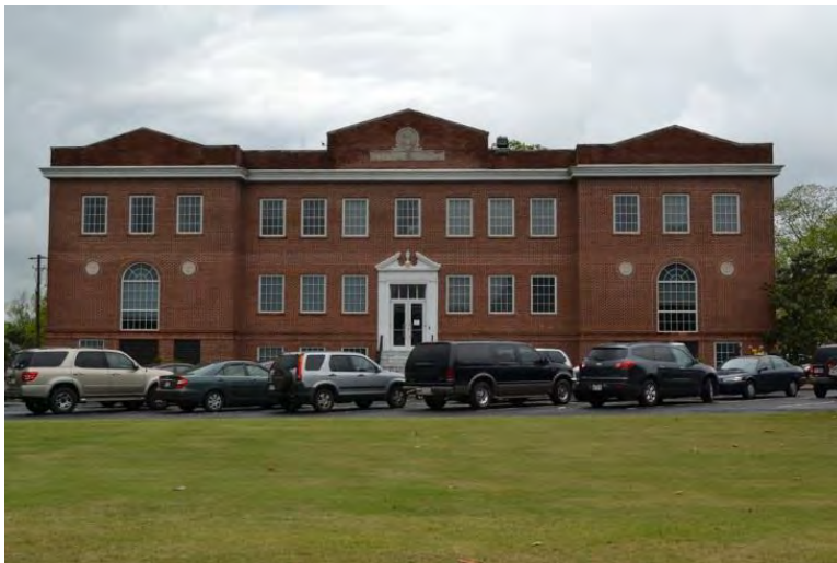
Figure 270. View toward the principal facade of Flynt, 2015.
