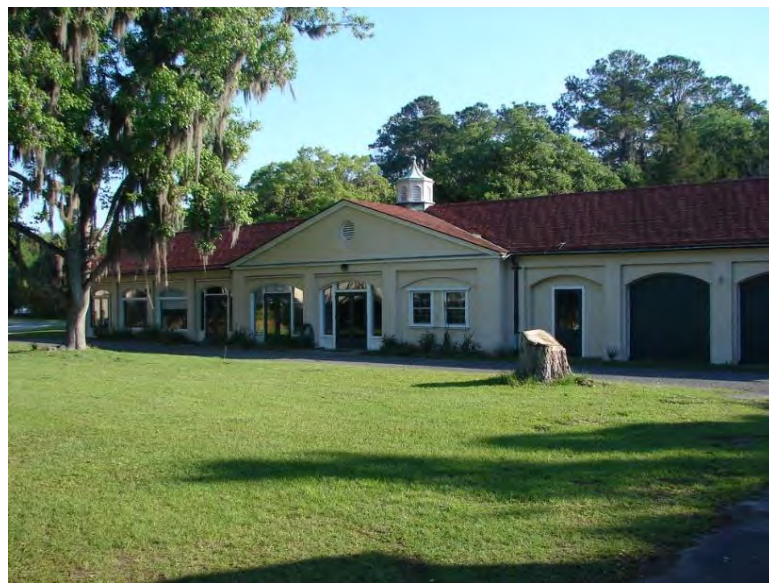
Figure 558. South End Office Building.
