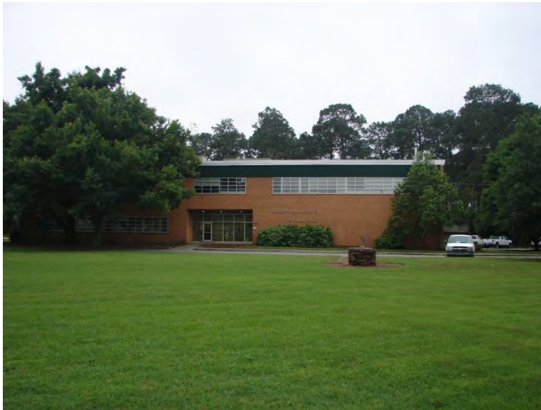
Figure 336. Front view of the Horticulture Building, 2015.
