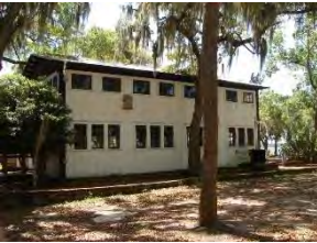
Figure 606. Mechanical Shop W-1
