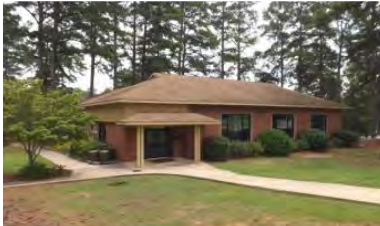
Figure 451. The Hastings Building.
