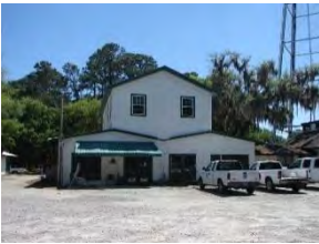
Figure 608. Mechanical Shop W-1.
