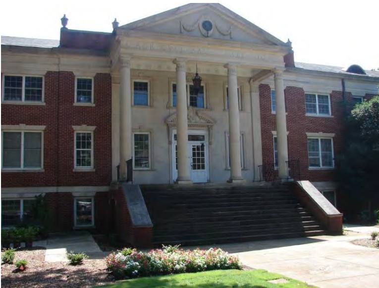
Figure 183. Hoke Smith Building, 2015.
