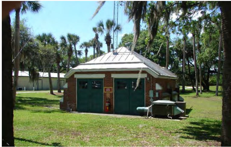
Figure 633. Chemical Storage Building.
