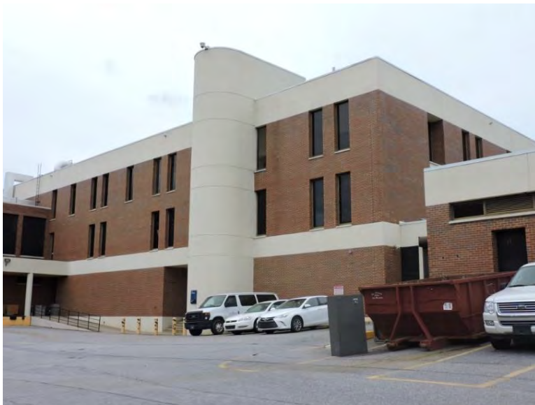
Figure 197. Veterinary School complex, 2015.
