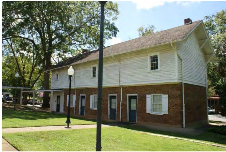
Figure 223. The carriage house, 2015.
