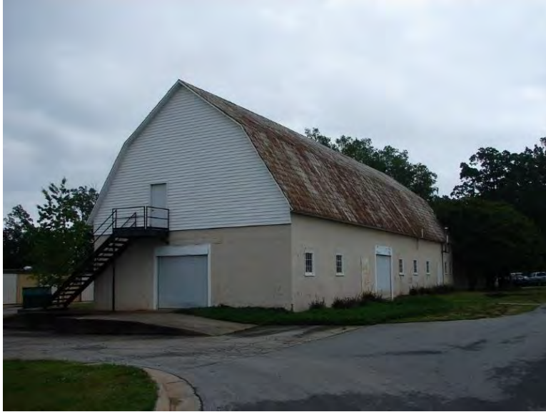
Figure 279. Research Services Building and Dairy Barn, west end, 2015.
