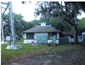
Figure 609. Mechanical Shop W-1.
