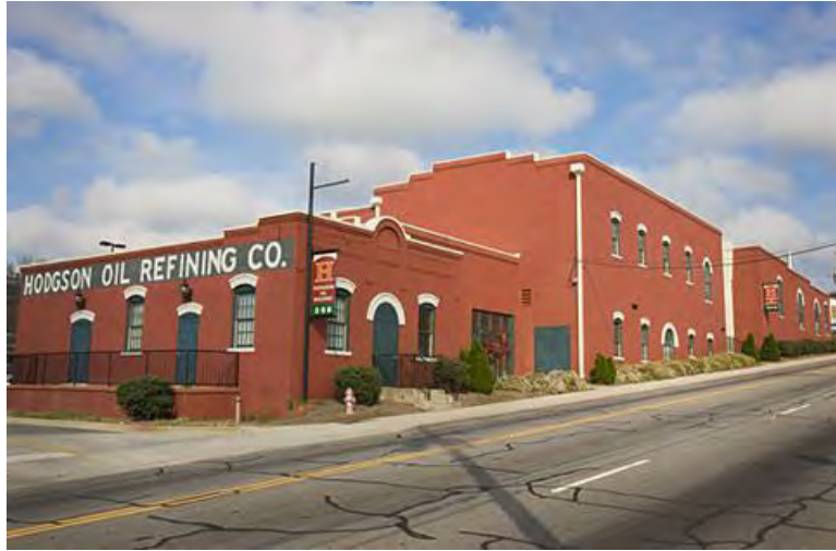
Figure 94. Hodgson Oil Refinery building. (Source: University of Georgia)
