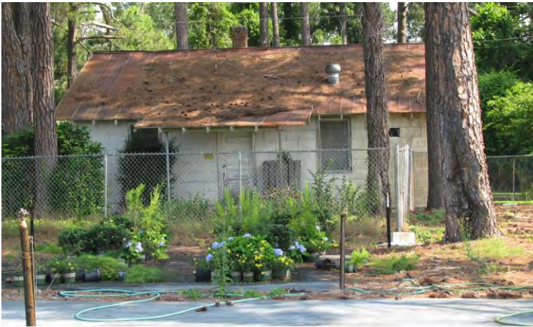
Figure 371. Laborers Cottage A.
