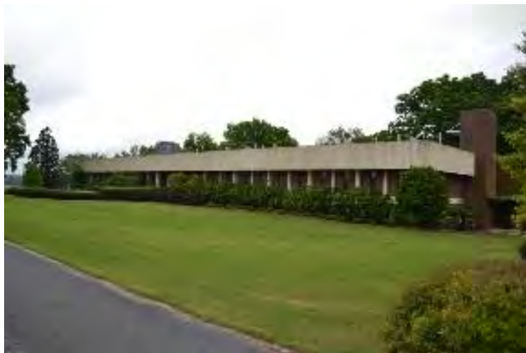
Figure 306. View southwest toward the Redding Building, 2015.
