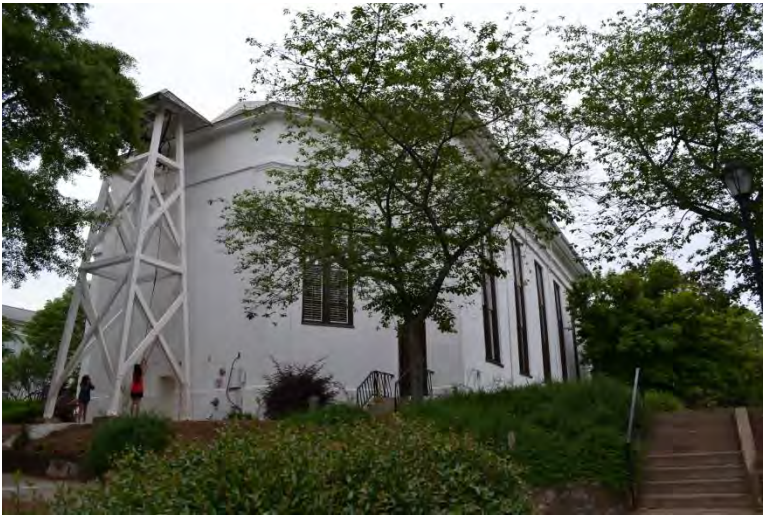
Figure 76. The bell tower, 2015.
