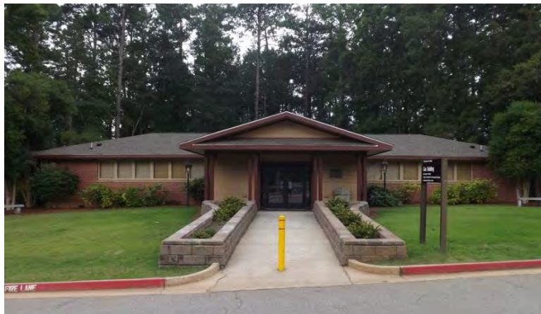
Figure 457. L.P. Gas Building.
