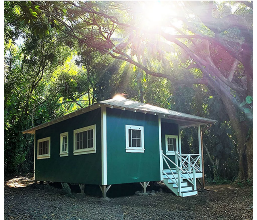
Montgomery House, Hā'ena State Park, Kaua'i. Photo by MASON
