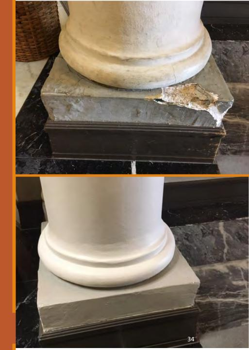
Ali'iōlani Hale, Honolulu, O'ahu. Damaged plaster on columns were repaired with in-kind materials.
