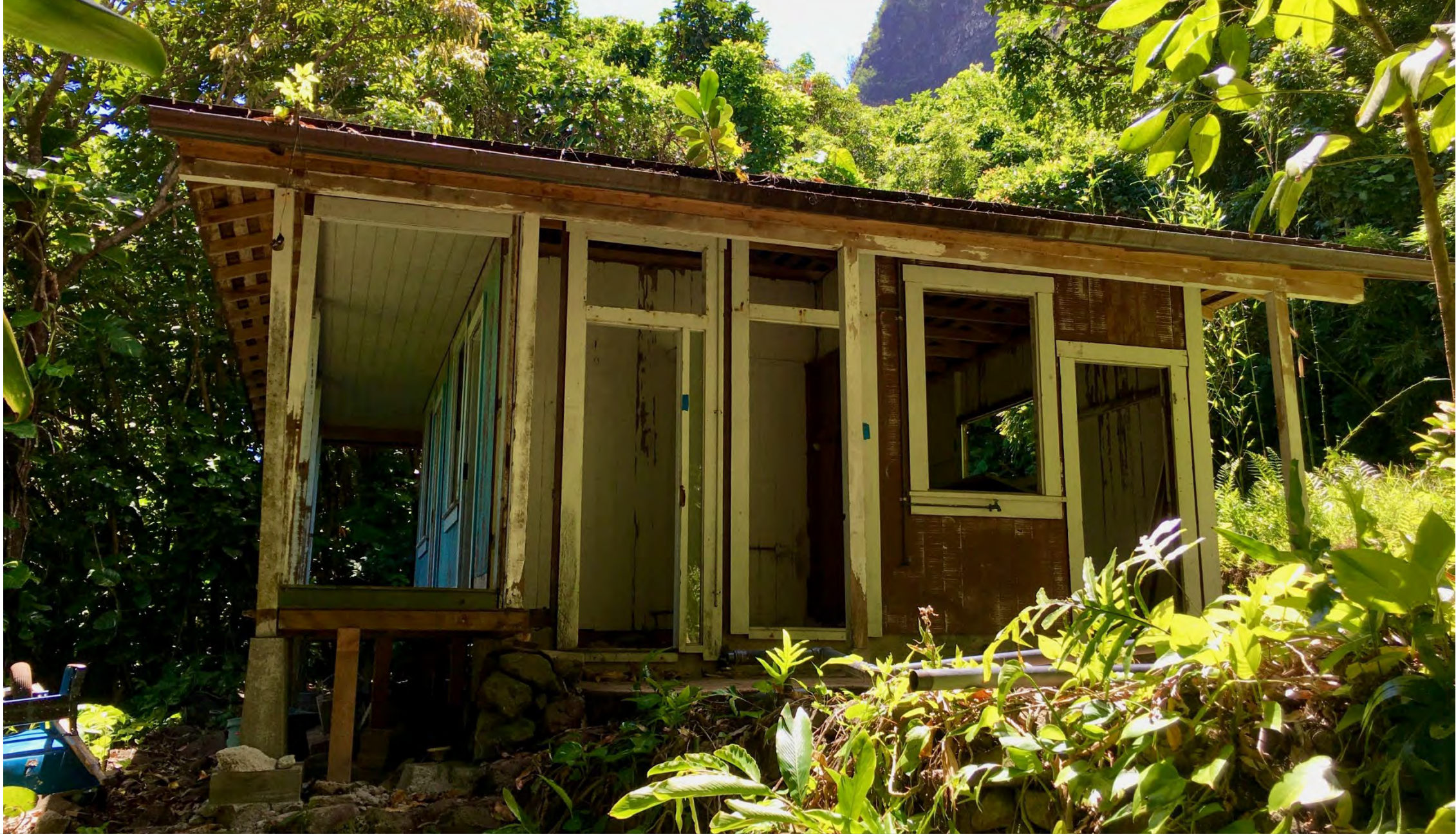
ALLERTON CARETAKER'S COTTAGE BEFORE
