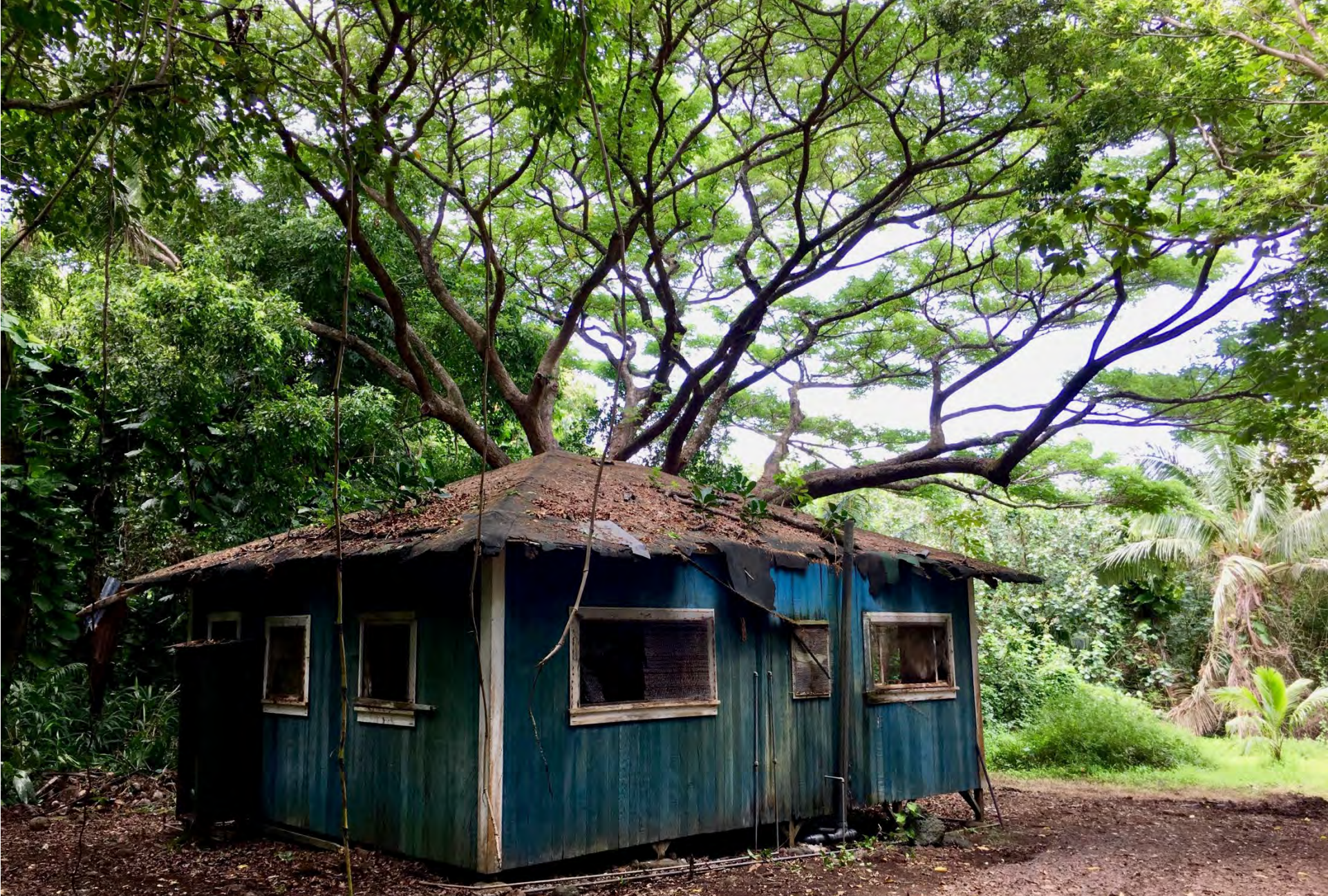
MONTGOMERY HOUSE BEFORE
