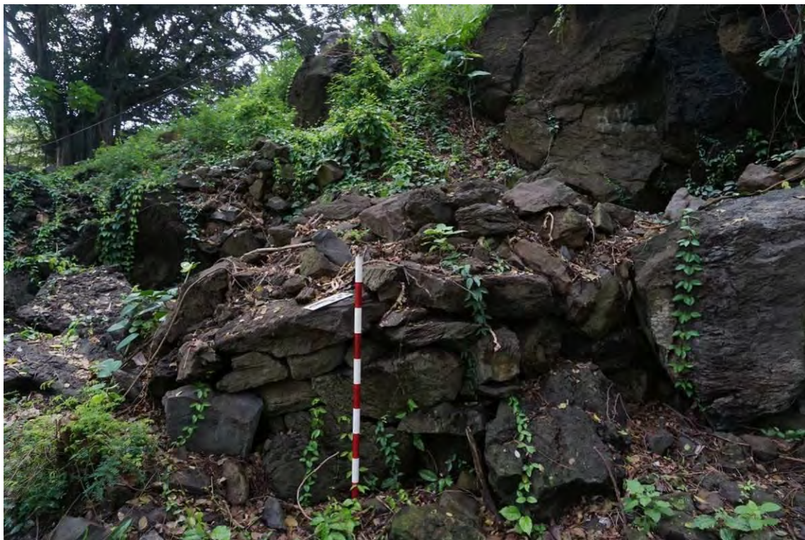
Figure 33. Photos of SIHP # -08768, Feature C and Feature D (enclosure, top photo) and close-up of Feature C (east arm of enclosure, bottom photo), view to southeast
