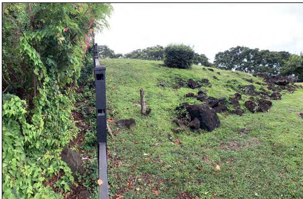
Figure 53. Photo showing a large feature atop a relatively flat hillside on Mid-Pacific Institute property, which Feature M connects to, view to east
