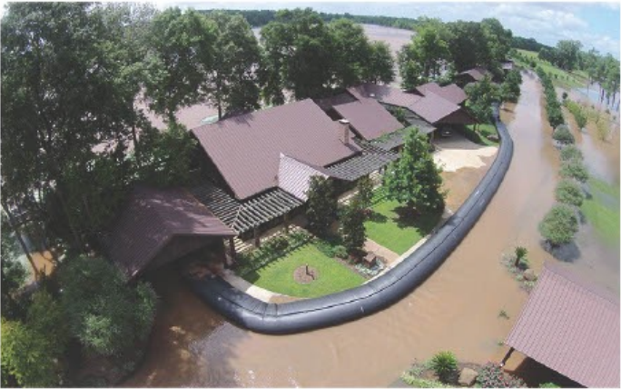
Temporary water-filled barriers are designed to keep areas protected from flood water.
