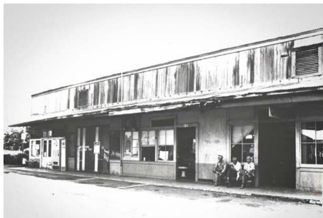
1960's Takahashi Building. Photo: Nancy Bannick
