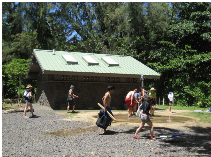
Photo 18 – New Comfort Station and Showers
