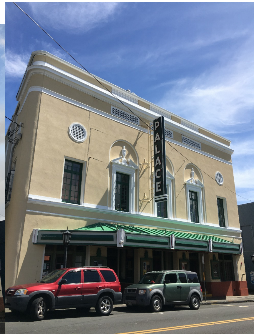
The Palace Theater in Hilo, Hawai'i Island before (left) and after exterior restoration.
