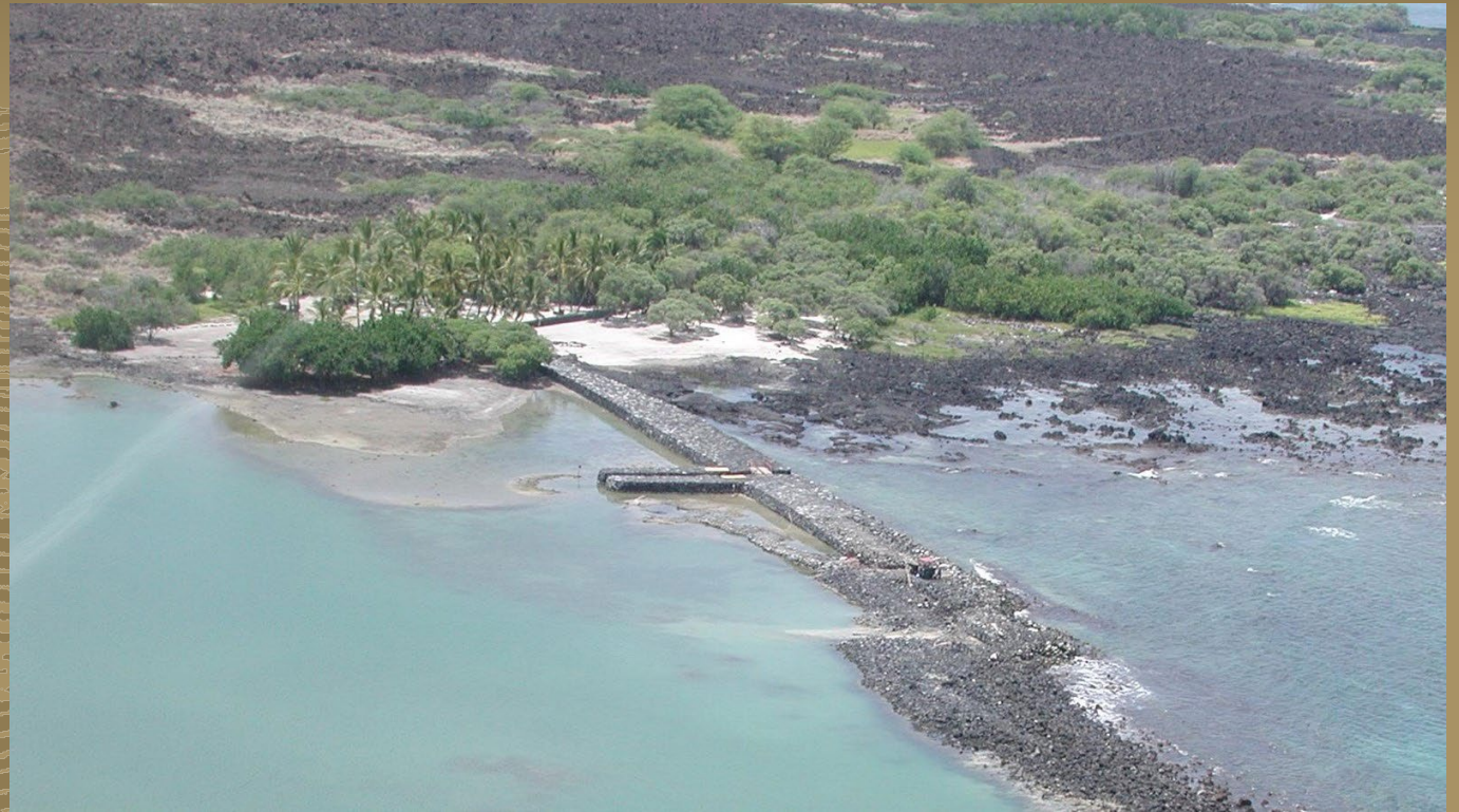
Rehabilitation of the 780-feet of the Kaloko Fishpond Wall, Hawaii
