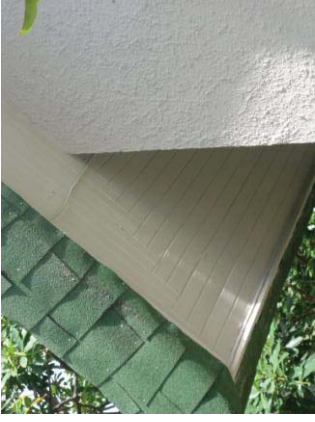
Closed or boxed eaves are enclosed by boards and/or molding so that the rafters are not visible.
