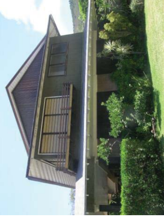
Closed or boxed eaves are enclosed by boards and/or molding so that the rafters are not visible.
