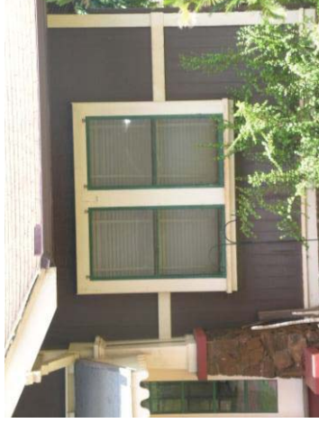
If sash windows slide in a vertical plane, they are double-hung windows and may be hung as a single, pair, or set of three.
