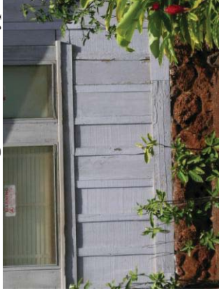
Board-and-batten is lapped siding.
