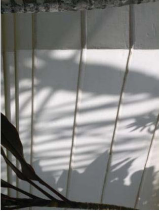
Drop siding has a simple channel
