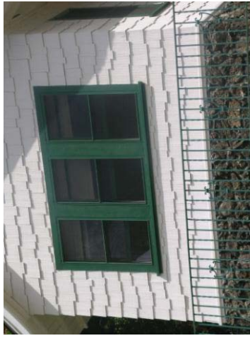
If sash windows slide in a vertical plane, they are double-hung windows and may be hung as a single, pair, or set of three.
