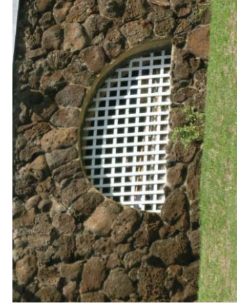
Lattice foundation vent
