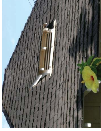
Wood slat attic vent
