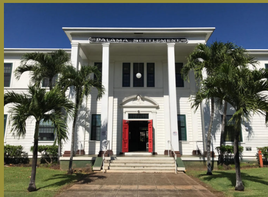
Pālama Settlement, Honolulu, O'ahu
