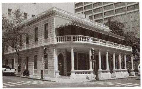
Kamehameha V Post Office (1871), Bethel and Merchant Streets, Honolulu Hawai'i's first all-concrete building, the Kamehemeha V Post Office was built by J.G. Osborne in 1871 using pre-cast concrete blocks reinforced with iron bars. Its successful use of concrete led to the building of other concrete structures, including the original Royal Hawaiian Hotel in 1872. Photo by Jon Radke.
