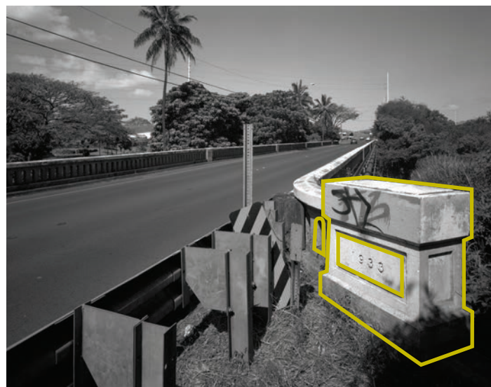
Clockwise from the top left: Two of the original end stanchions, the bridge deck, arched voids, a balustrade stanchion with expansion joint, and an original end stanchion. These elements are outlined in yellow.
