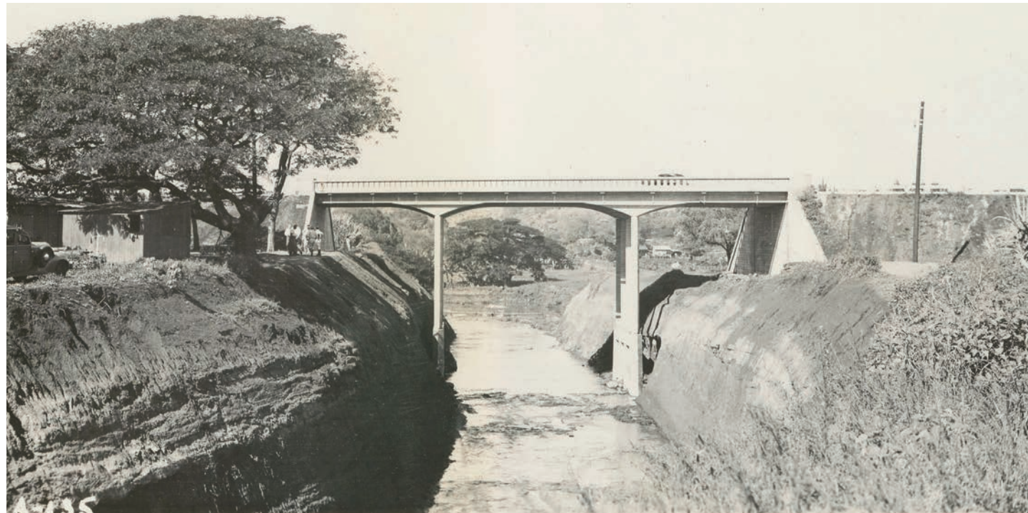
Waikele Canal Bridge, ca. 1940 National Archives, ID 169139914
