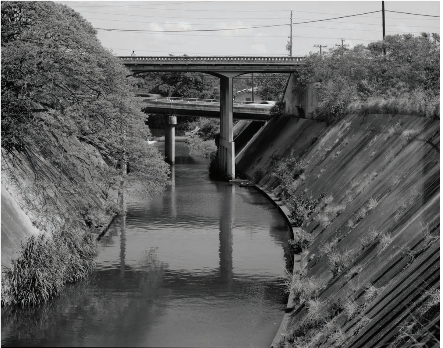
Waikale Canal Bridge, 2012 David Franzen, Hawai'i State Archives
