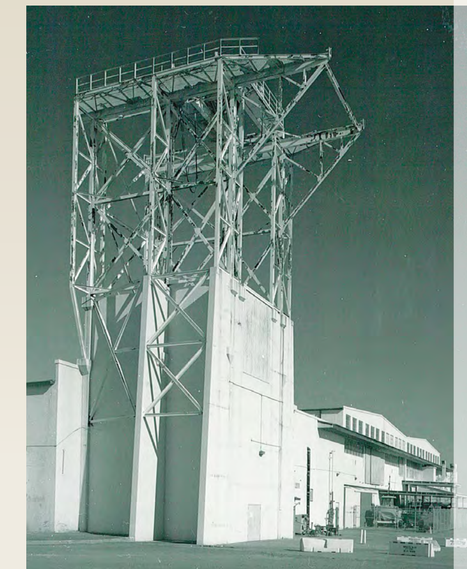
Franzen Photography, HAER No. HI-86-7
