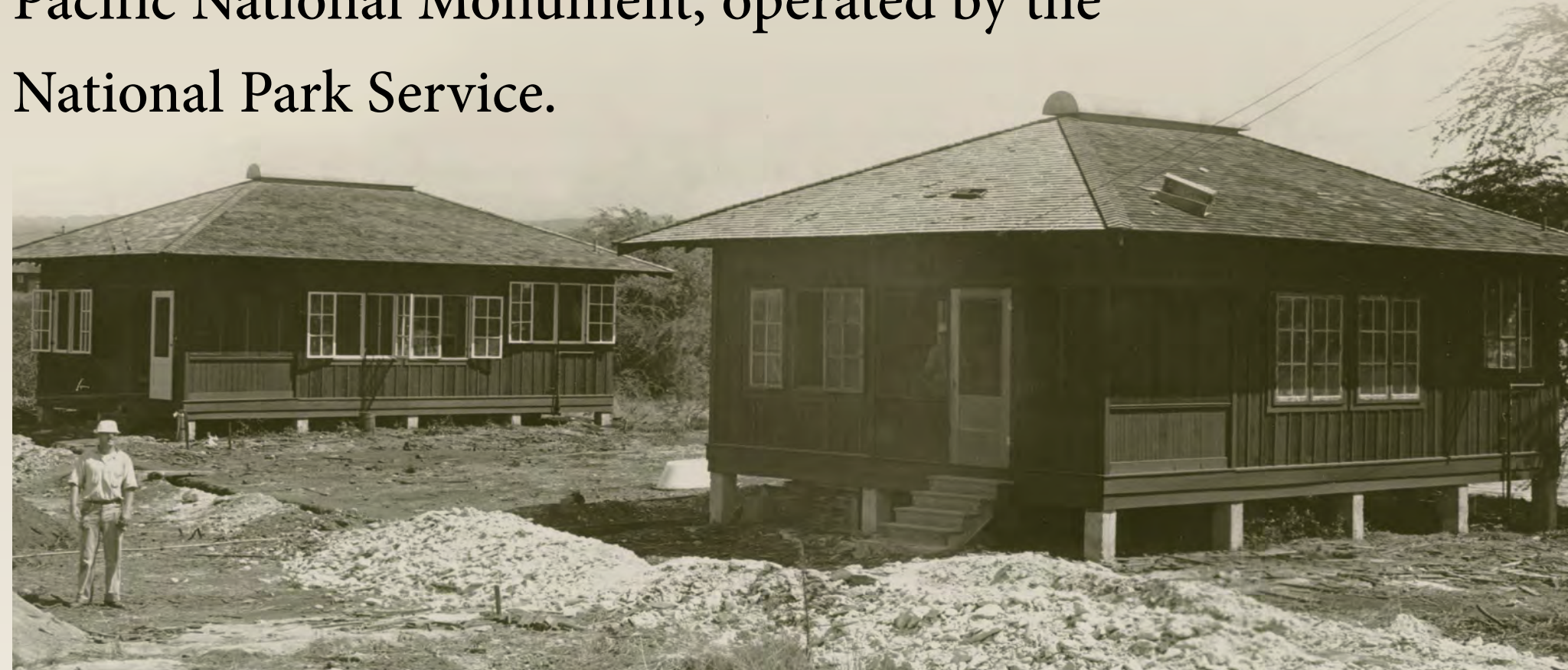
Two CPO houses under construction in October 1923.
