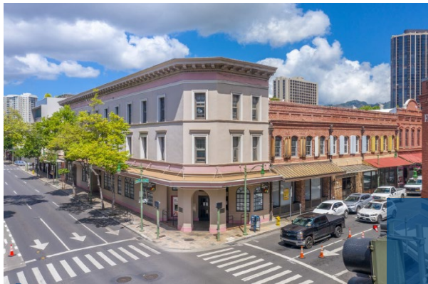
Hocking Building Originally Built in 1914.
