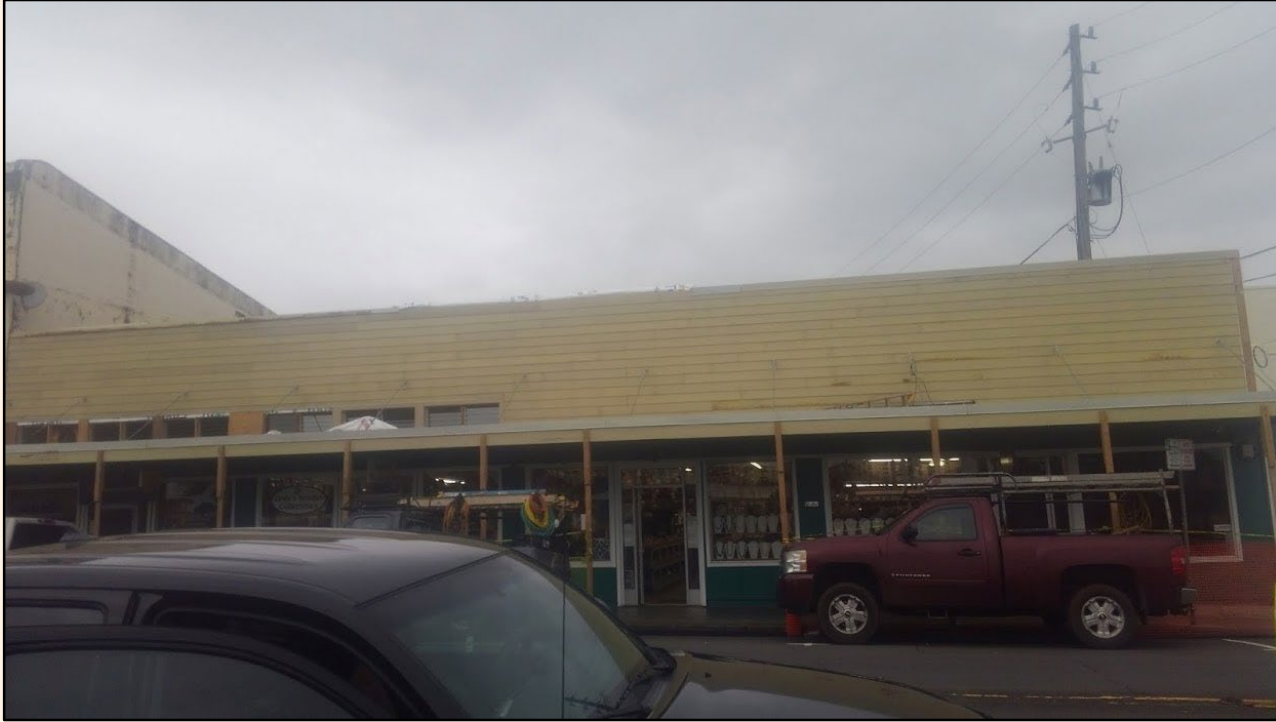
Repaired front façade, roof leaks and exterior painting (2019).
