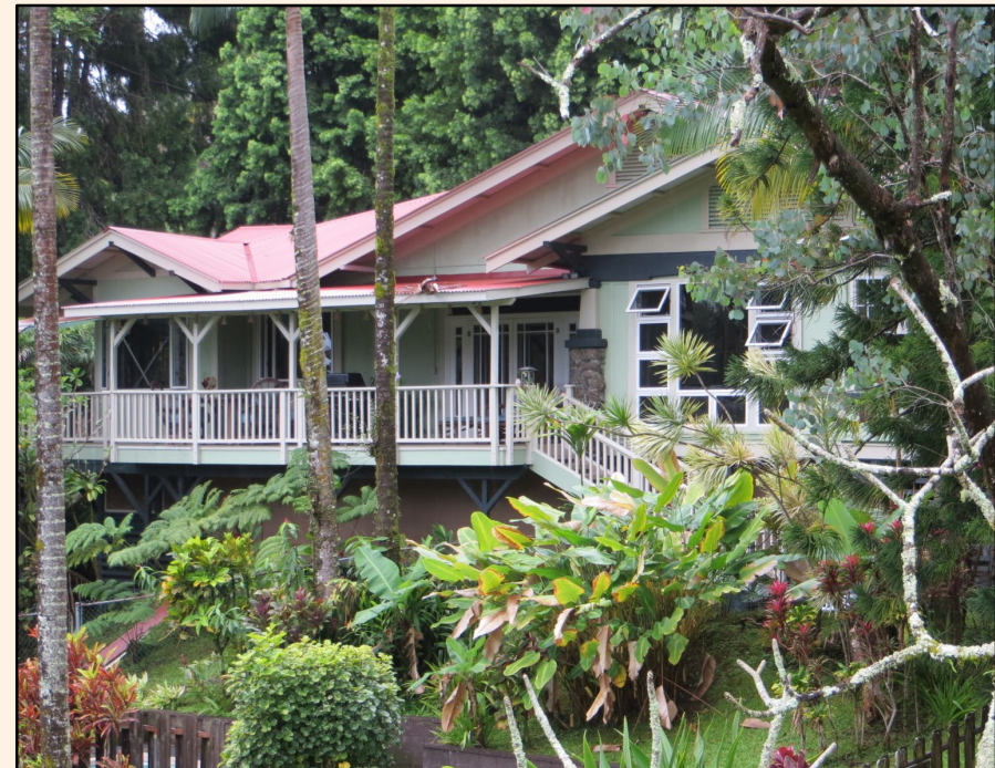
Henderson residence, Hilo. Photo courtesy of Historic Hawai'i Foundation
