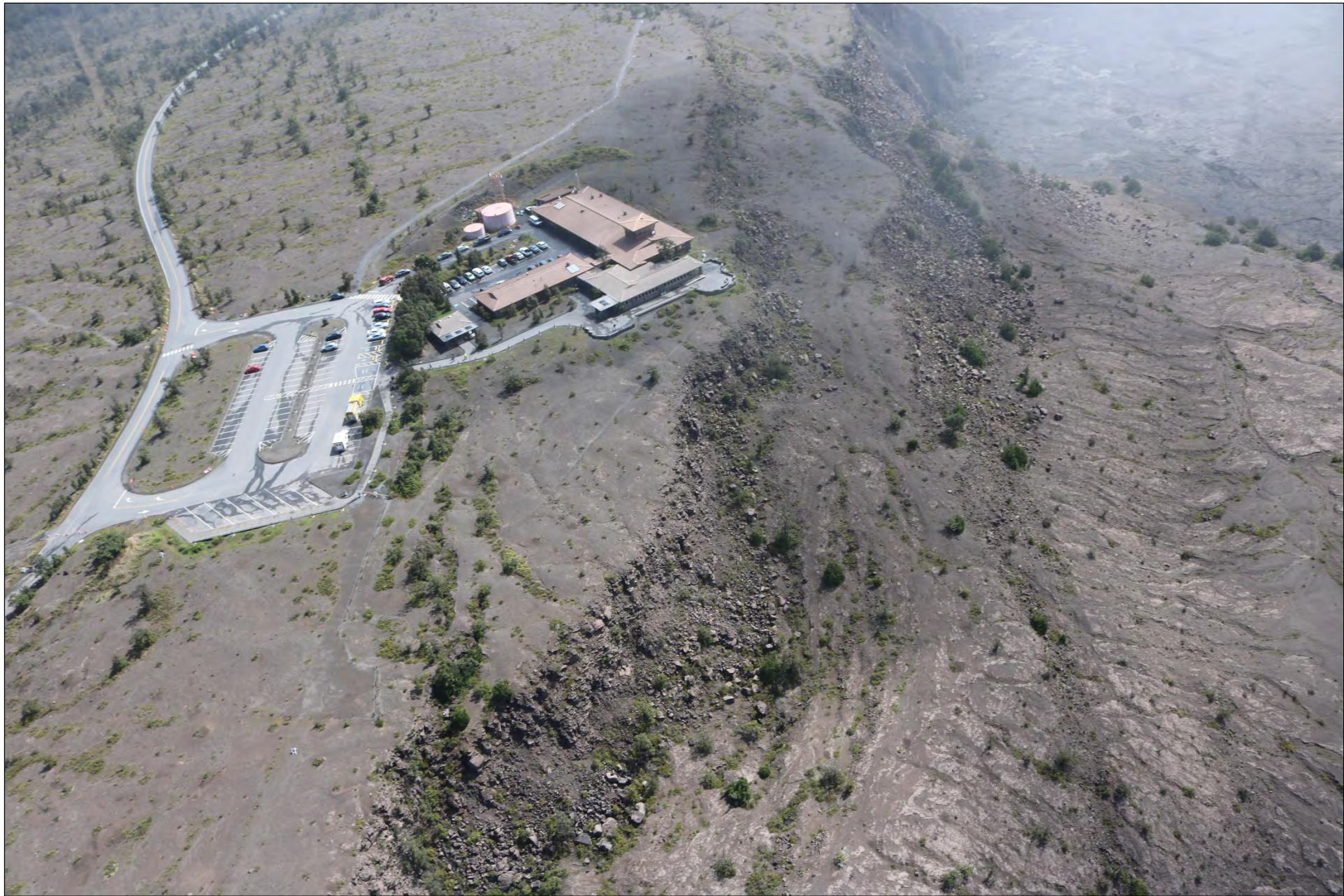
Uēkahuna Bluff, including Jaggar Museum and the USGS-operated Reginald T. Okamura facility and equipment, May 2018. Photo NPS.
