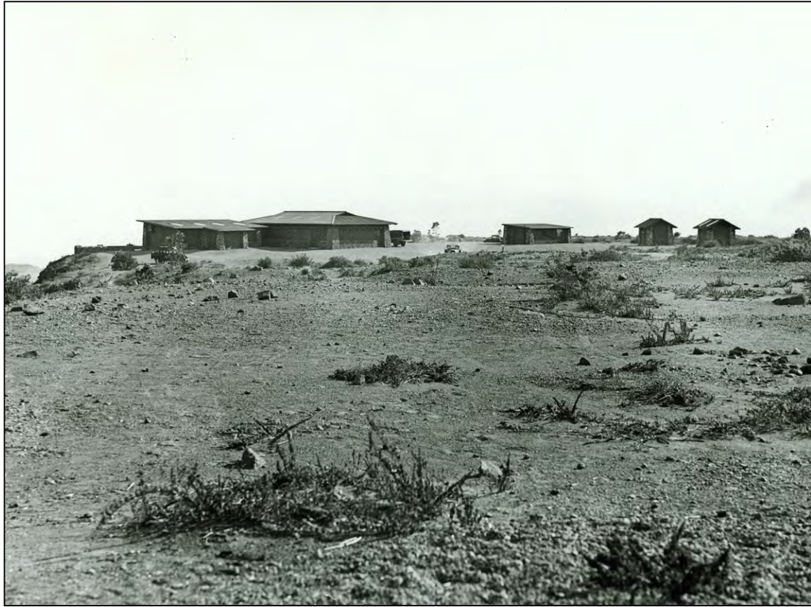
Naturalist Building, Lecture Hall, Geo-chemical and HVO Office, Comfort Stations ca. 1930
