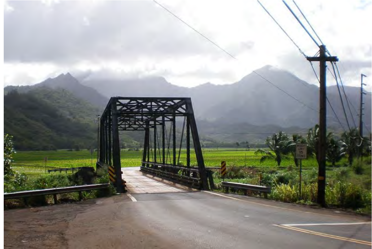
Hanalei Bridge. Photo by Joel Bradshaw.
