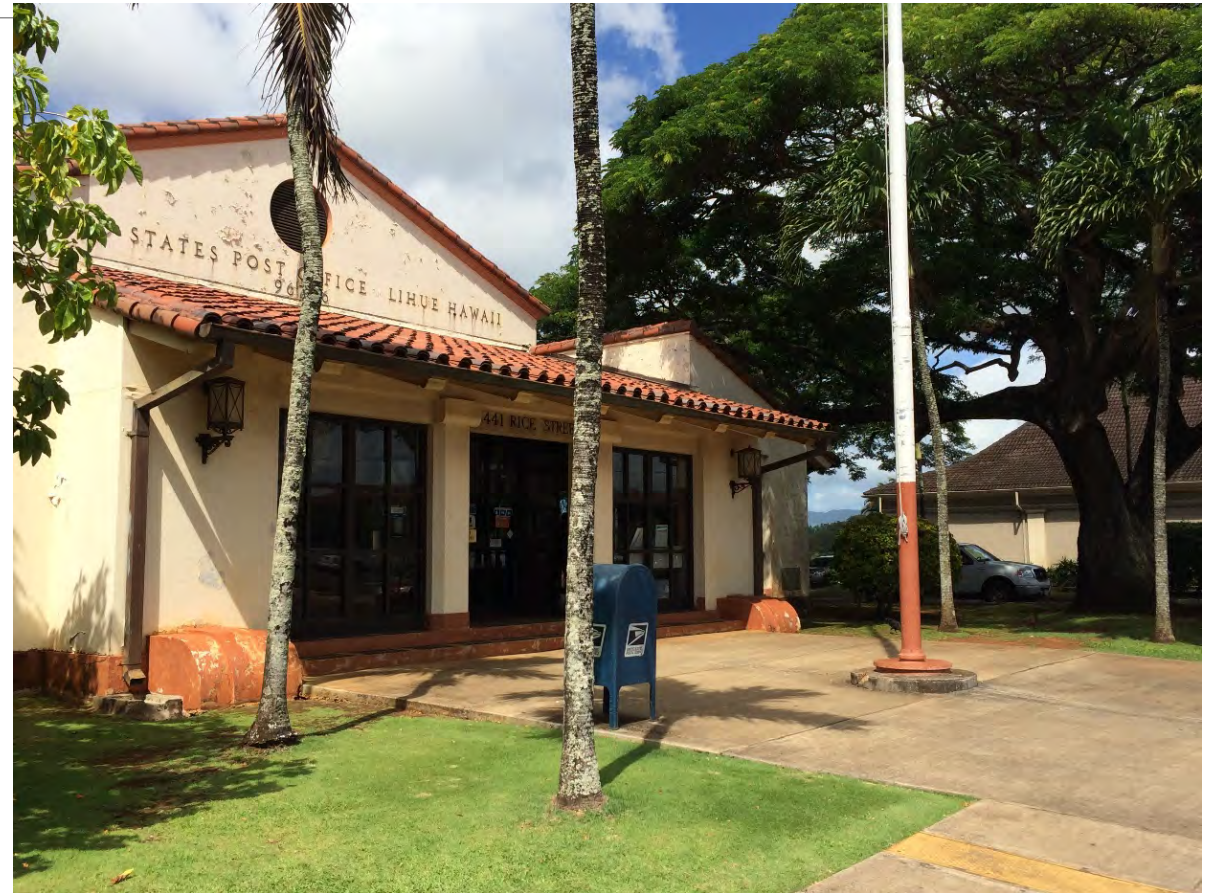
Līhu'e Post Office, Kaua'i, USPS reversed its decision to transfer the historic post office after Sec 106 and other public input opposed the proposal. Photo courtesy HHF.
