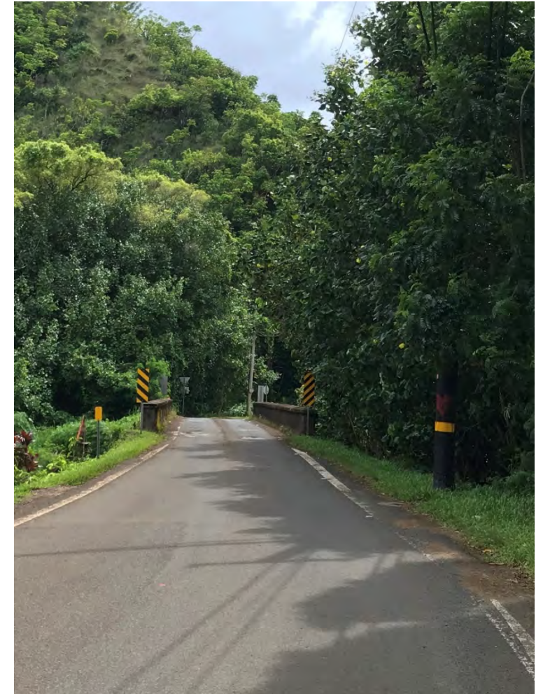
Kaua'i Belt Road Historic District
