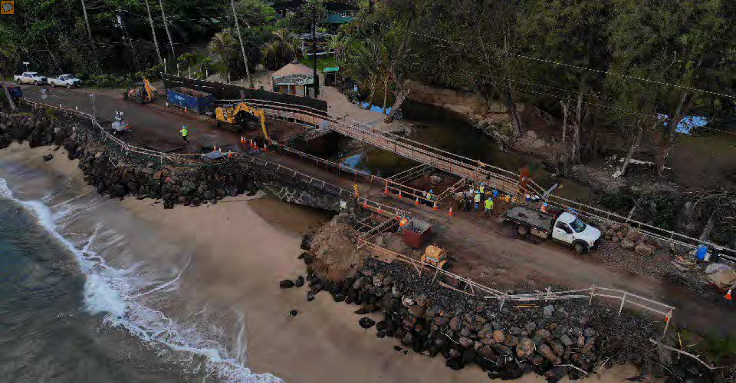
Waikoko Bridge Repairs, April 27, 2019. Photo courtesy HDOT
