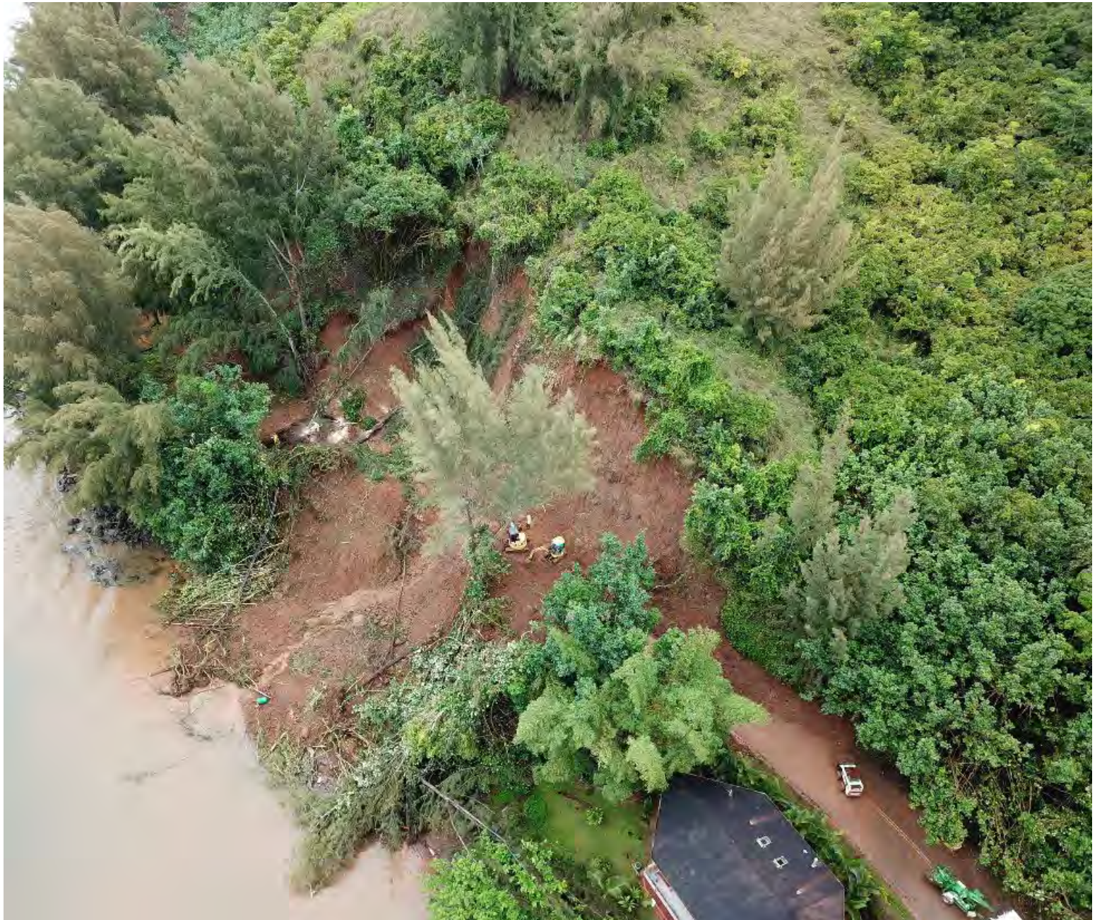
Repair Site #2. Courtesy HDOT.
