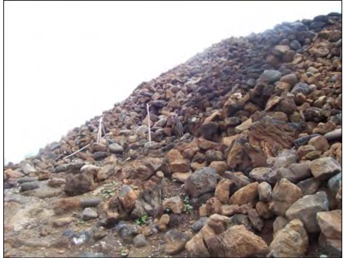
Earthquake Damage at Pu'ukohalā Heiau, Hawai'i. Photo courtesy NPS.
