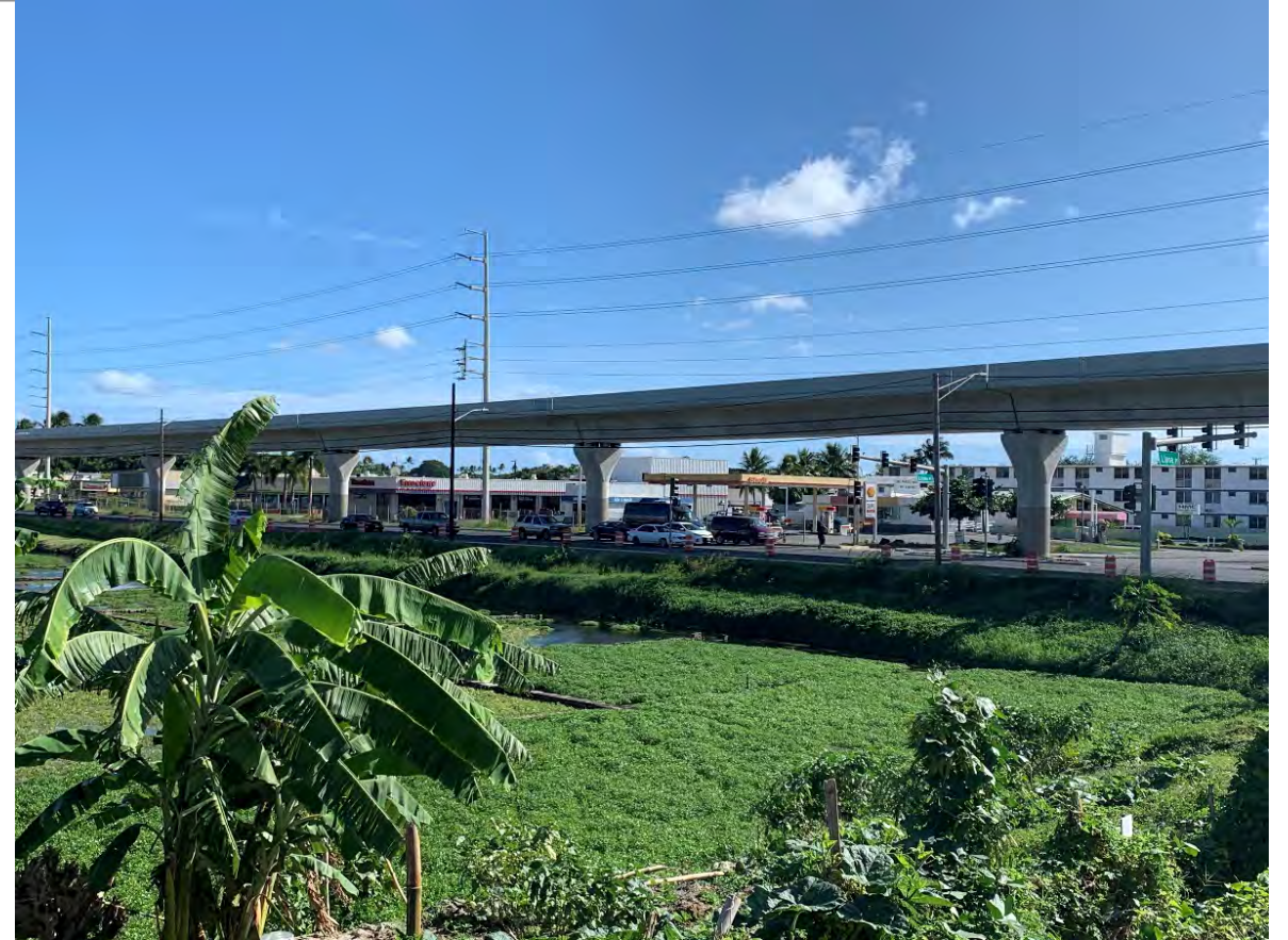
A segment of Honolulu's elevated transit project is adjacent to several sites, including the Sumida Watercross Farm. Photo courtesy HHF.
