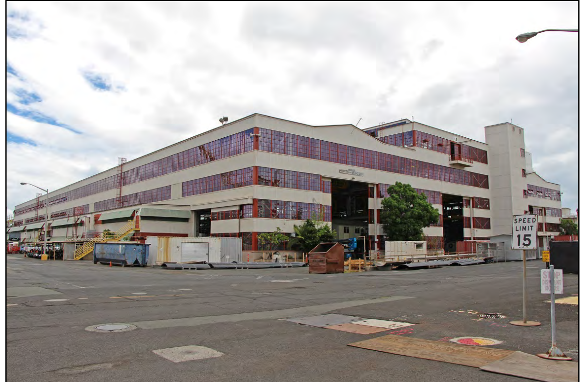
Building 155 in the Pearl Harbor National Historic Landmark avoided adverse effect through the redesign of the project so it complied with SOI Standards. Photo courtesy of US NAVY, PHNSY & IMF
