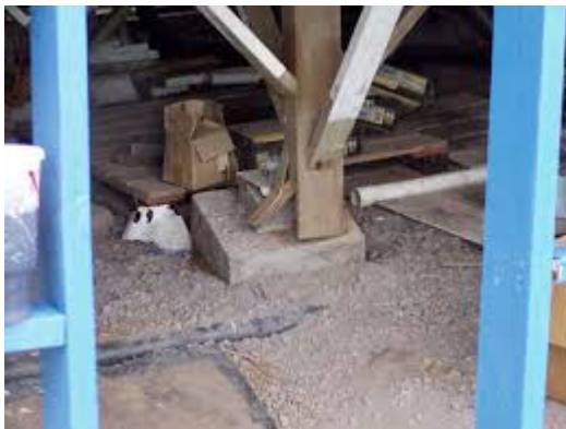
Figure 1 — Post Base with 1" Standoff
