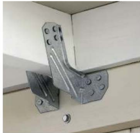
Two HPTZ ties installed with nails.
