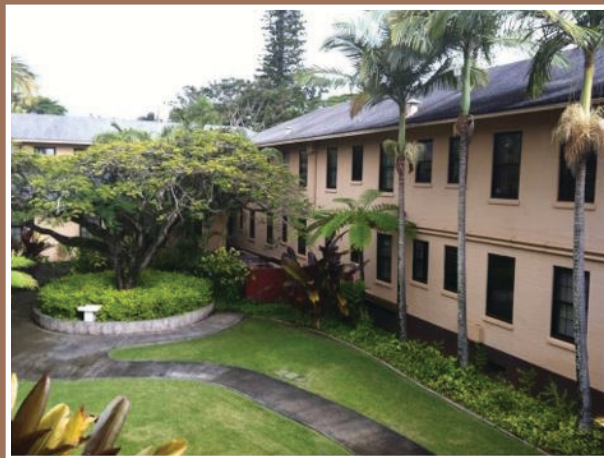
Schofield Barracks Medical Clinic O'ahu
