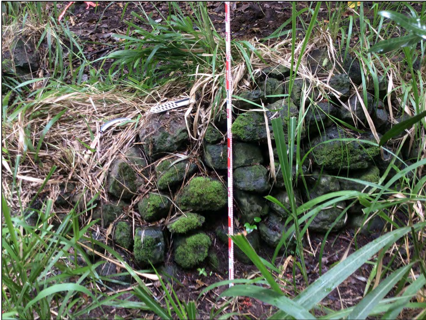
Figure 55. Northwest wall of SIHP # 50-80-03-7977 Feature A terrace showing the stacked basalt construction approximately five to six courses tall, view to east
