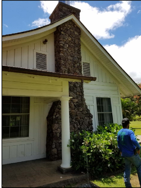
Figure 25. General overview of western side of great room; basalt fireplace visible in center of photograph, view to southeast
