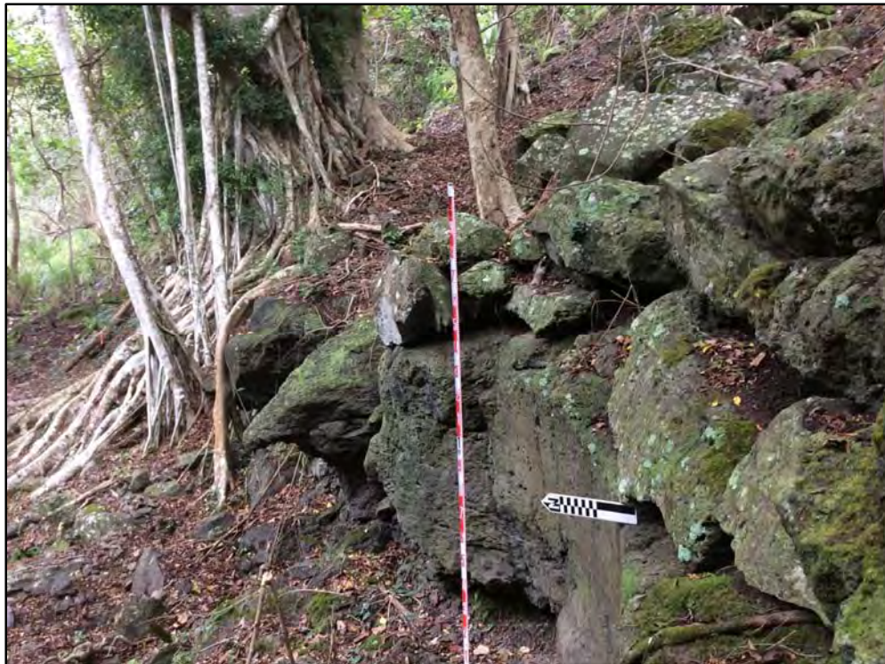
Figure 59. Northern portion of terrace wall of SIHP # 50-80-03-7977 Feature D, showing growth of banyan tree on wall face, view to east
