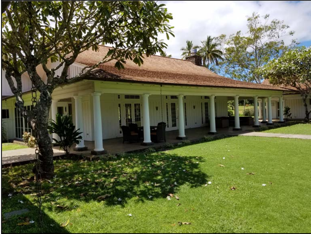
Figure 21. General overview of north-facing portico of the “Big House,” view to southwest
