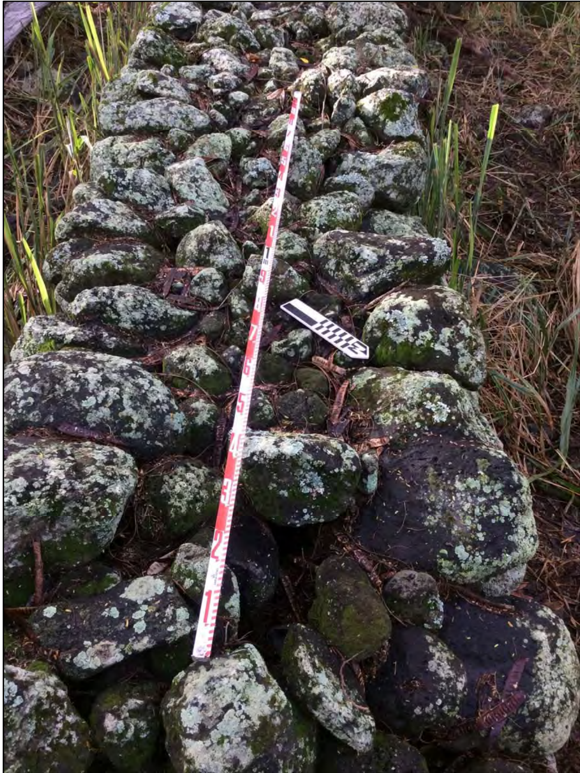
Figure 30. Oblique view showing top of SIHP # 50-80-03-4777 Feature C (intact portion), view to southwest
