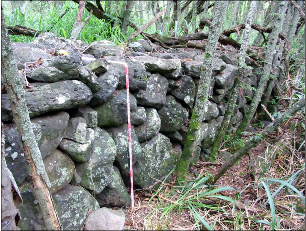
Figure 27. Photograph of SIHP # 50-80-03-4777 Feature A wall, view to north (Tulchin and Hammatt 2008a)
