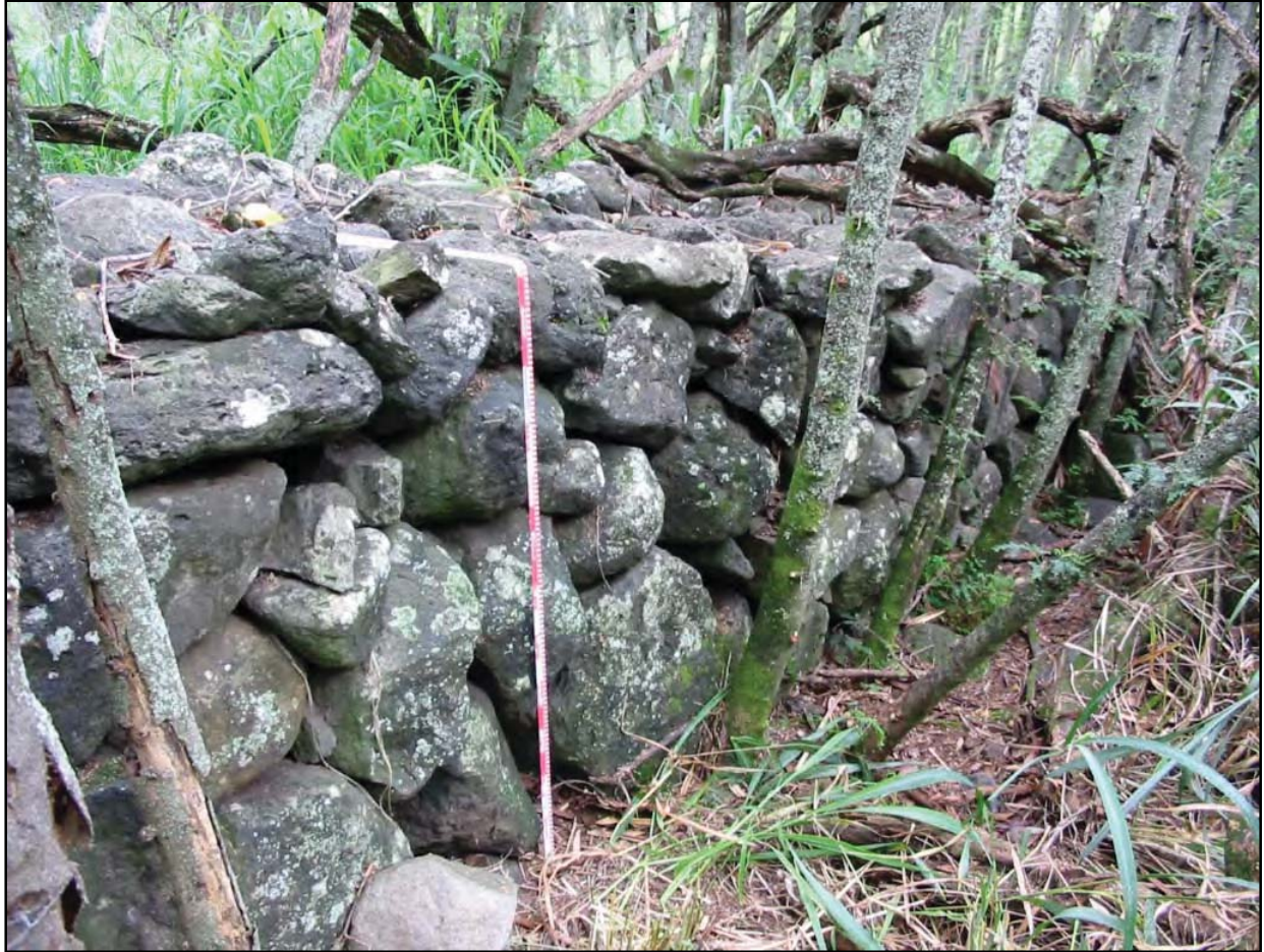
Figure 40. Photograph of SIHP # 50-80-03-4777 Feature A wall, view to north (Tulchin and Hammatt 2008a)
