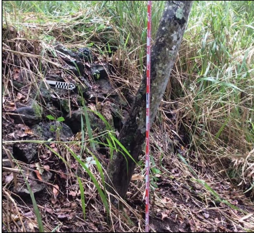
Figure 85. SIHP # 50-80-03-7977 Feature E terrace wall that runs in an east-west orientation across the river valley, view to west (Belluomini et al. 2017–draft)
