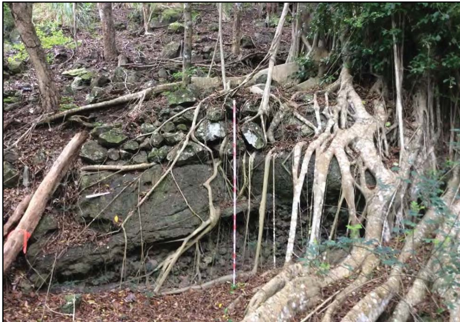
Figure 82. Southern portion of terrace facing of SIHP # 50-80-03-7977 Feature D, showing the banyan tree overtaking most of the structure, view to east (Belluomini et al. 2017–draft)
