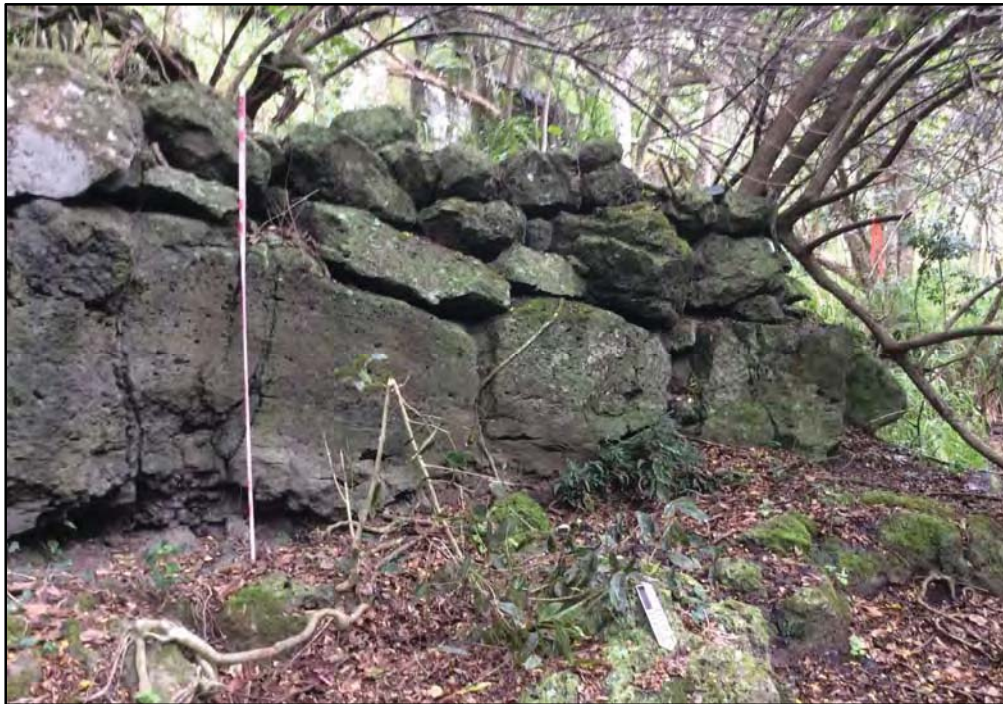
Figure 84. Southern portion of SIHP # 50-80-03-7977 Feature D wall showing stacked stone atop boulder construction, view to south (Belluomini et al. 2017–draft)
