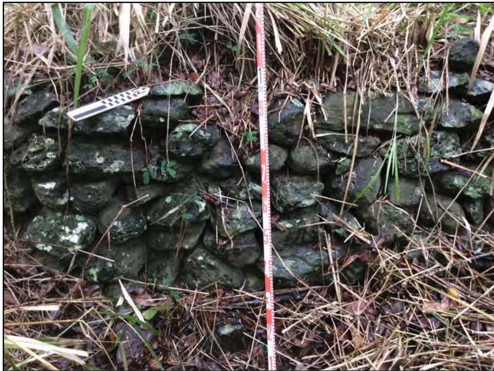
Figure 87. Stacked basalt wall of SIHP # 50-80-03-7977 Feature F located on west bank of stream, view to west (Belluomini et al. 2017–draft)
