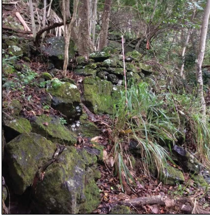
Figure 81. Northern portion of SIHP # 50-80-03-7977 Feature C showing the terrace wall and SIHP # 50-80-03-7977 Feature D in the background, view to south (Belluomini et al. 2017–draft)
