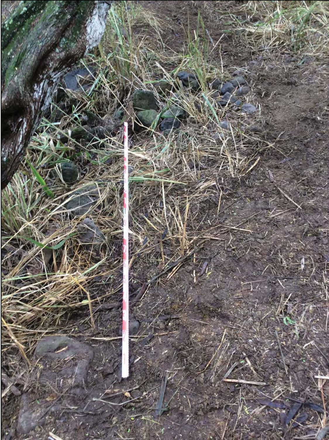
Figure 46. SIHP # 50-80-03-4777 Feature C (remnant portion) at the wash, showing the portion of the wall completely destroyed by water runoff, view to north (Belluomini et al. 2017–draft)
