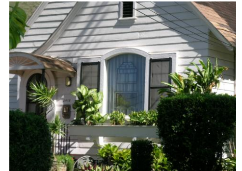
Sash windows may be divided into three parts of varying heights
