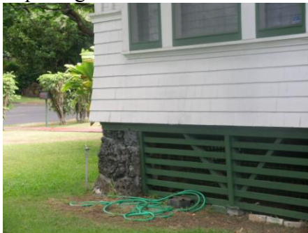
Wood-slat foundation vent
