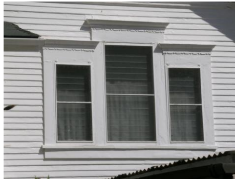
Sash windows may be divided into three parts of varying heights
