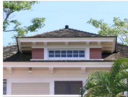
A hipped dormer has a roof with flat surfaces that slope upward at the front of the dormer as well as on both sides.
