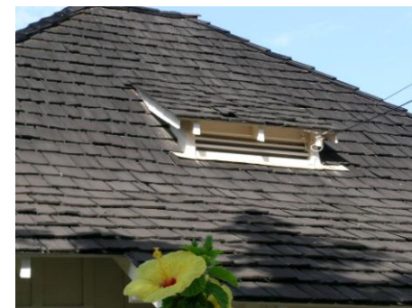
Wood slat attic vent
