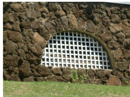
Lattice foundation vent
