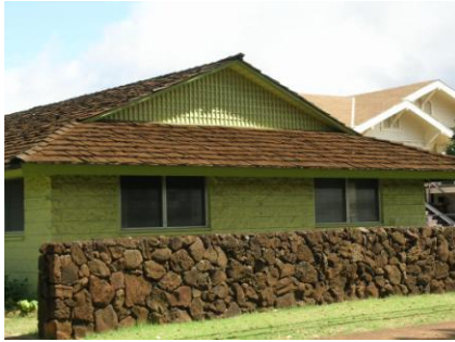
A gable-on-hip roof has a gable that sits on a hipped roof. If the gable is small, it may be called a gablet.
