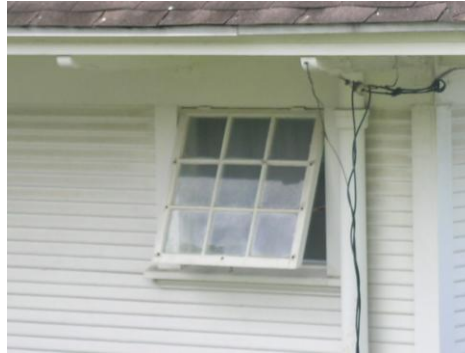
If a sash window pivots about a horizontal axis, they are awning windows.
