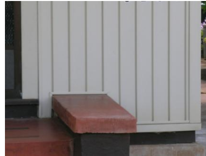
Vertical channel siding has a simple channel
