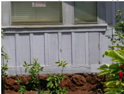
Board-and-batten is lapped siding.
