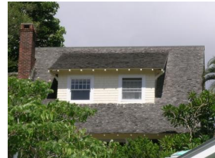
These dormers are shed dormers or shed-roof dormers, whose eave line is parallel to the eave line of the main roof.
