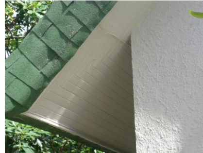
Closed or boxed eaves are enclosed by boards and/or molding so that the rafters are not visible.
