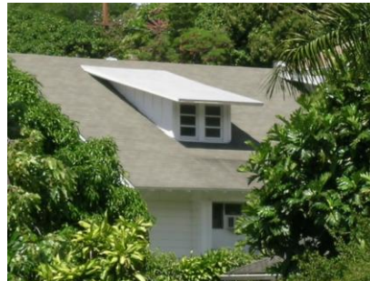
These dormers are shed dormers or shed-roof dormers, whose eave line is parallel to the eave line of the main roof.
