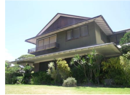
A gable-on-hip roof has a gable that sits on a hipped roof. If the gable is small, it may be called a gablet.
