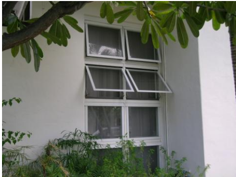
If a sash window pivots about a horizontal axis, they are awning windows.
