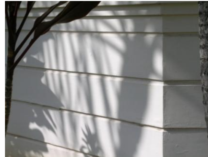
Drop siding has a simple channel
