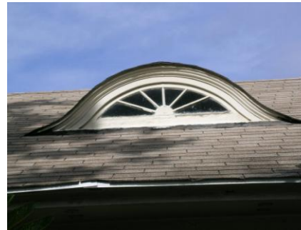
An eyebrow dormer has no sides and roof is carried over in a wavy line. An inset dormer is partially set below the sloping roof.
