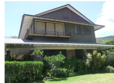
Closed or boxed eaves are enclosed by boards and/or molding so that the rafters are not visible.
