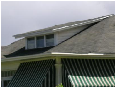
These dormers are shed dormers or shed-roof dormers, whose eave line is parallel to the eave line of the main roof.
