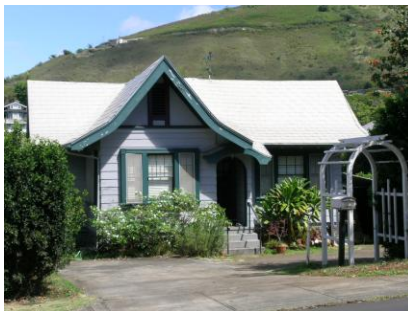
Bellcast eaves or flared eaves are the part of the roof that has a gradually diminishing slope and projects beyond the face of an exterior wall, flaring upward near its lower end. Flemish in origin.
