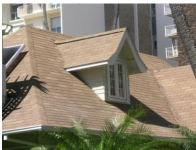
Above are gable dormers, also known as gabled dormer or triangular dormer, which have a triangular gable roof.
