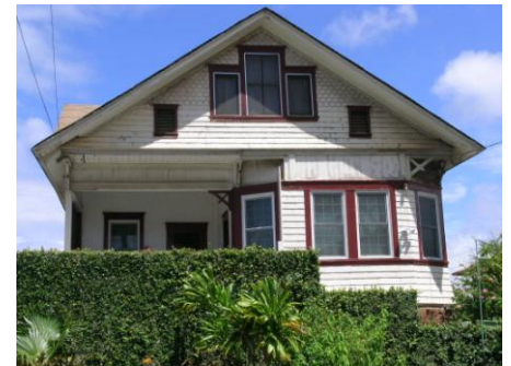
These houses have an inset, or integral, porch which is set within the main structure of the house
