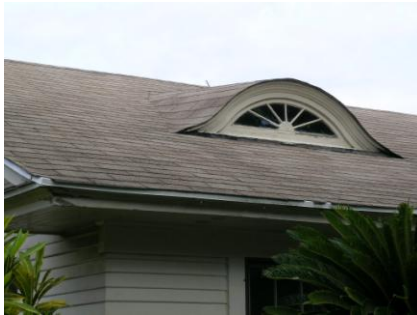
An eyebrow dormer has no sides and roof is carried over in a wavy line. An inset dormer is partially set below the sloping roof.
