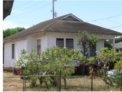
A gable-on-hip roof has a gable that sits on a hipped roof. If the gable is small, it may be called a gablet.
