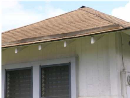
Open eaves are overhanging eaves in which the roof rafters are visible from below.
