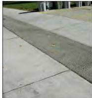
Stormwater percolates through pavement to either infiltrate or be collected and directed to storm drain line. Added depth of subbase can
