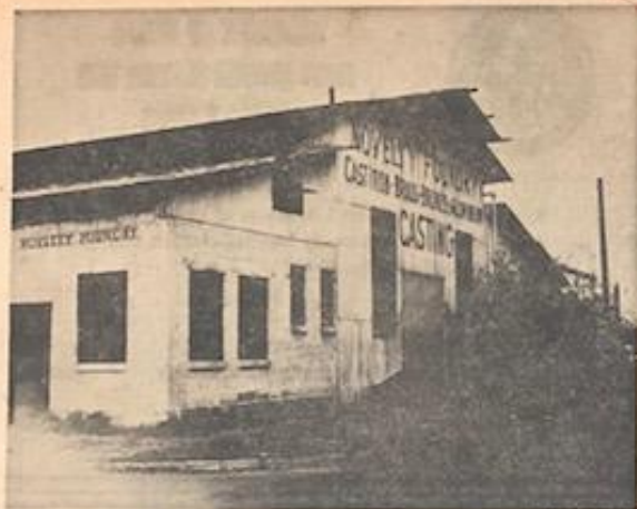
Exterior of junk-strewn metal foundry before work began.
