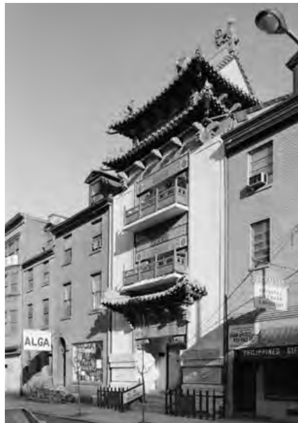
Built in 1832 and altered considerably over time, the YMCA building is an icon in Philadelphia’s Chinatown; it once housed the Chinese Cultural and Community Center, but has been closed since 2007. Photo courtesy of the Library of Congress.
