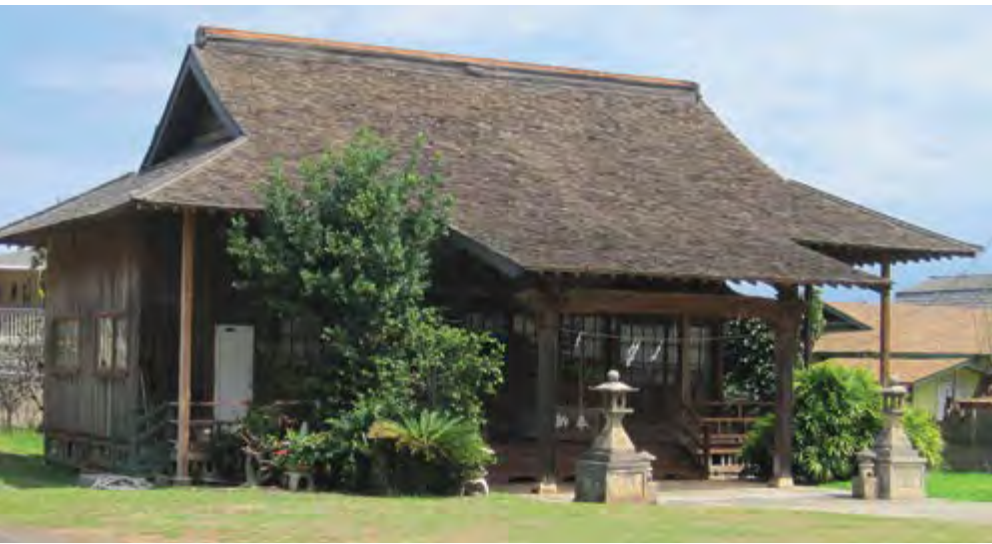
The Jinsha Mission shrine is the only major Shinto shrine in Maui and one of the best preserved examples of the traditional shrine-building techniques employed by Japanese carpenters. Photo by Joel Bradshaw; courtesy of Wikimedia Commons, licensed under Creative Commons.
