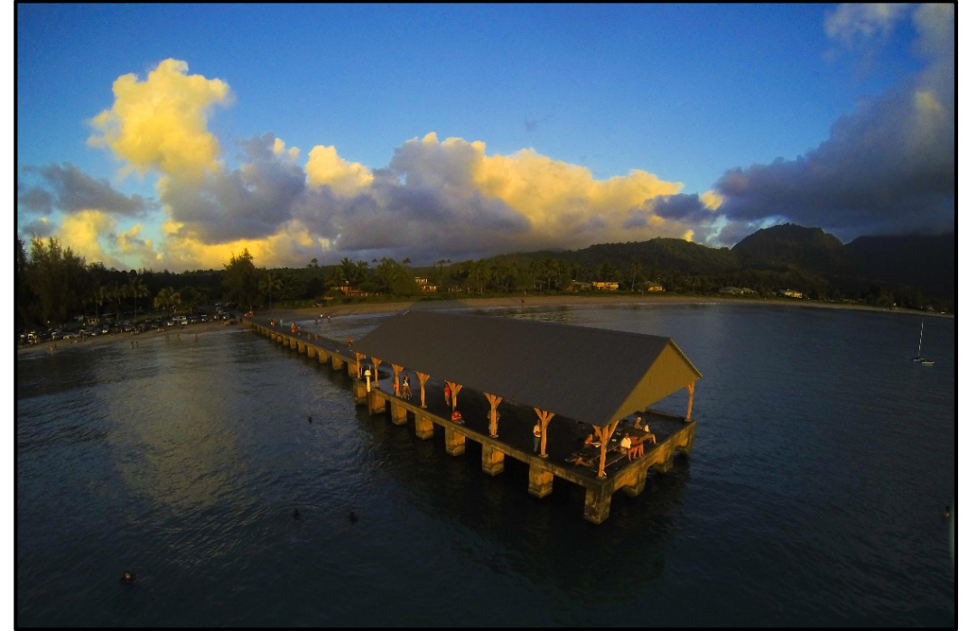
Hanalei Pier (Photo by Joel Guy)
