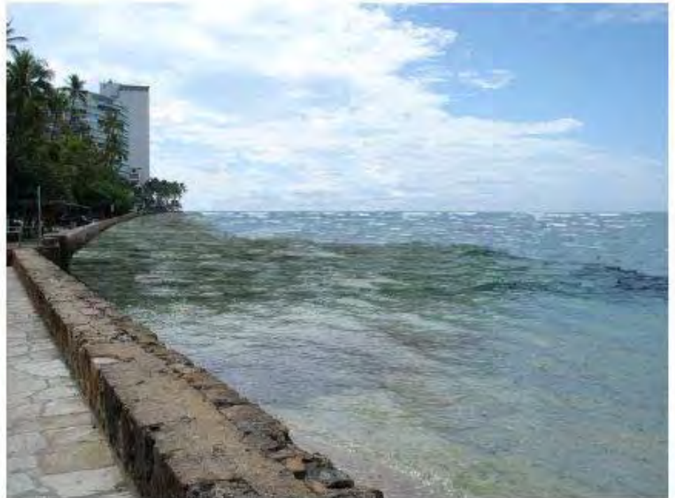
View After the Removal
