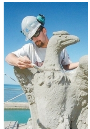
Replacing an eagle's head on the facade in 2000.
