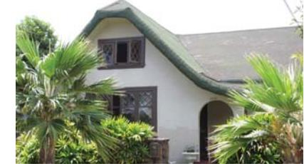
**12** The **Helene Morgan Residence** is a single story, Hawaiian style duplex with a pair of double-pitched hipped roofs with overhanging eaves and exposed rafter tails. Presently, the house is a single family dwelling, but originally it was two separate laid out units connected by a passage. The duplex sits on a raised, post and pier, foundation with lava rocks at the base.
