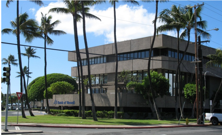
WARD PLAZA, 1969 AU, CUTTING, SMITH AND ASSOCIATES
