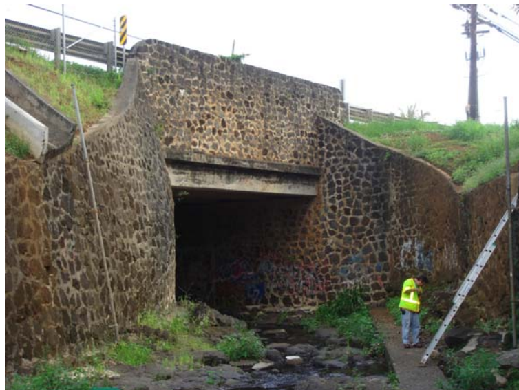
Kawa Stream Bridge (1939) Oahu State: 003063001400065
