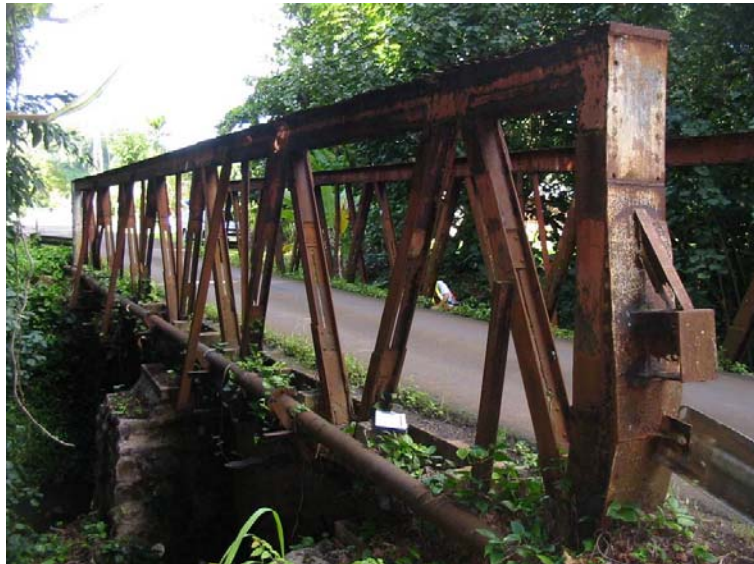
Opaekaa Bridge (1900) County of Kauai: 007420151142001
