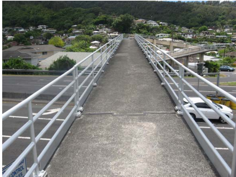
Kula Kolea Pedestrian Overpass (1960) Oahu State: 003000630000234
