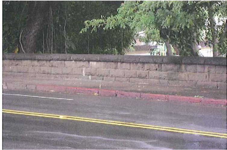
Nuuanu Stream Bridge County of Honolulu: 003083471400113
