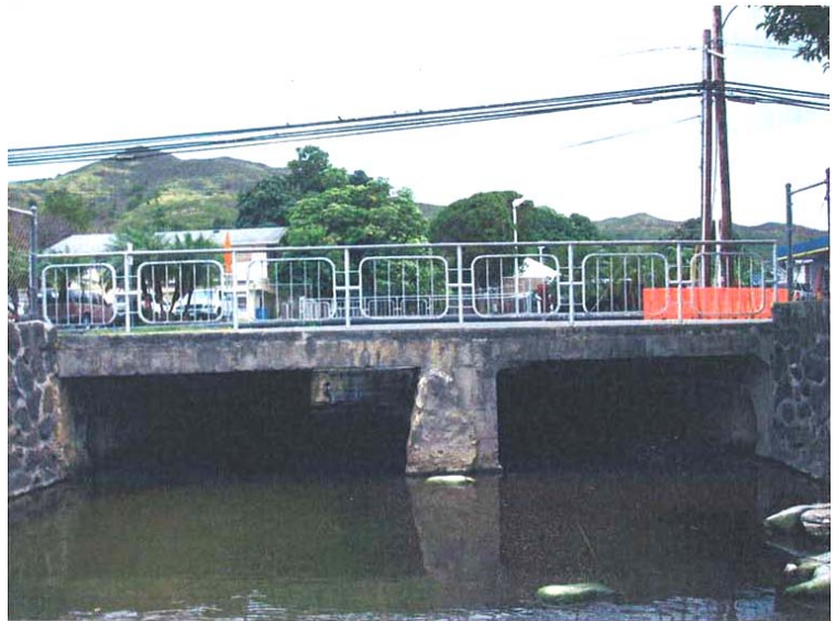
Keolu Drive Bridge-Hele Drainage Channel (1957) County of Honolulu: 003427001100001
