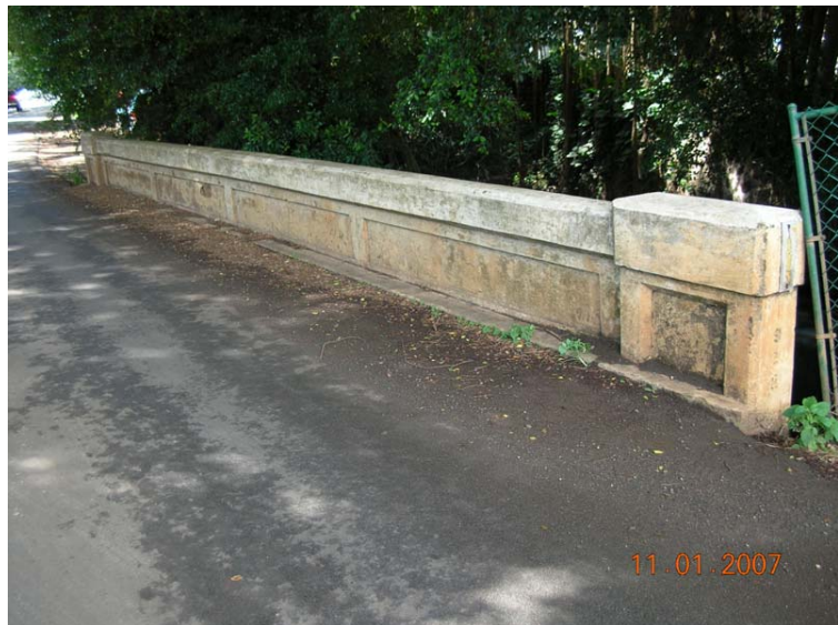
Waikomo Stream (Koloa Road Bridge) (1928) County of Kauai: 007270100828001
