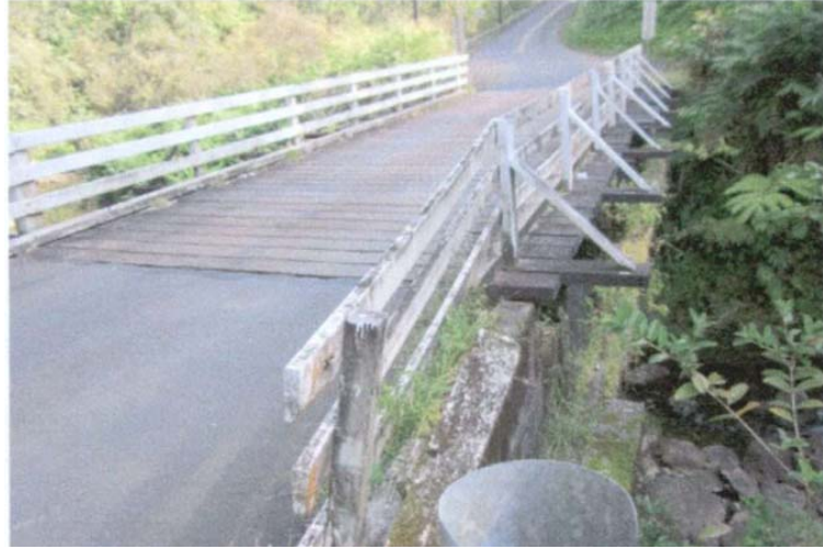
Maili Stream Bridge (1900, replaced in kind in 1974) County of Hawaii: 001260001100003
