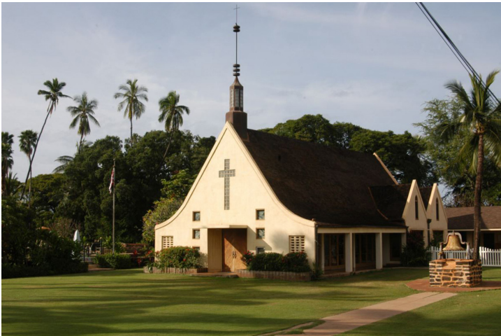
Figure 23 : Waiola Congregational Church, (1953) Source: https://sah-archipedia.org/buildings/HI-01-MA23
