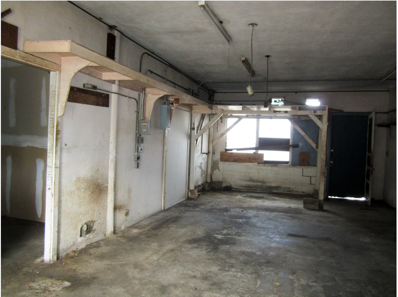
Figure 6: First floor former Chikara Mochi commercial space. View facing southeast.
