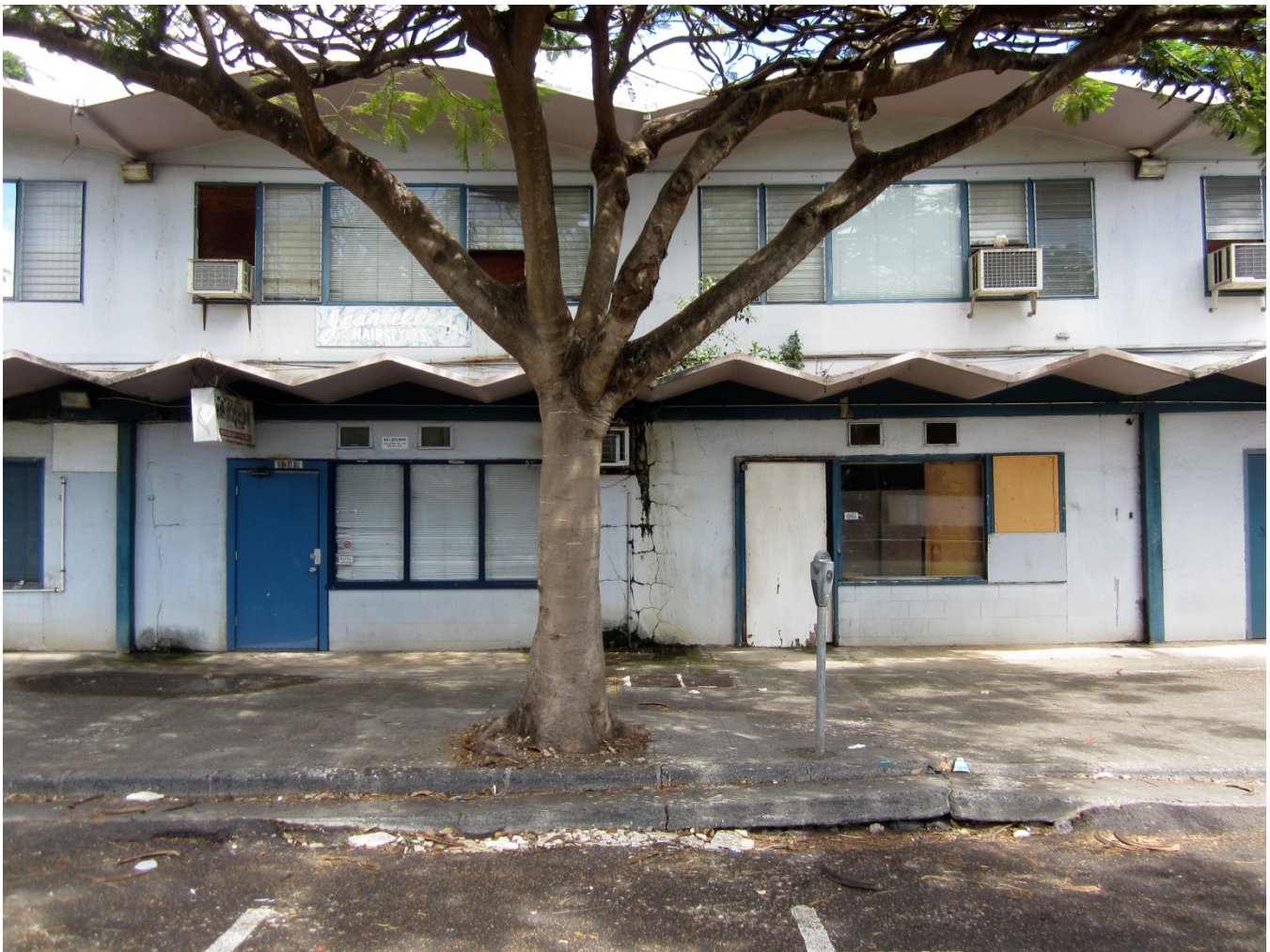
Figure 1: View of River Street façade, showing typical store front spaces with folded plate concrete awning at first floor and second floor offices with thin shell concrete barrel arched roof. View facing southeast.
