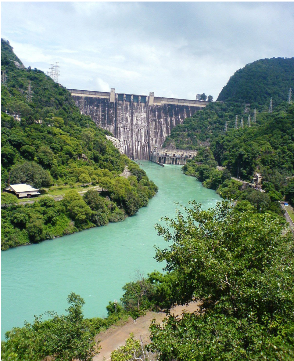
Figure 3.1. Bhakra Dam, 1963, Bilaspur, Himachal Pradesh, India. At 226 meters (741 feet) in height, this concrete gravity dam is the tallest in India and among the tallest in the world. It dams the Satluj River to create India's third-largest reservoir, holding excess waters during the monsoon and providing regulated release throughout the year. The dam feeds the Bhakra Canal, which provides irrigation to ten million acres of fields in Punjab, Haryana, and Rajasthan. Electric power produced by the dam's generators is distributed to Himachal Pradesh and five neighboring states.
