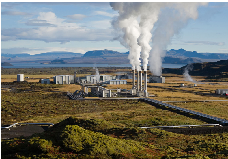
Figure 2.4. Nesjavellir Geothermal Power Plant, 1990, Thingvellir, Iceland. This facility, the second-largest geothermal power station in Iceland, serves the space-heating and hot-water needs of Reykjavik by tapping into the earth’s heat and using underground water to operate a turbine, which generates electricity. In the early twentieth century, the rising demand for electricity led to the search for new sources of electric power. Geothermal electricity was first produced commercially in Italy in 1913. While other countries experimented with it, it was not until 1958 that the second major geothermal plant opened, in New Zealand. Additional plants followed, continuing the ever-expanding search for electrical power sources.
