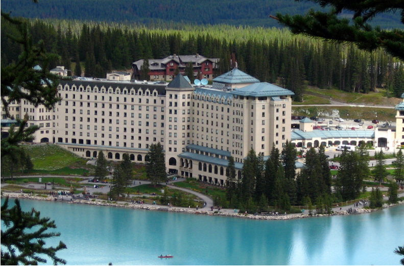
Figure 8.13. Chateau Lake Louise, 1890s–1980s, Banff National Park, Alberta, Canada. One of a series of tourist hotels constructed by the Canadian Pacific Railway along its transcontinental line, Chateau Lake Louise provided lodgings for travelers but, with its spectacular natural setting, was also a destination in itself. Such grand railway hotels spurred the development of national park tourism in Canada, the US, and other countries. The Chateau was expanded and modernized a number of times over the years (the oldest portion of the current hotel dates to 1912) to accommodate growing numbers of visitors, especially after the advent of automobile travel.
