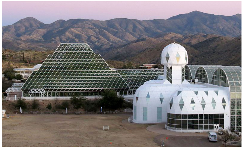
▶ Figure 2.14. Biosphere II, 1987–91, Oracle, Arizona, USA. This innovative scientific research facility was designed to emulate the earth's environment to assess whether humans could build self-sustaining colonies in outer space. Essentially a giant terrarium, the privately funded, 3.14-acre (1.27-hectare), airtight steel-and-glass structure holds five biomes, including living quarters and agricultural areas. It is the largest closed system ever constructed. In 1991, a team of four men and four women were sealed inside for a two-year period to study survivability; a second, much shorter mission was conducted in 1994. It is currently operated by the University of Arizona.
