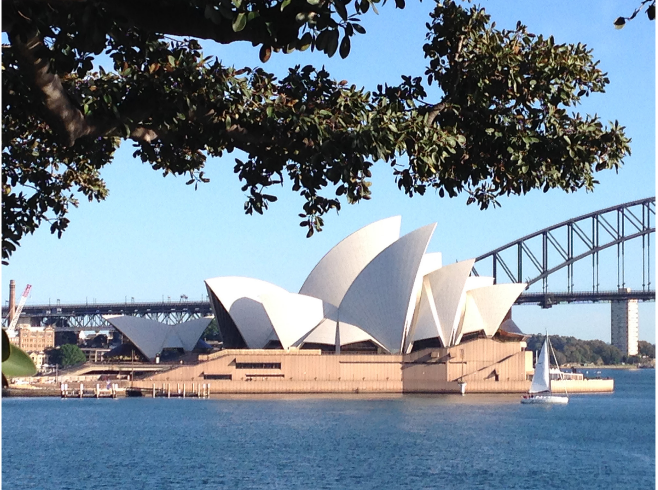
▲ Figure 2.5. Sydney Opera House, 1958–73, Sydney, Australia. Designed by Danish architect Jørn Utzon with British-born Ove Arup as structural engineer, the structure features three groups of interconnecting, vaulted concrete shell structures set on a monumental podium on a harbor peninsula. To understand the complex forces to which the curving, precast panels and arches would be subjected, the designers were among the earliest to use computers in structural analysis. The site was inscribed on the World Heritage List in 2007 as a “masterpiece of human creative genius.”
