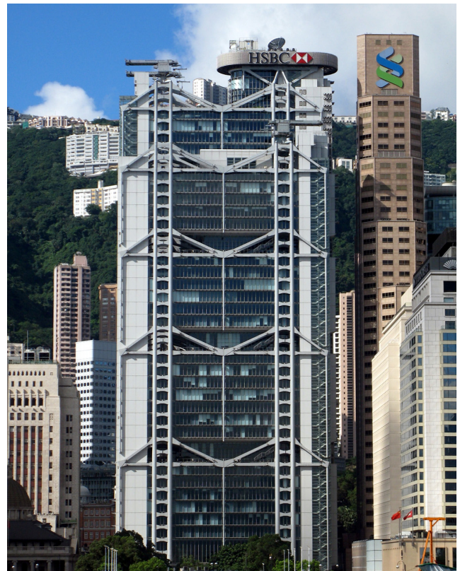
Figure 2.7. Hongkong and Shanghai Banking Corporation (HSBC) headquarters, 1979–86, Hong Kong, China. Located in central Hong Kong, the HSBC was designed by British architect Norman Foster and structural engineering firm Arup Partners, based in London. It is an example of the High-Tech phase of modern architecture, which clearly expresses the building's structural system and materials and a high degree of prefabrication. The pronounced exterior mast structure and placement of exposed service cores on the outside edges of the towers allow for an open interior free of structure. This included a ten-story atrium, on top of which a mirrored sun scoop reflected light down through the atrium to the ground-level plaza.
