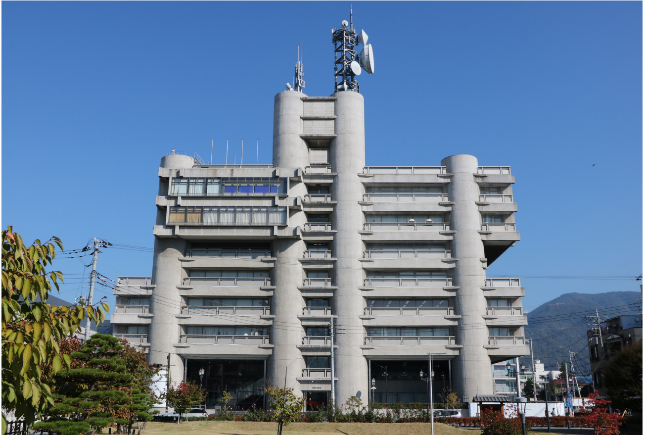
▲ Figure 5.11. Yamanashi Press and Broadcasting Center, 1961–66, Kōfu, Yamanashi Prefecture, Japan. Designed by Japanese Metabolist architect Kenzo Tange, this cast-in-place concrete building was planned to accommodate three major communication functions: a newspaper printing plant, a radio station, and a TV broadcasting station. These functions were legible in the design of the facade, with printing equipment located on the ground floor, sealed studios on upper floors, glass-walled offices with balconies, and cylindrical service shafts for stairwells, elevators, and HVAC. In addition, free open-plan spaces and fluid transitions to the urban space outside were incorporated.
