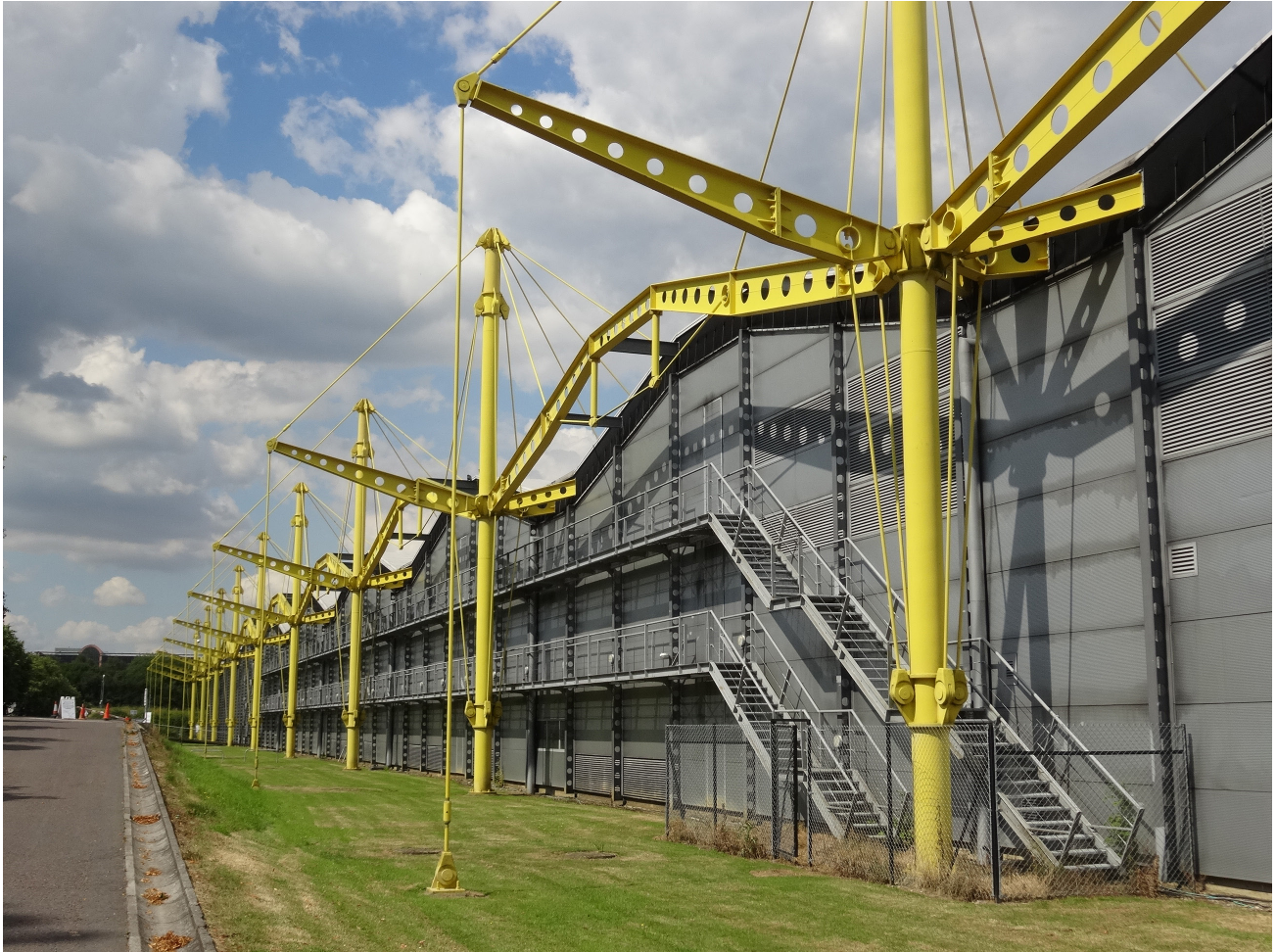
▲ Figure 4.3. Renault Distribution Center, 1982, Swindon, England. During the 1970s, the French car company Renault Group began expanding globally. Designed by Manchester-born architect Norman Foster in the British High-Tech manner, this highly innovative industrial facility incorporated new materials, technology, and design solutions that allowed for interior flexibility and expansion. Renault moved out in 2001, and the structure is now known as the Spectrum Building.
