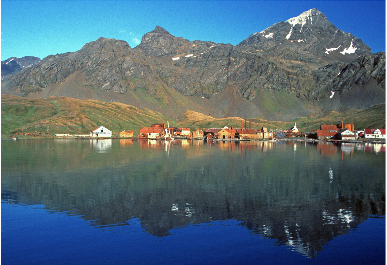
▲ Figure 7.9. Grytviken whaling station, 1904–66, Grytviken, South Georgia Island, British Overseas Territory. Commercial whaling was limited and eventually banned by environmental agreements, reviving some whale species and leaving a heritage of abandoned whaling stations and relics. After sixty-two years of operation, Grytviken whaling station ceased production in 1966 following depletion of the whale population. During that time, an estimated nine million barrels of whale oil were produced at the site. Several species have gradually returned to the area, and the abandoned station has become a tourist attraction.
