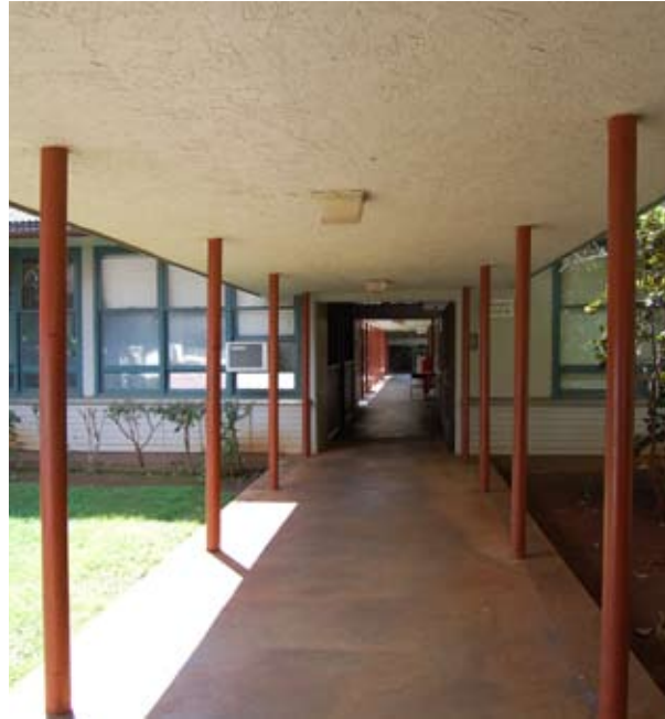
Fig 7.20: Steel Columns at Krauss Hall
