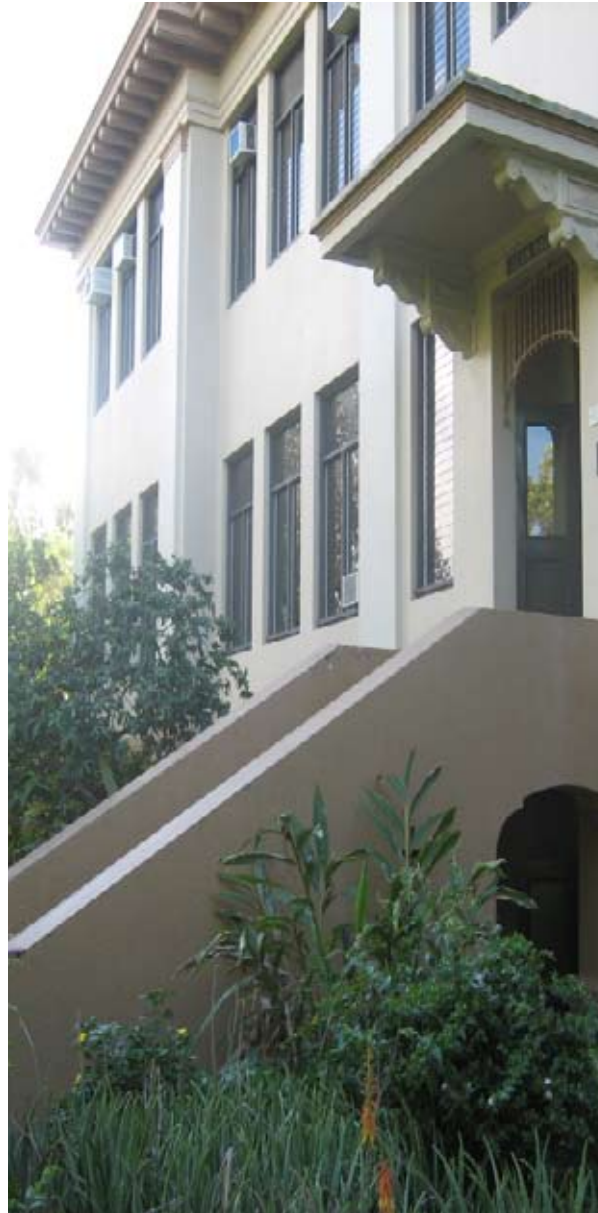
Fig 5.56: Dean Hall main entry, 2007
