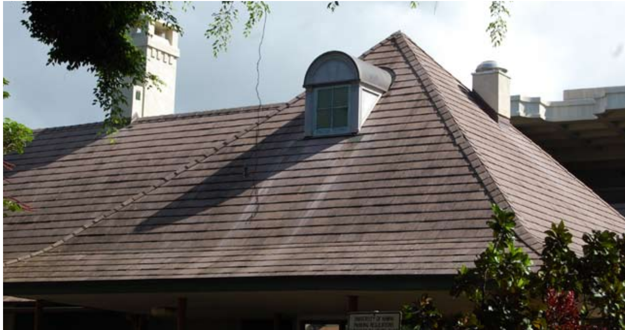
Fig 7.23: Dormer and Chimney on Roof of Krauss Hall, 2008
