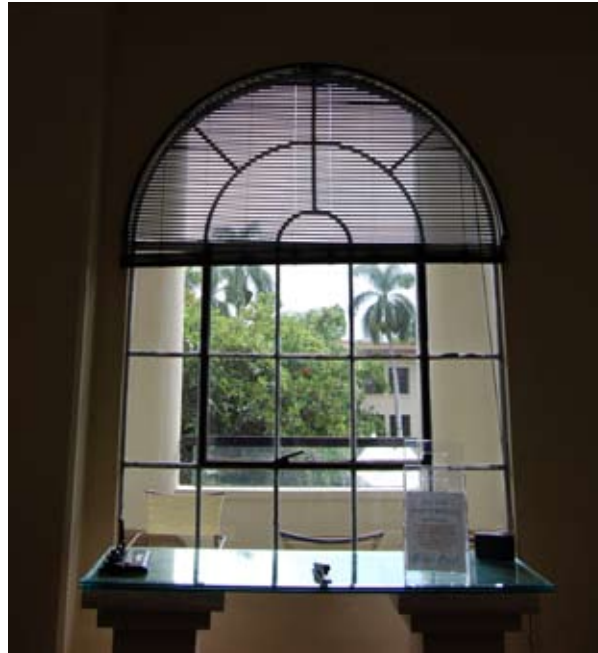
Fig 7.29: Metal Windows at Gartley Hall, 2008
