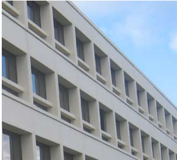
Fig 5.180: Burns Hall western façade, 2007
