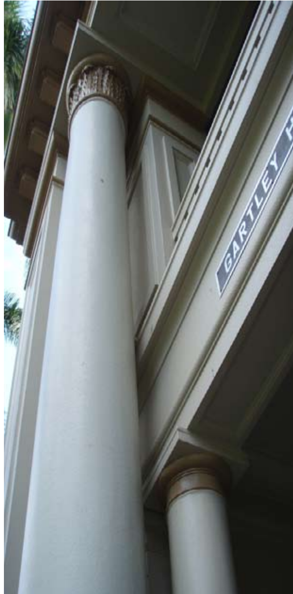
Fig 5.46: Gartley Hall Entry Column Detail, 2007
