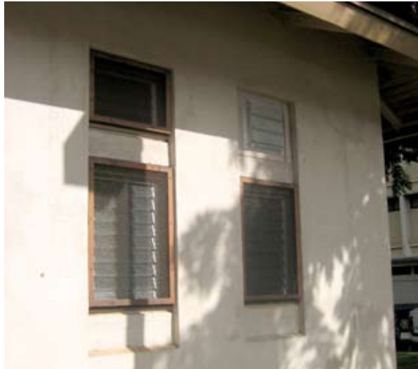
Fig 5.120: Building 37 Window Detail, 2007
