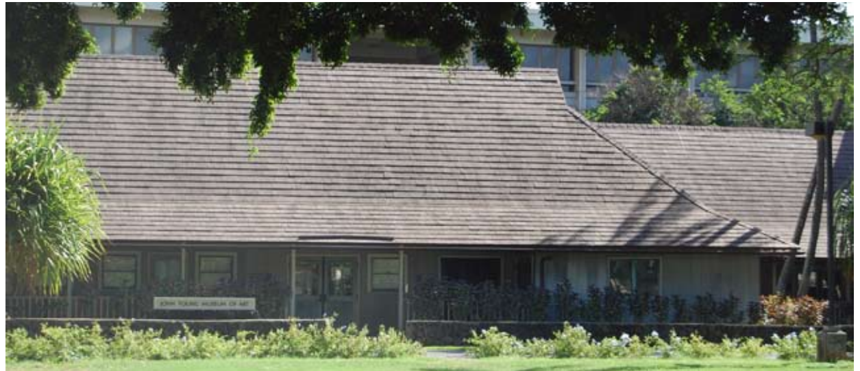
Fig 7.22: Double Pitch Roof with Wooden Shingles at Krauss Hall, 2008
