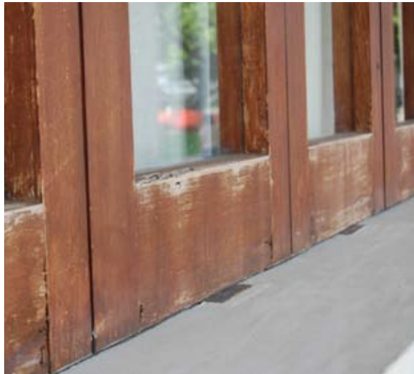
Fig 7.26: Window frames at Jefferson Hall, 2008
