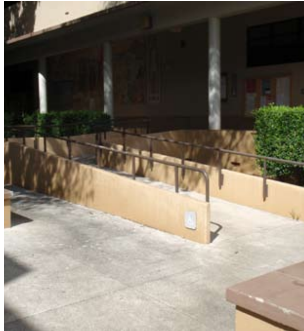
Fig 7.41: ADA Access at Bilger Hall, 2008
