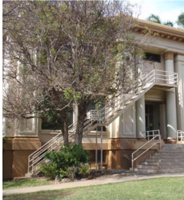
Fig 7.43: Steel Fire-escape at Dean Hall, 2008
