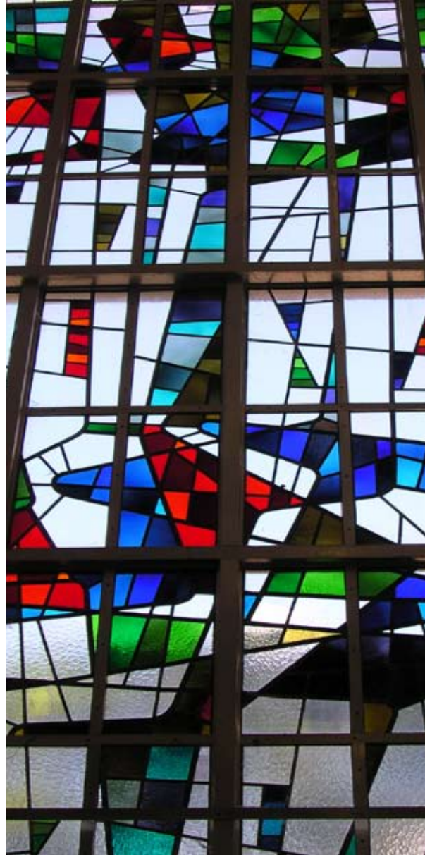
Fig 5.131: Stained Glass Façade, 2007
