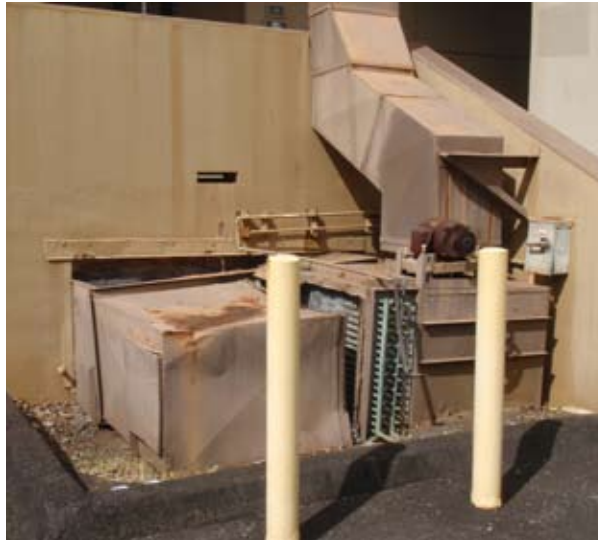
Fig 7.44: Deteriorated AC Duct Work, 2008 Fig 7.45: Deteriorated AC Duct Work, 2008
