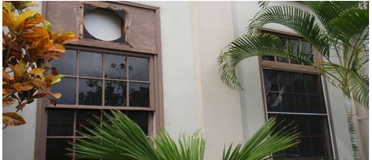
Fig 7.28: Window Modification for Air Conditioning, 2008
