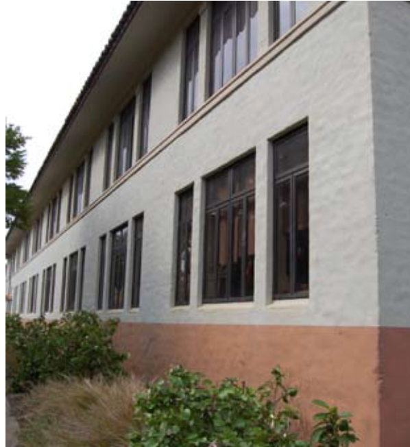
Fig 7.10: Stucco Wall at Wist Hall, 2008
