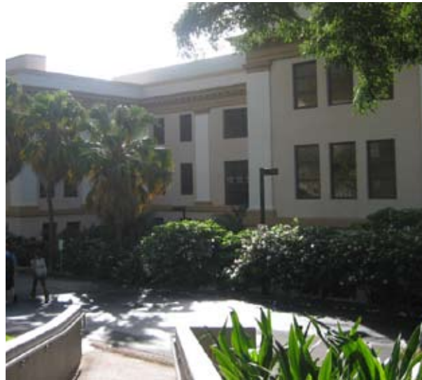
Fig 5.60: Crawford Hall Eastern Facade, 2007
