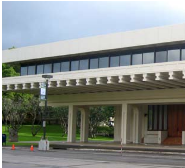
Fig 5.157: Jefferson Hall as seen from East-West Road, 2007
