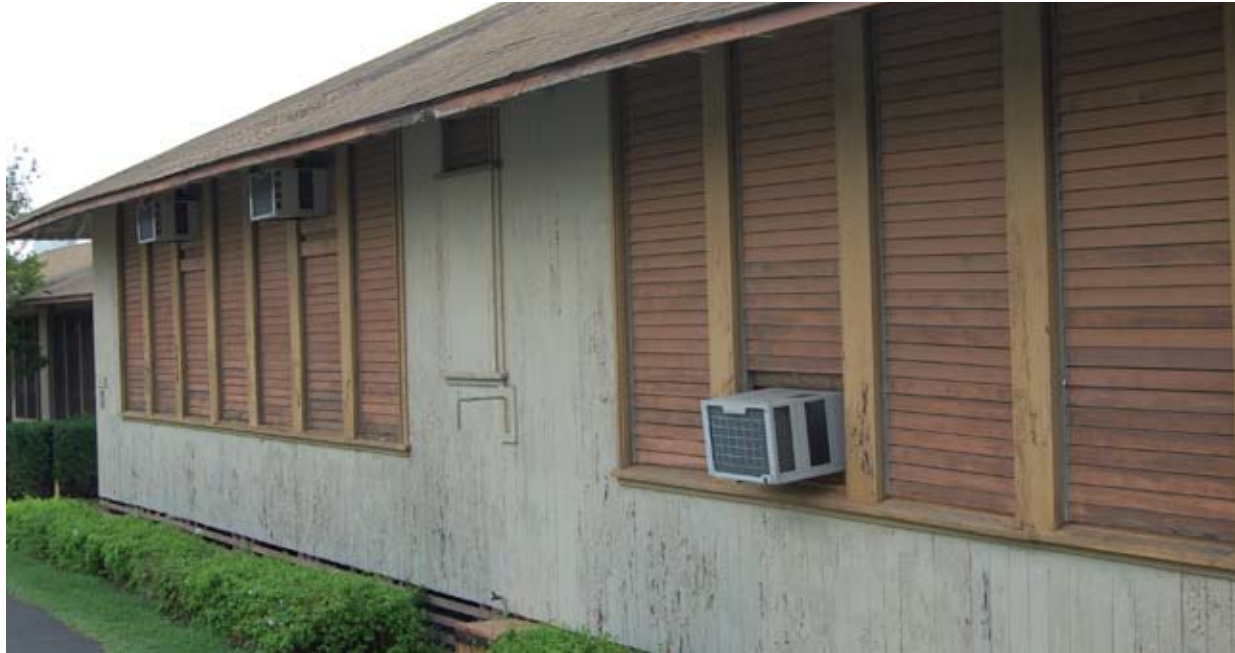
Fig 7.17: Wooden Louver Windows at University High School, 2008
