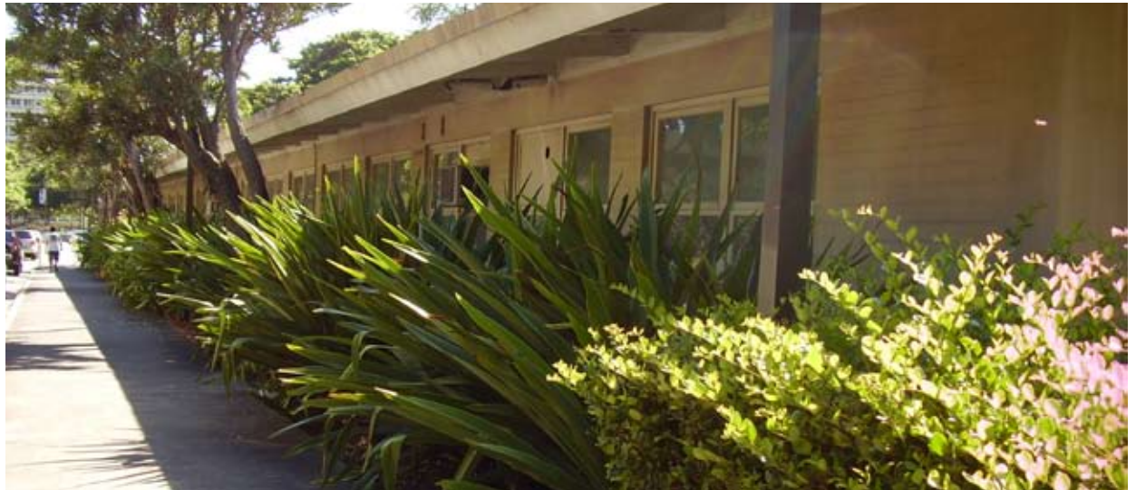
Fig 5.109: View along East-West Road, 2007
