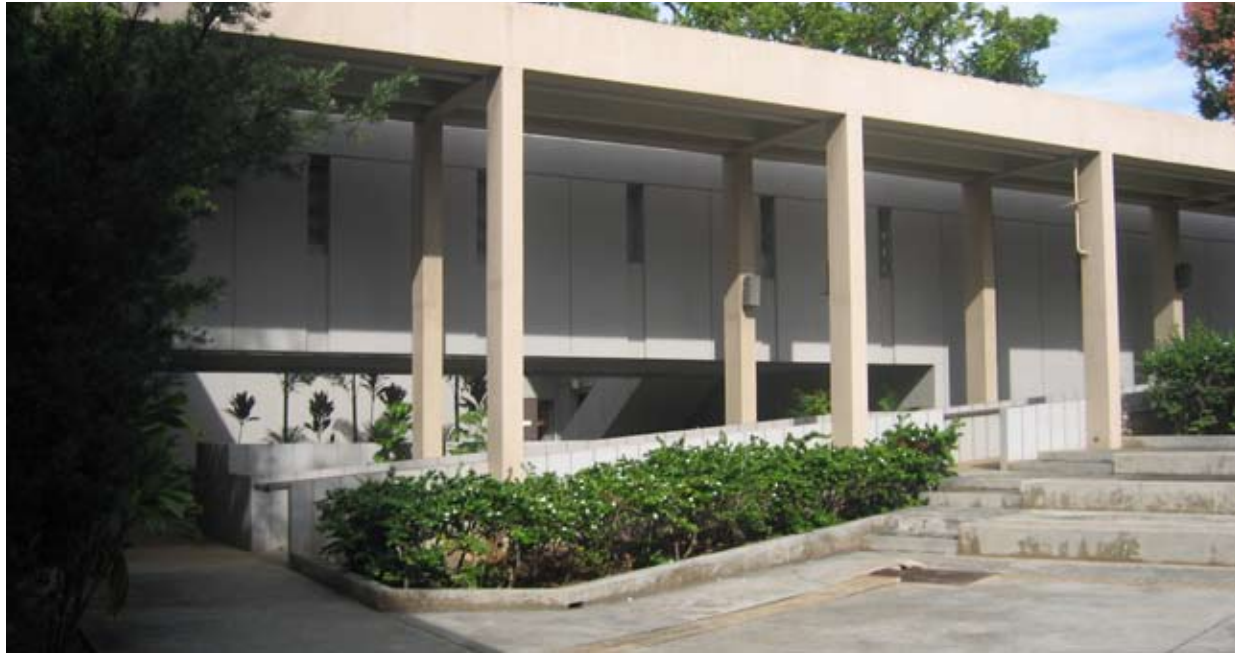
Fig 5.7: Covered Access Ramp, 2008
