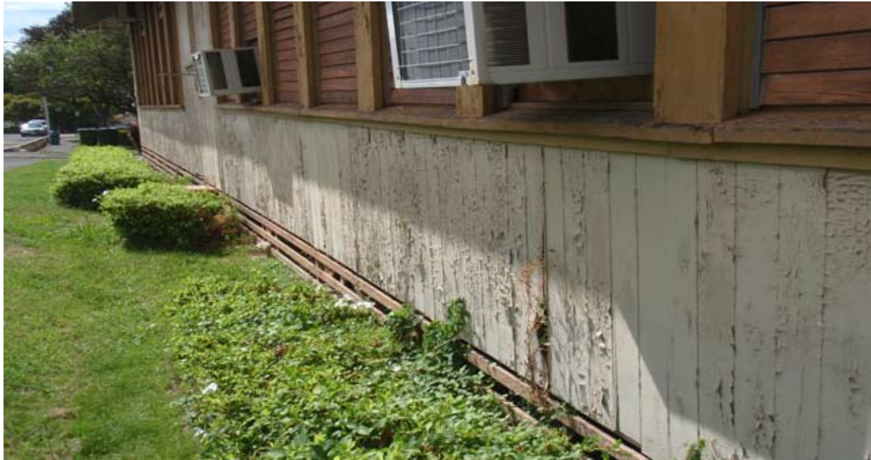
Fig 7.38: Modified Windows to Accommodate Air Conditioning, 2008
