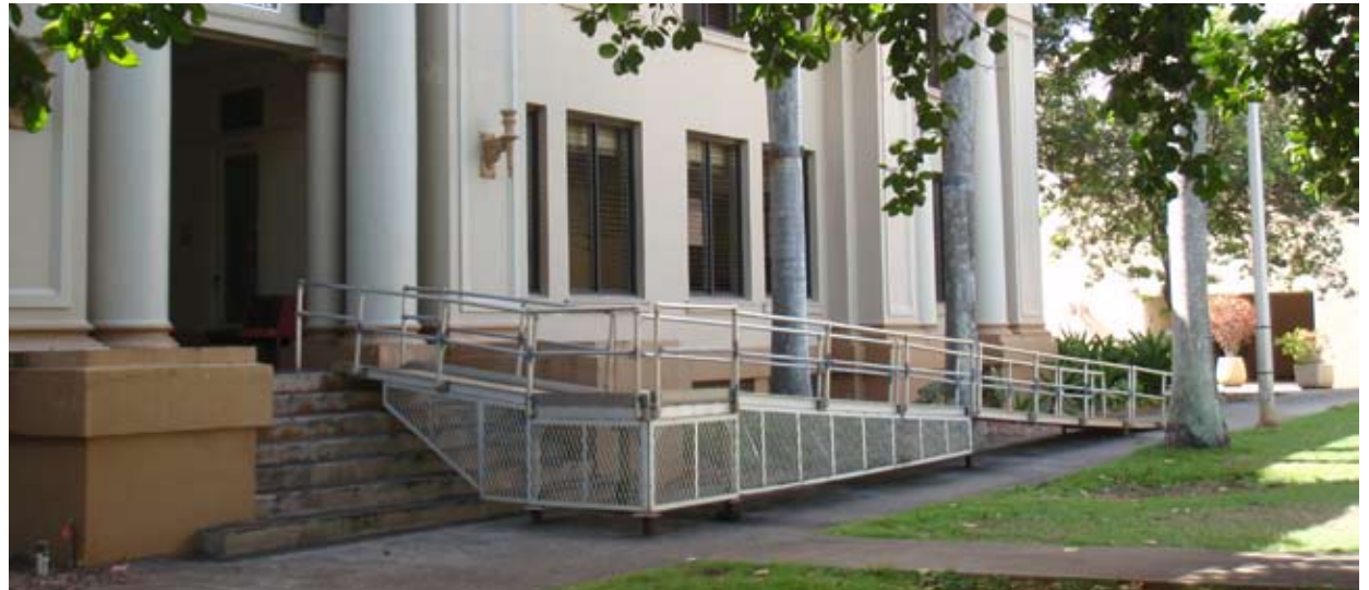
Fig 7.40: Temporary ADA ramp at George Hall, 2008
