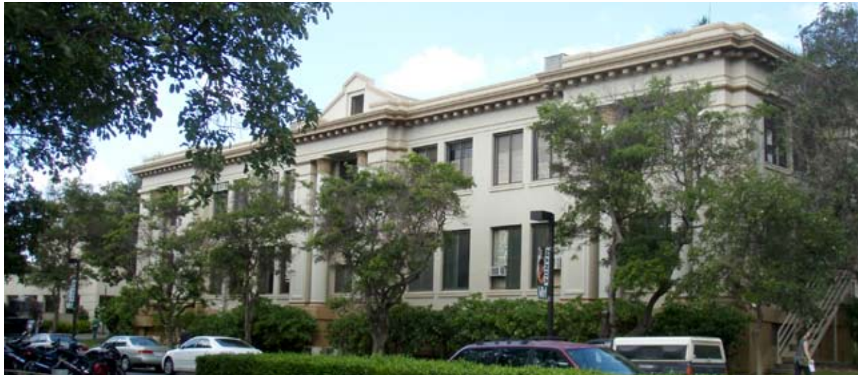
Fig 5.44: Gartley Hall as seen from Campus Road, 2007
