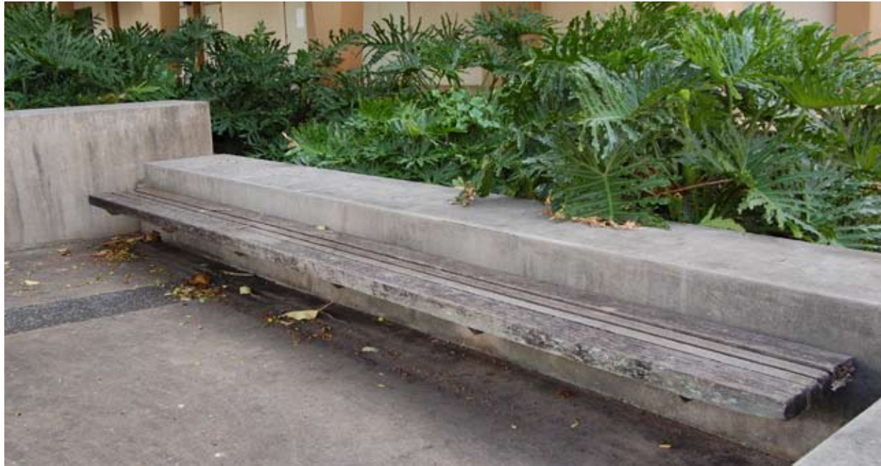
Fig 7.14: Wooden Bench with no Protective Coating at Watanabe Hall, 2008
