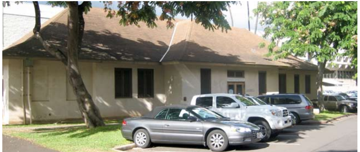
Fig 5.118: Building 37 Main Façade and Entry, 2007
