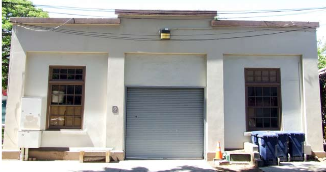
Fig 5.72: Engineering Quad façade with 'roll-up' door. 2007
