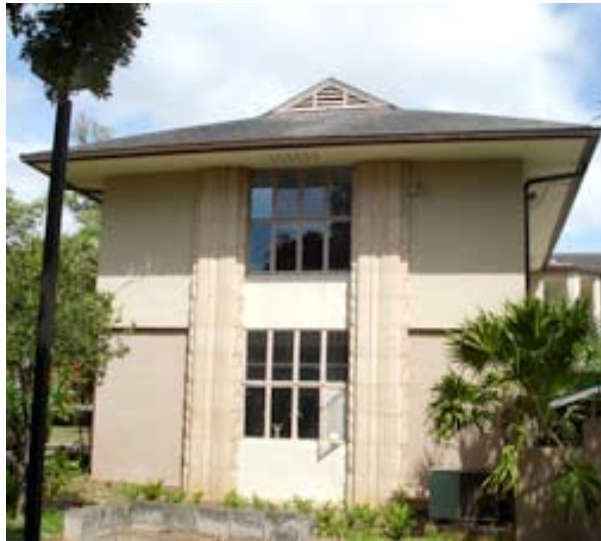
Fig 5.76: Hemenway Hall Western Facade, 2007
