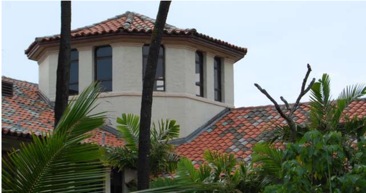
Fig 7.25: Clay Tile Roof Detail at Wist Hall, 2008
