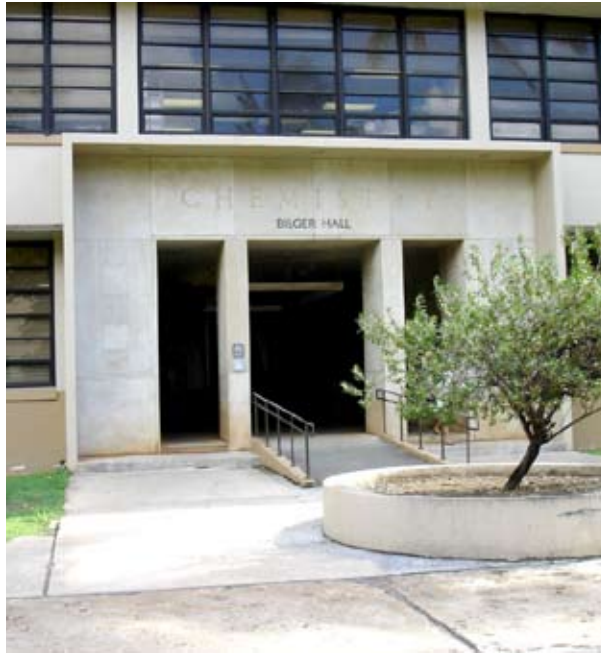
Fig 5.123: Bilger Hall Entry, 2007
