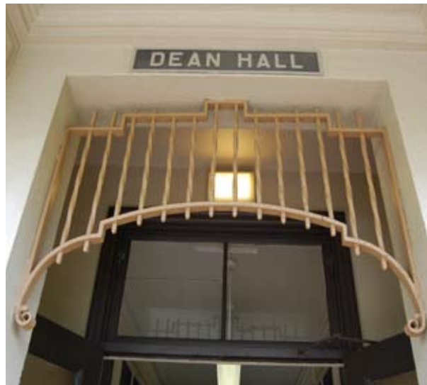
Fig 7.21: Wrought Iron Grill Detail at Dean Hall, 2008
