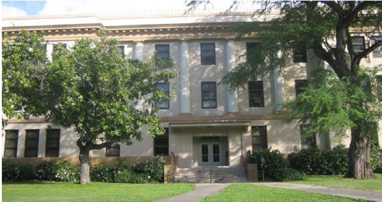
Fig 5.58: Crawford Hall Entry, 2007
