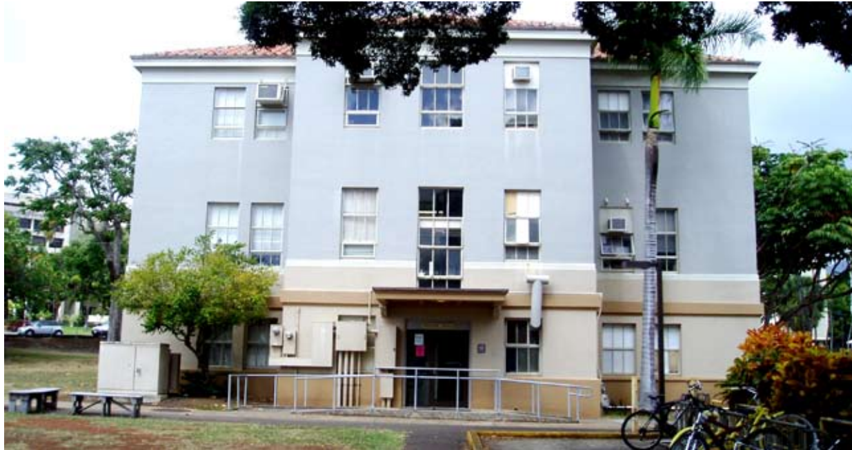
Fig 5.66: Miller Hall Rear Façade, 2007
