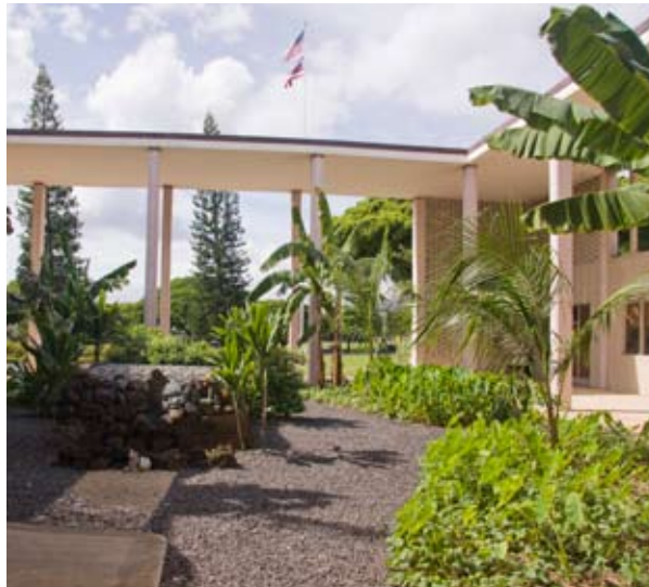
Fig 6.5: Bachman Hall Courtyard, 2008
