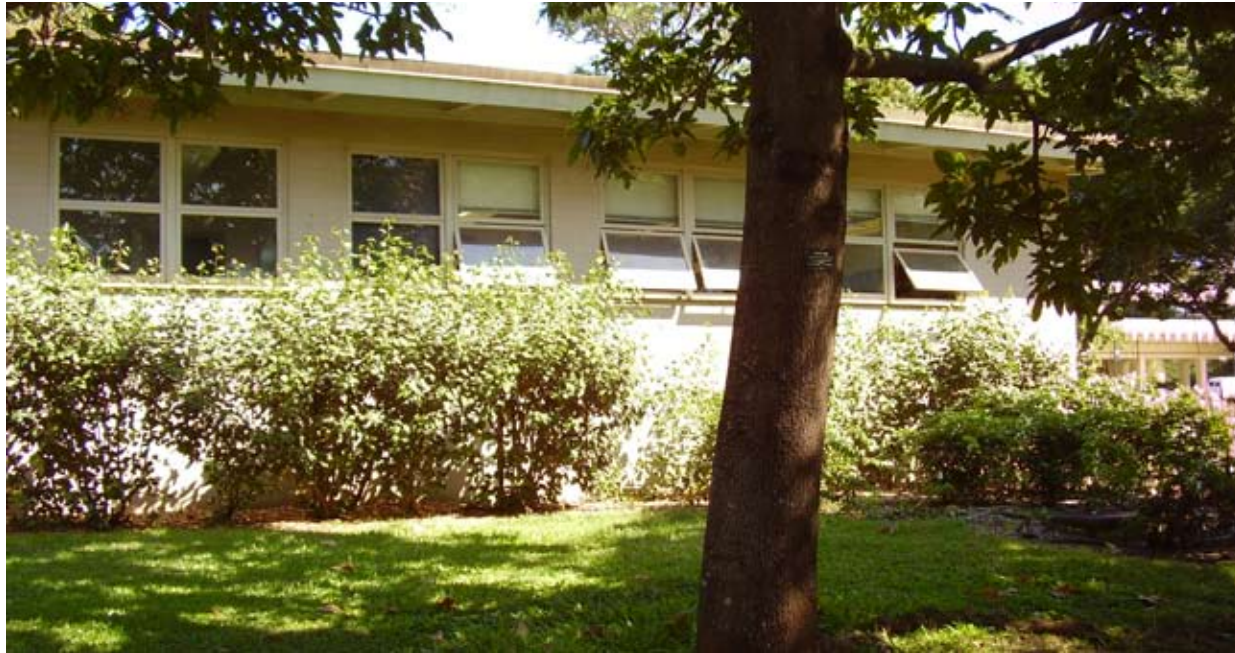
Fig 5.112: Henke southern façade, 2007
