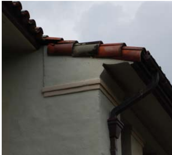
Fig 7.24: Clay Tile Roof Detail at Wist Hall, 2008
