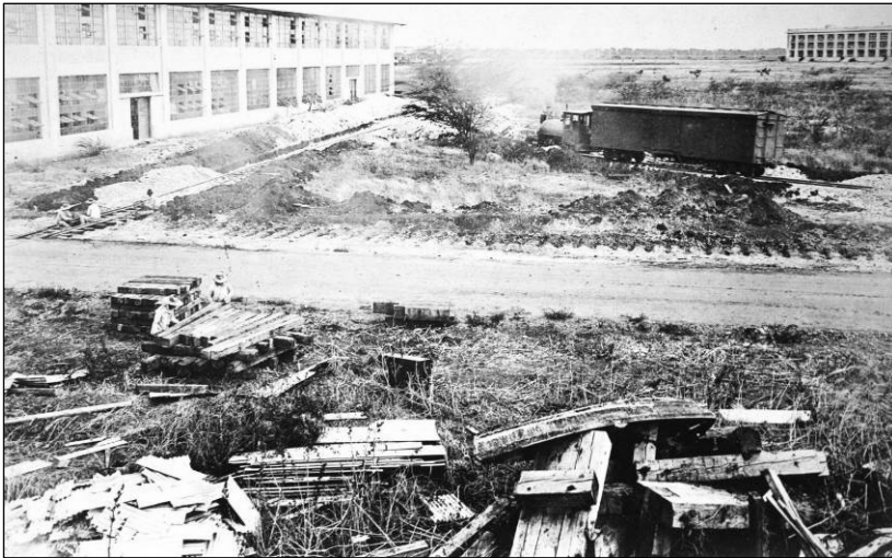
Figure 29. Railroad tracks near Fac. 14, Pattern Shop (left) on Port Royal Street, former Second Street, 6 October 1916. View looking southeast. Record Group 71, NARA.
