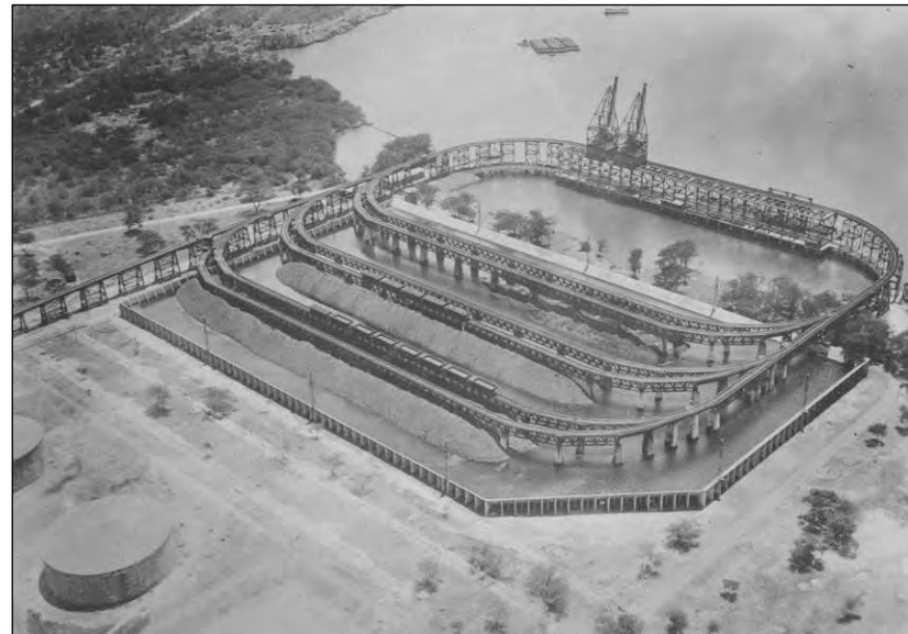
Figure 21. The coaling wharf as seen from Radio Tower No. 1, 18 August 1919. Hawaiian Railway Society Collection.
