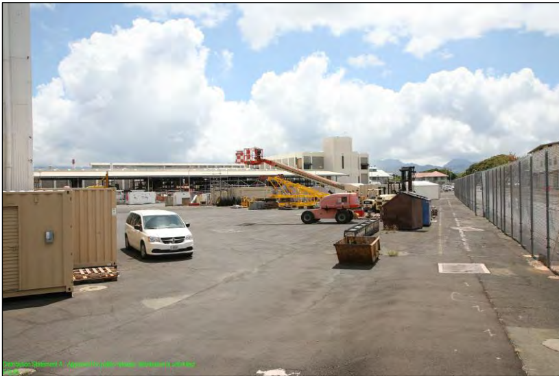
Figure 172. Survey Area 20, looking northeast along Central Avenue.
