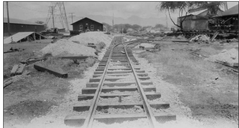
Figure 56. Ballast work on nearly completed trackage. View taken from Second Street looking west, 2 June 1928. Record Group 71, National Archives and Records Administration.
