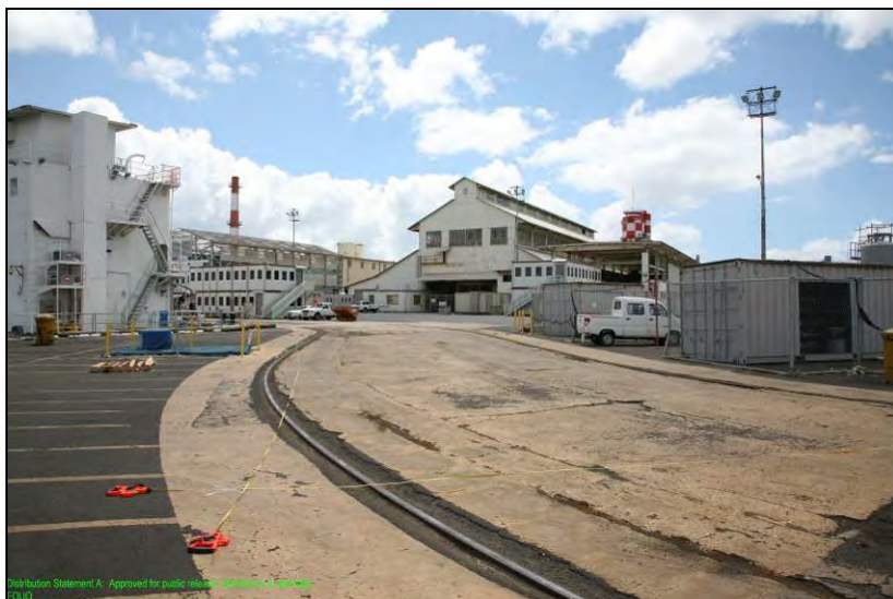
Figure 133. Survey Area 11 looking east across crane rails toward Fac. 5.
