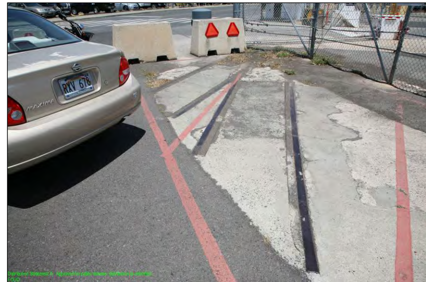
Figure 167. Feature 18.6, looking southeast from southeast corner of Area 18.
