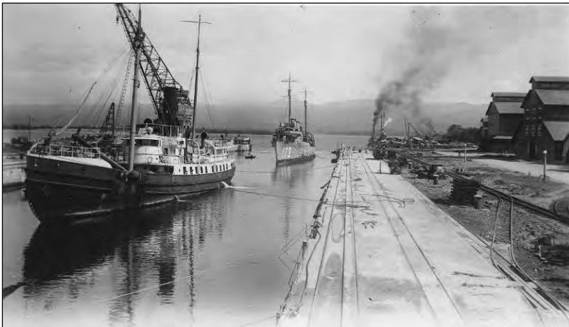
Figure 45. The completed Dry Dock No. 1 with rail access, 9 February 1921, view looking north. Record group 71, NARA.
