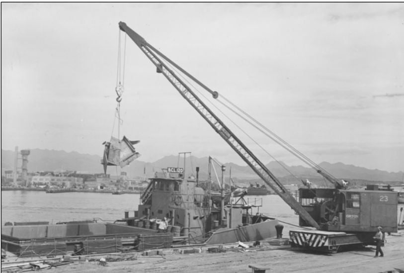
Figure 67. A railroad crane loading scrap metal onto an Army barge, 18 January 1943. Hawaiian Railway Society Collection.
