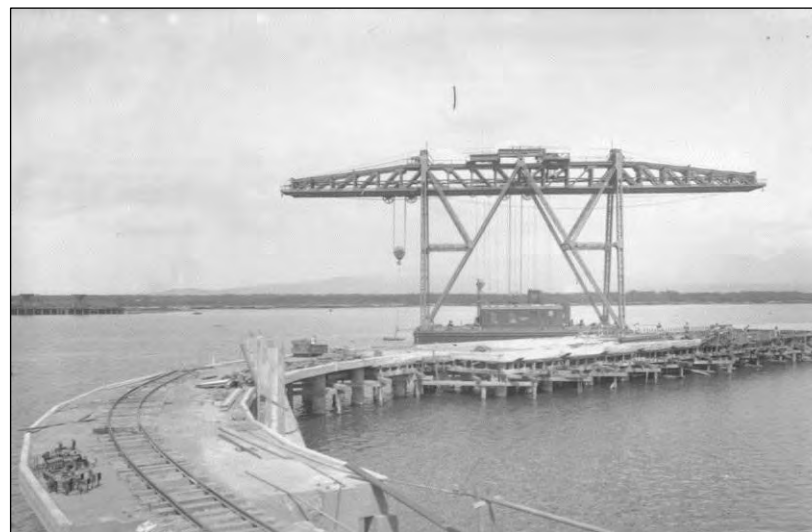
Figure 19. The construction of the Coaling Wharf and construction crane at Pearl Harbor, May 1914. Hawaiian Railway Society Collection.
