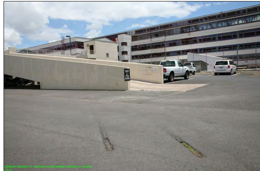
Figure 105. Feature 5.3, looking northwest across Paul Hamilton Avenue with Fac. 155 in the background.
