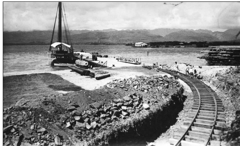
Figure 38. Railroad track turnout at Torpedo Boat Pier No. 3, 6 August 1918. Record Group 71, National Archives and Records Administration.
