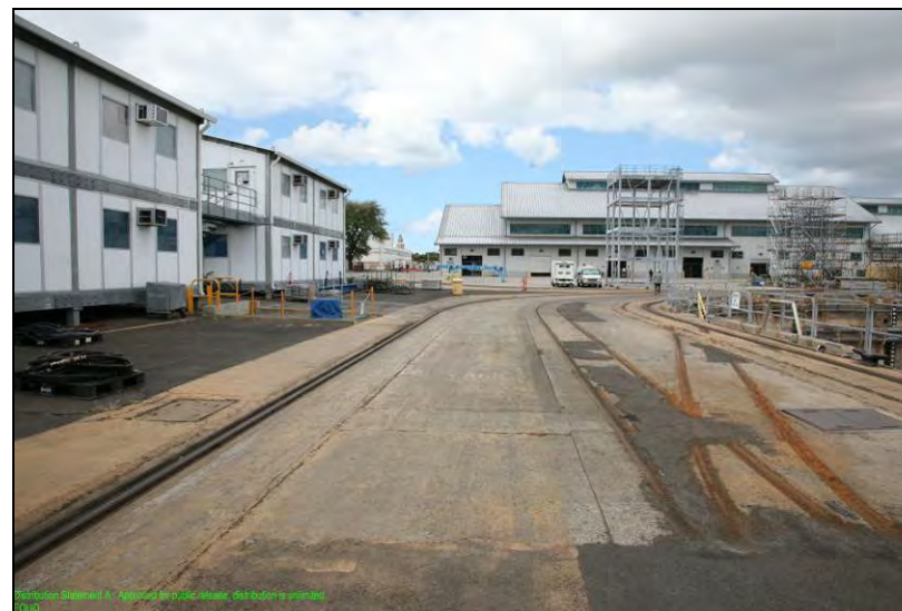
Figure 136. Survey Area 12, looking southwest along the east wall of Dry Dock No.1.
