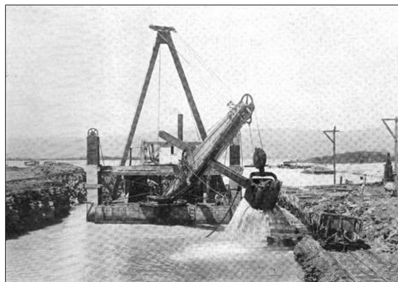
Figure 14. The dredge Governor at work on the Dry Dock during the first half of 1910. At right, the dump cars of the contractors are seen. Taylor 1910.
