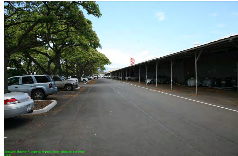
Figure 96. Feature 3.6 and 3.7 looking northwest along south elevation of Fac. 159.
