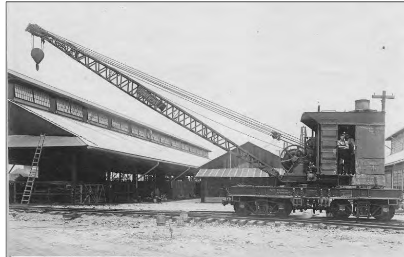
Figure 24. The first locomotive train at Pearl Harbor (pictured) was manufactured in Cleveland, Ohio, by the Brown Hoisting Company. Photo dated 1 May 1913. Record Group 71, National Archives and Records Administration.
