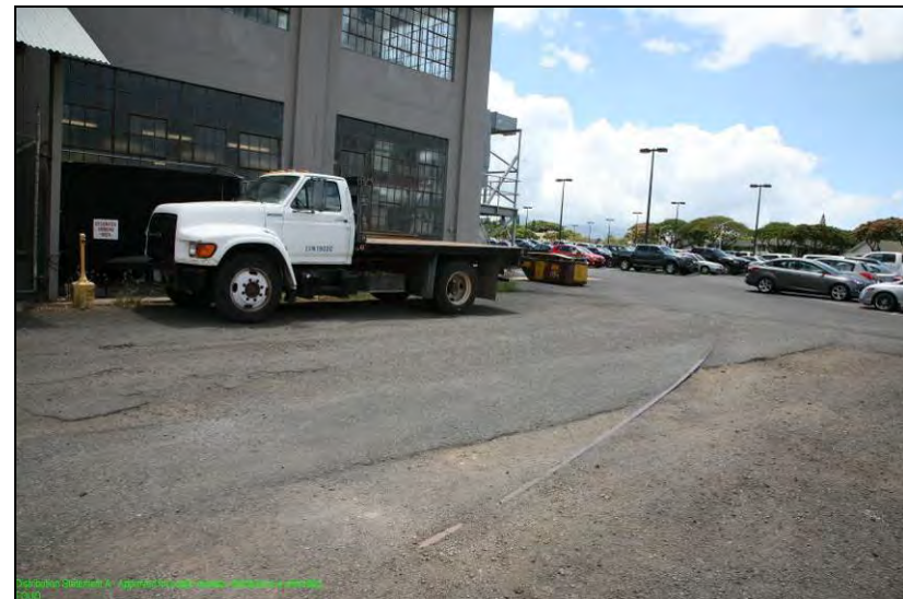
Figure 111. Feature 6.2, looking east at southeast corner of Fac. 14.
