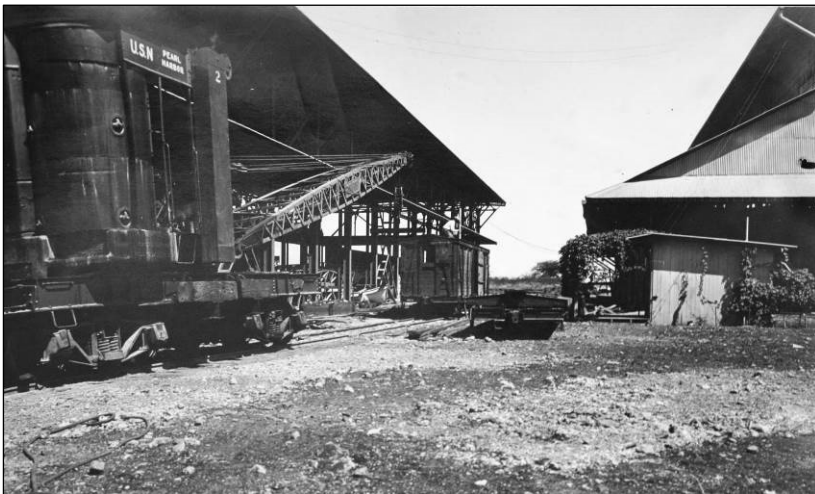
Figure 30. Railroad track between the Fac. 6, Foundry (right) and Fac. 12, Boat Storehouse (left), 11 September 1917. One of the Station's locomotive cranes is visible at left. View looking southeast.
