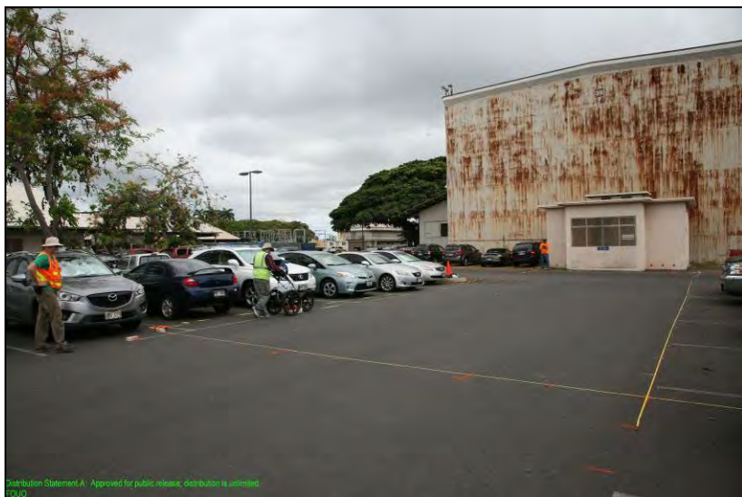
Figure 91. Survey Area 3, looking west at east elevation of Fac. 39, Heavy Storage.
