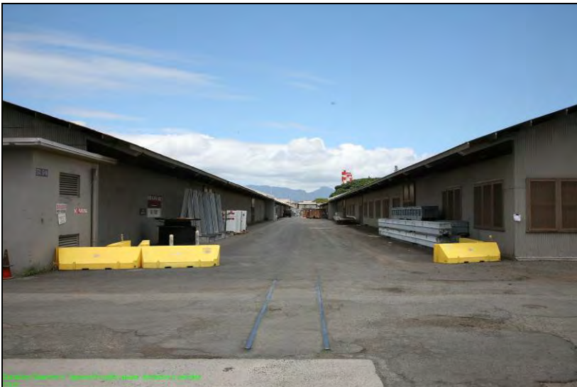
Figure 95. Feature 3.5, looking northwest between Fac. 159 and Fac. 158.
