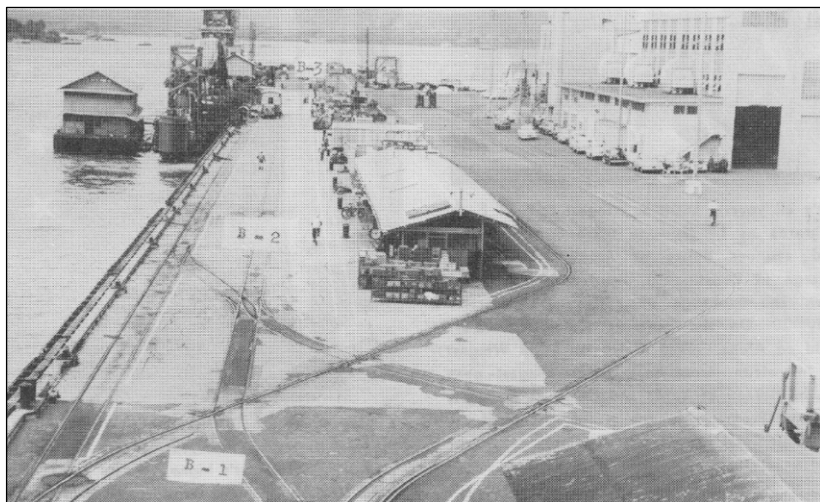
Figure 79. Crane trackage near Berth B-1 and B-2, 1010 Dock, View looking north with Fac. 67 and 67B to right, 1964. Record Group 5, Seabee Museum Archives.
