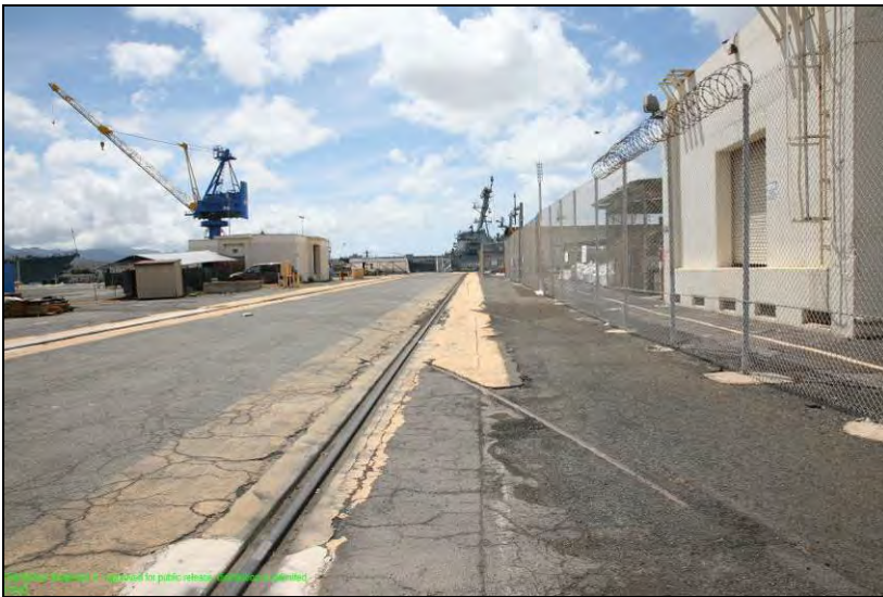
Figure 148. Survey Area 15, at head of Repair Basins looking east with Fac. S100 to right.
