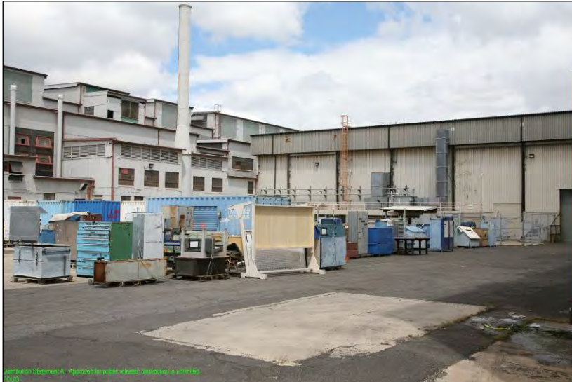
Figure 153. Survey Area 16, looking west from northeast corner of survey area.
