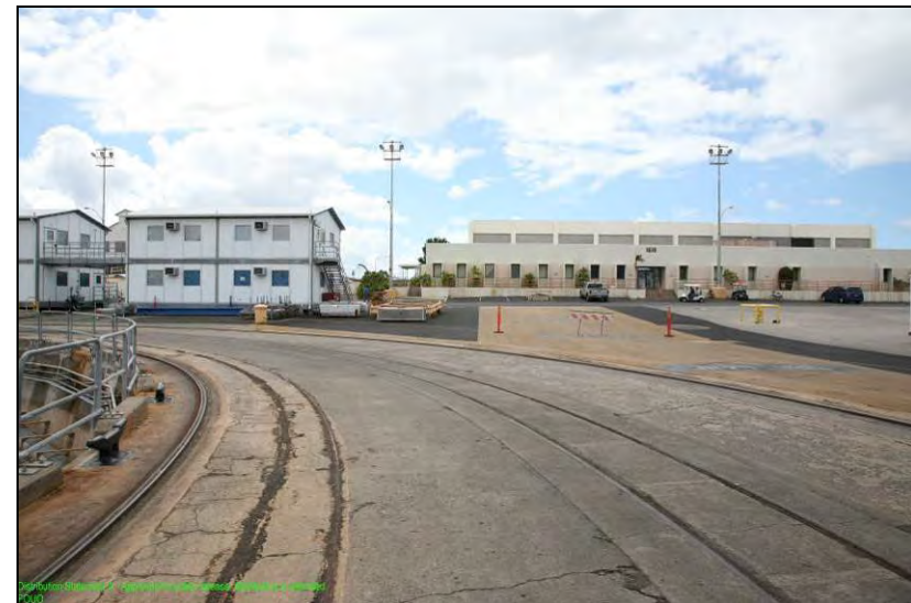
Figure 140. Survey Area 13, looking east toward Fac. 1670 at head of Dry Dock No. 1.
