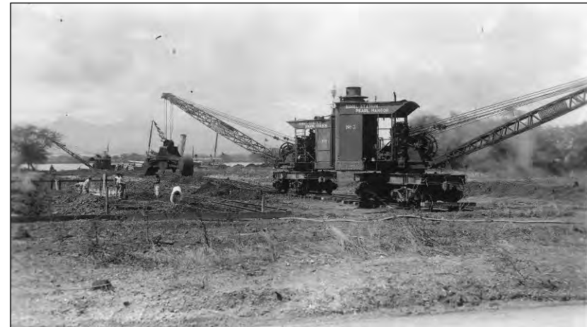
Figure 49. Locomotive cranes employed in the excavation of the foundation for Machine Shop (Building 67), 4 October 1921. Records Group 71, National Archives and Records Administration.
