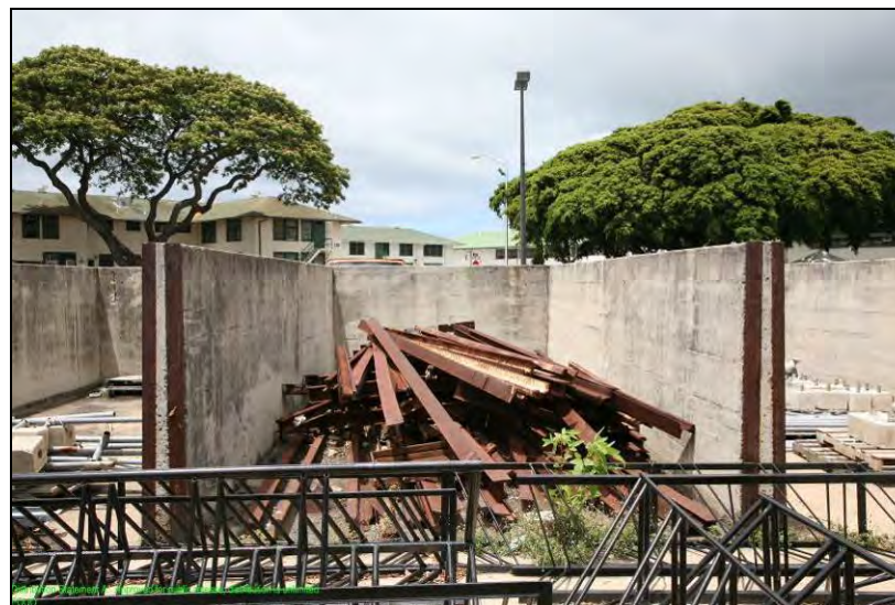
Figure 114. Removed Rails from Parking Lot F former Navy Yard Depot and stored in former ore ingot bins near Survey Area 6, looking south.
