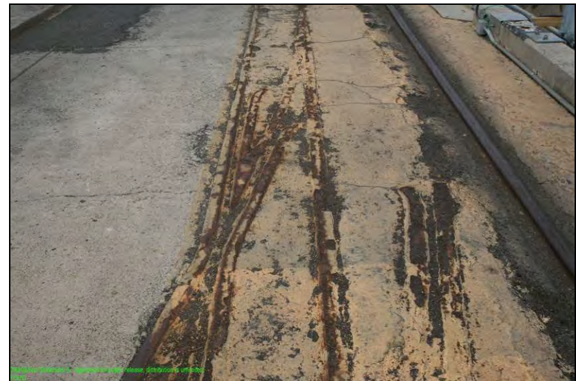
Figure 135. Feature 11.8, looking southwest at narrow gauge rails running parallel to crane rails at Dry Dock No. 1.
