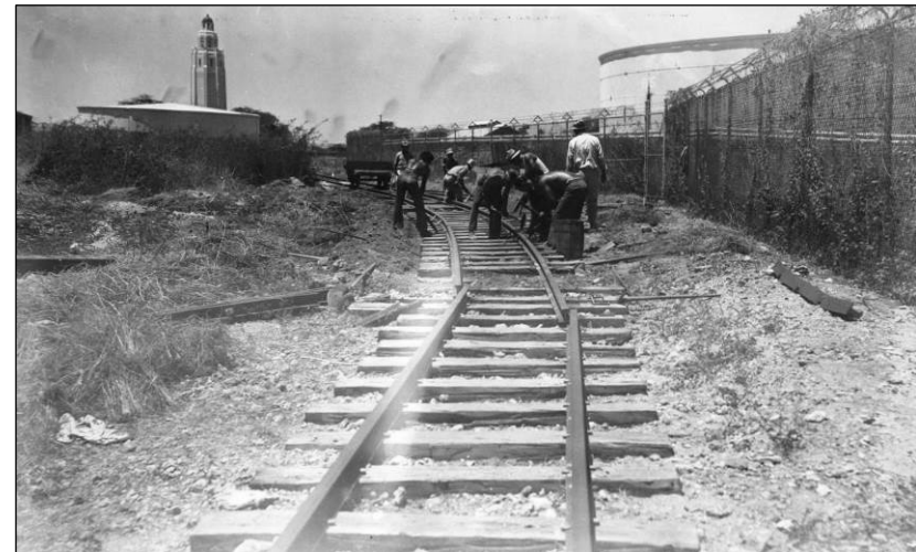
Figure 59. New railroad tie installation along the spur track that lead to the Mixing Plant, 1 August 1938. Record Group 71, National Archives and Records Administration.
