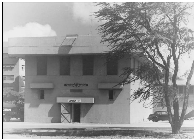
Figure 77. Railroad tracks in the vicinity of Fac. 41, Main Office of the Power Plant at Navy Yard, Pearl Harbor, October 1945. Record Group 5, Seabee Museum Archives.
