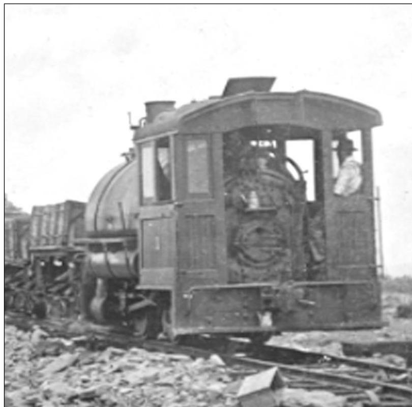
Figure 12. Locomotive #1, built by H. K. Porter Company of Pittsburg, Pennsylvania, at work at the Navy Yard in 1917. Hawaiian Railway Society Collection.
