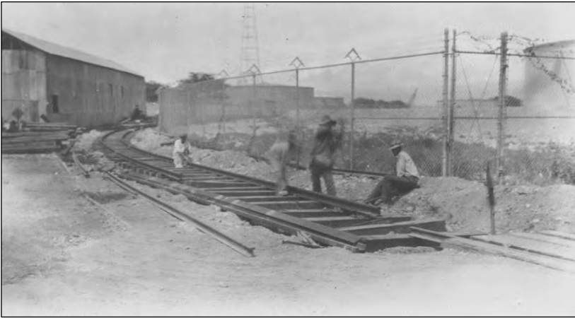
Figure 57. Replacement of railway track, 20 September 1928. View looking northeast from South Avenue. Hawaiian Railway Society.
