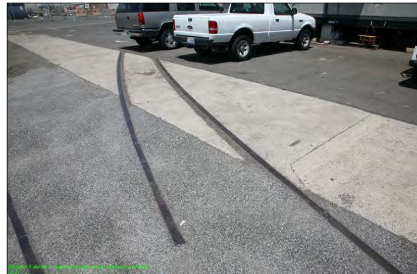
Figure 162. Feature 17.3, looking north.
