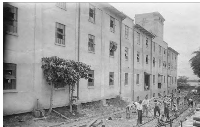
Figure 39. Relocation of trackage along Building 9A (a Storehouse), 6 June 1918. View facing southwest. Record Group 71, National Archives and Records Administration.
