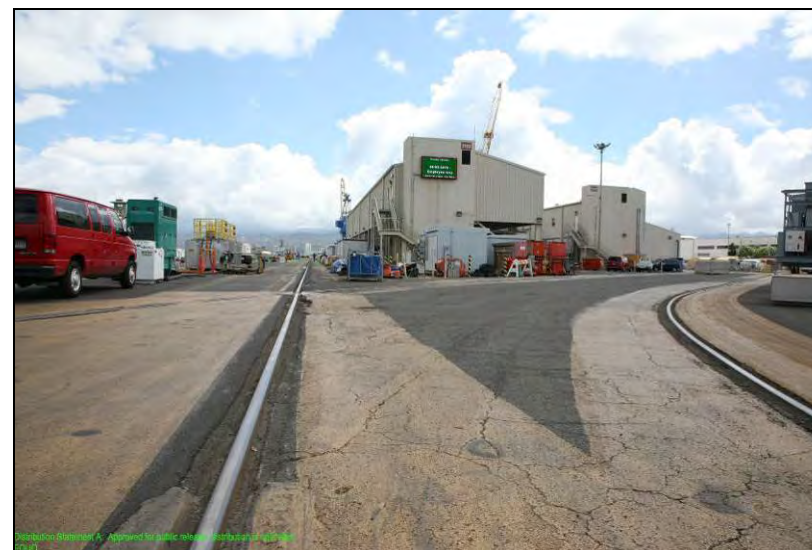
Figure 144. Survey Area 14, looking northeast between Dry Dock No. 1 and Dry Dock No. 2.
