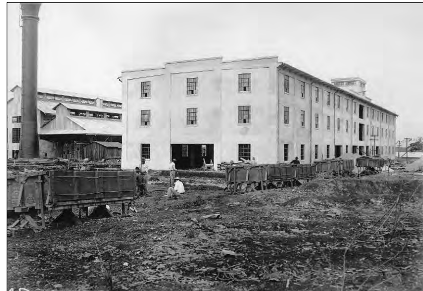
Figure 23. Manually operated Dump Cars employed in work near Fac. 9, General Storehouse. View looking west. 1 April 1913. Record Group 71, NARA.
