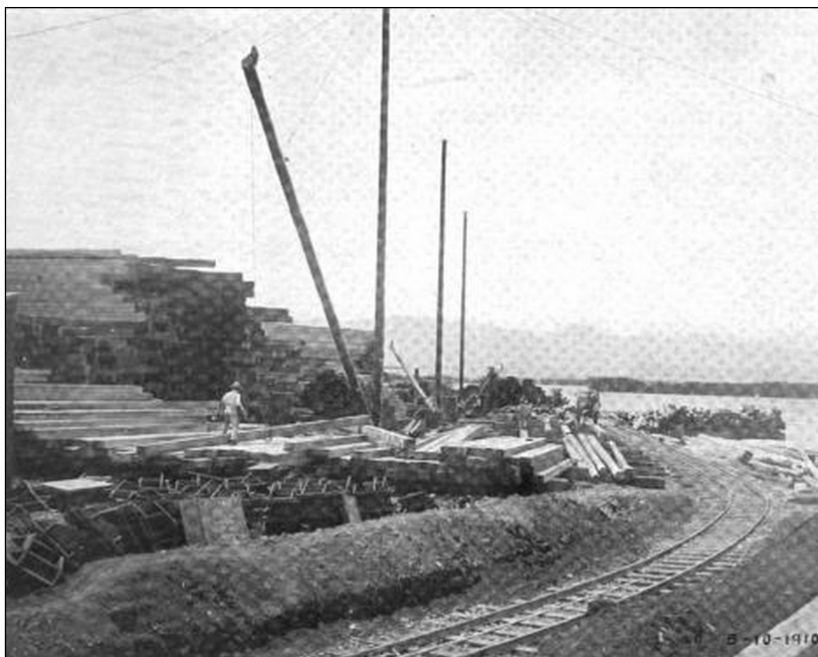
Figure 15. The temporary Framing Yard for the Dry Dock crib is featured in this May 1910 photograph. At right, the temporary railroad track of the developing Navy Yard is seen. Taylor 1910.
