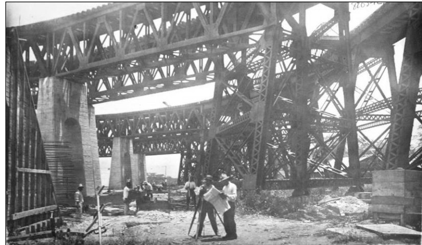
Figure 20. Work underway on Coaling Wharf, 6 May 1918. Record Group 71, National Archives and Records Administration.
