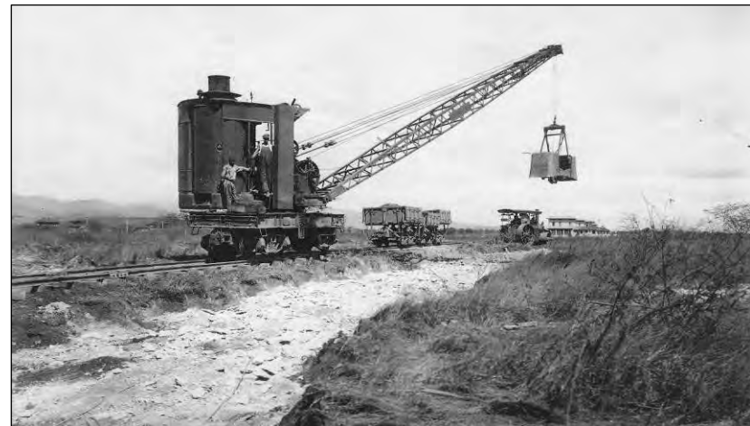
Figure 25. A locomotive crane and dump cars employed in excavation for construction of a Lumber Shed, September 1914. Record Group 71, National Archives and Records Administration.
