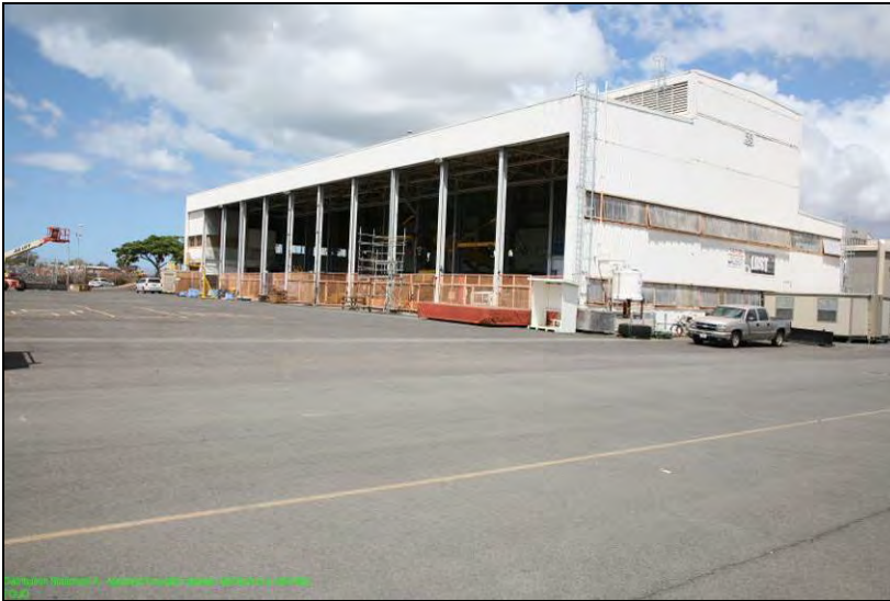
Figure 174. Building 58 (Transportation Building), former Engine House, looking southwest from Ingersoll Avenue.
