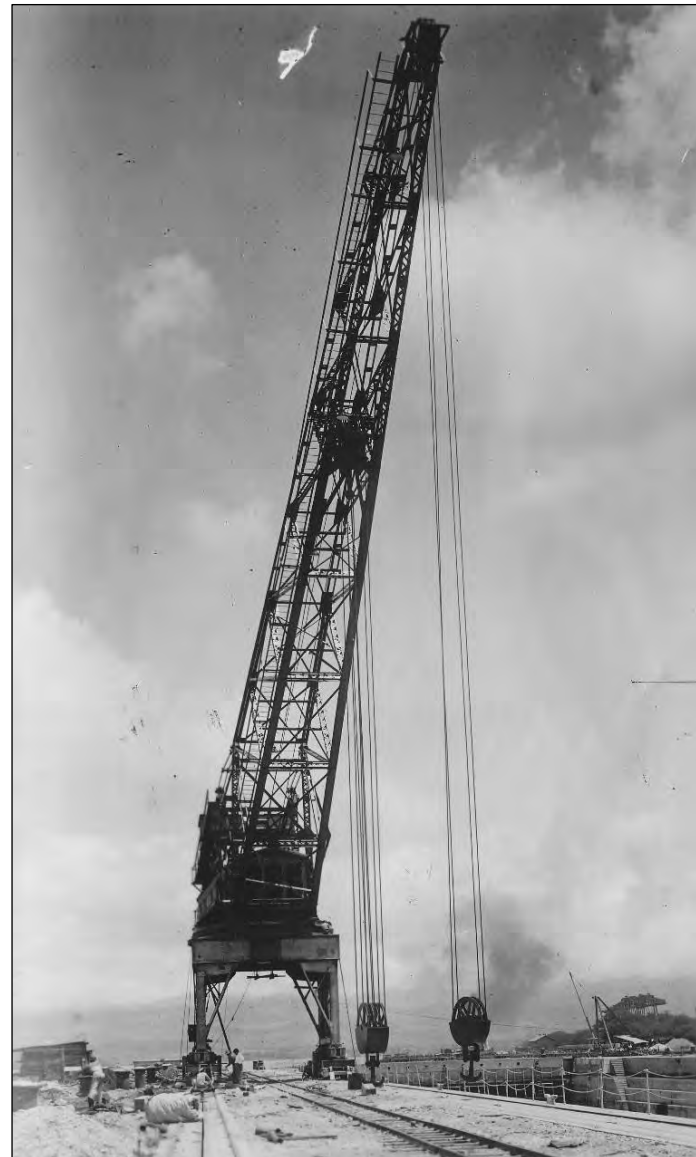
Figure 74. 50-ton electric locomotive crane for use at the Dry Dock. 20 August 1943. Record Group 71, National Archives and Records Administration.
