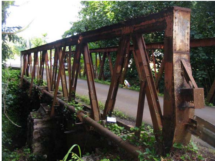
Opaekaa Bridge (1900) County of Kauai: 007420151142001
