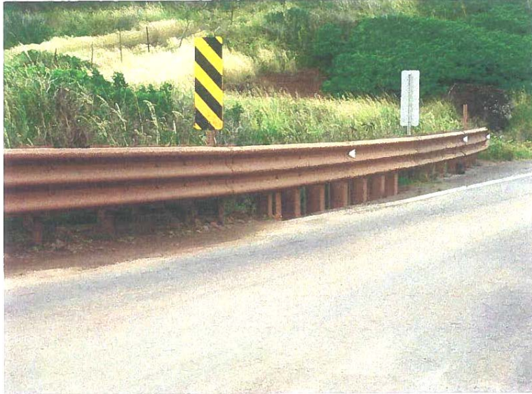
Anakaluahine Stream Bridge No.69 (1924) Maui State: 009000300303899
