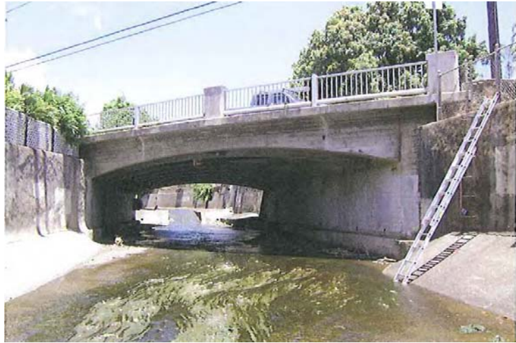
Palolo Stream Bridge County of Honolulu: 003083531400155
