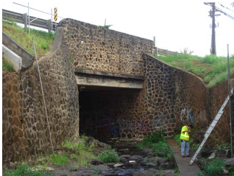
Kawa Stream Bridge (1939) Oahu State: 003063001400065
