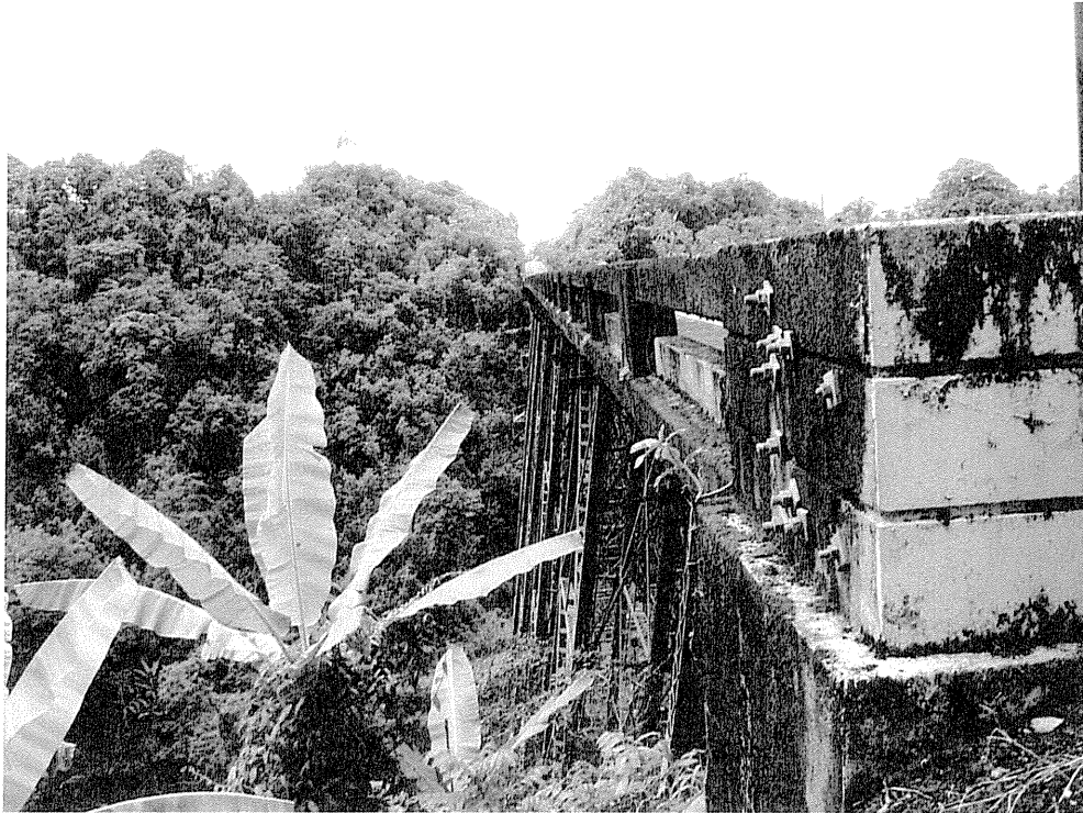
Photo #3: Trestle Substructure
