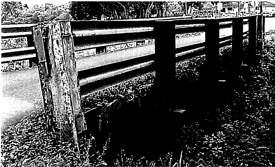
VIEW FROM NORTHWEST SIDE
