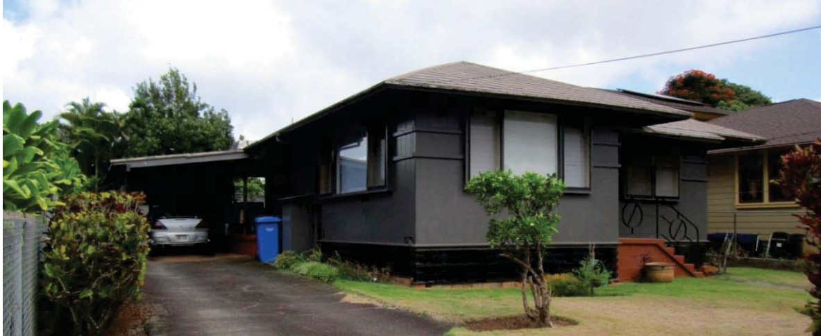
14 Circle Drive, built 1951
