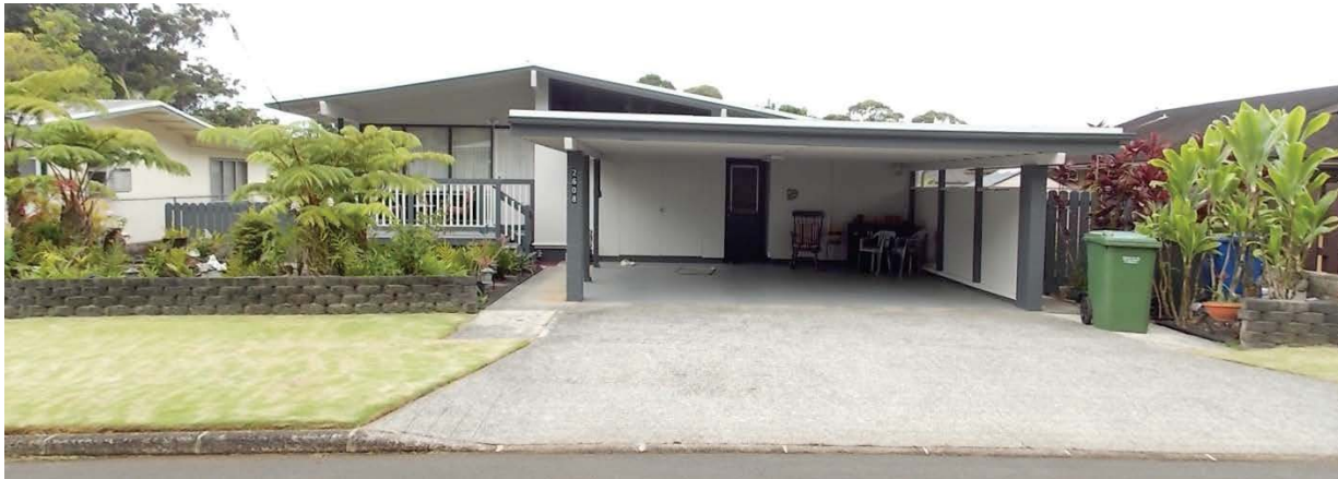
2608 California Avenue, built 1964.
