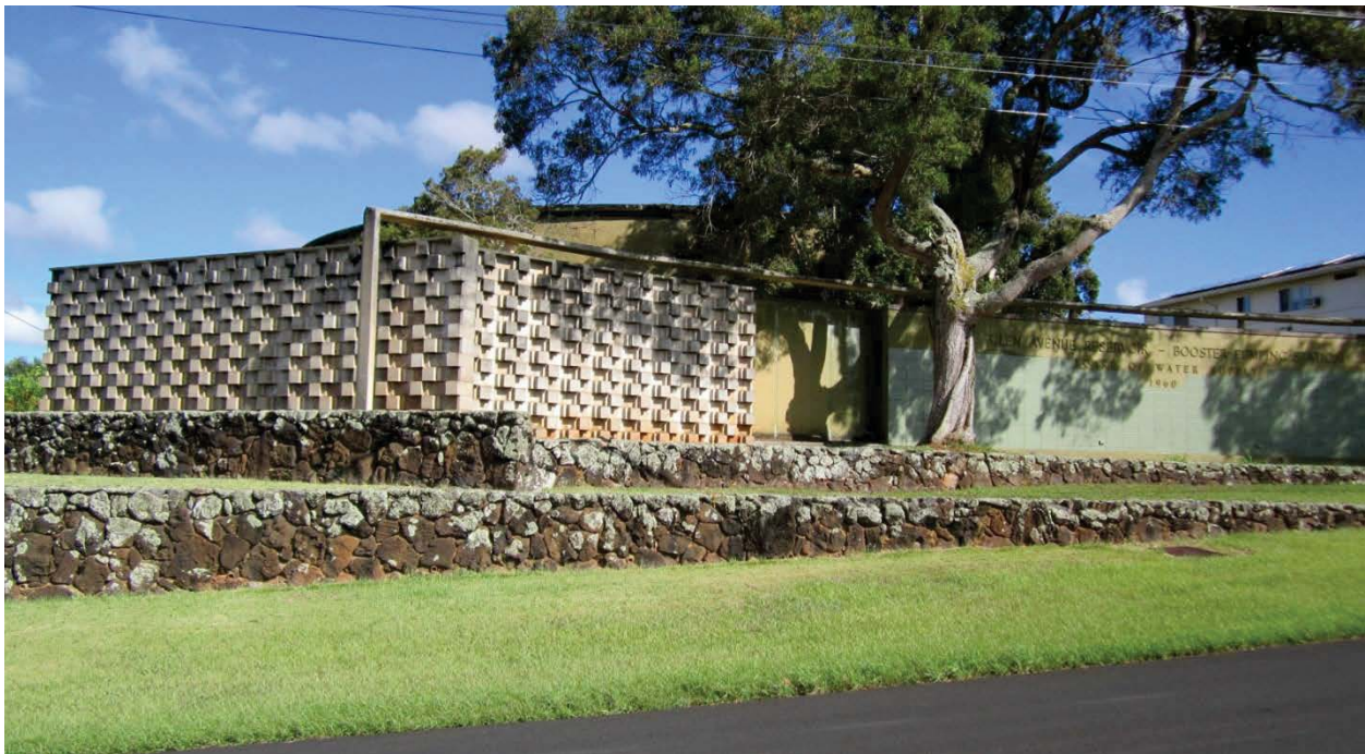
1610 Glen Avenue - Water Tower, built 1960
