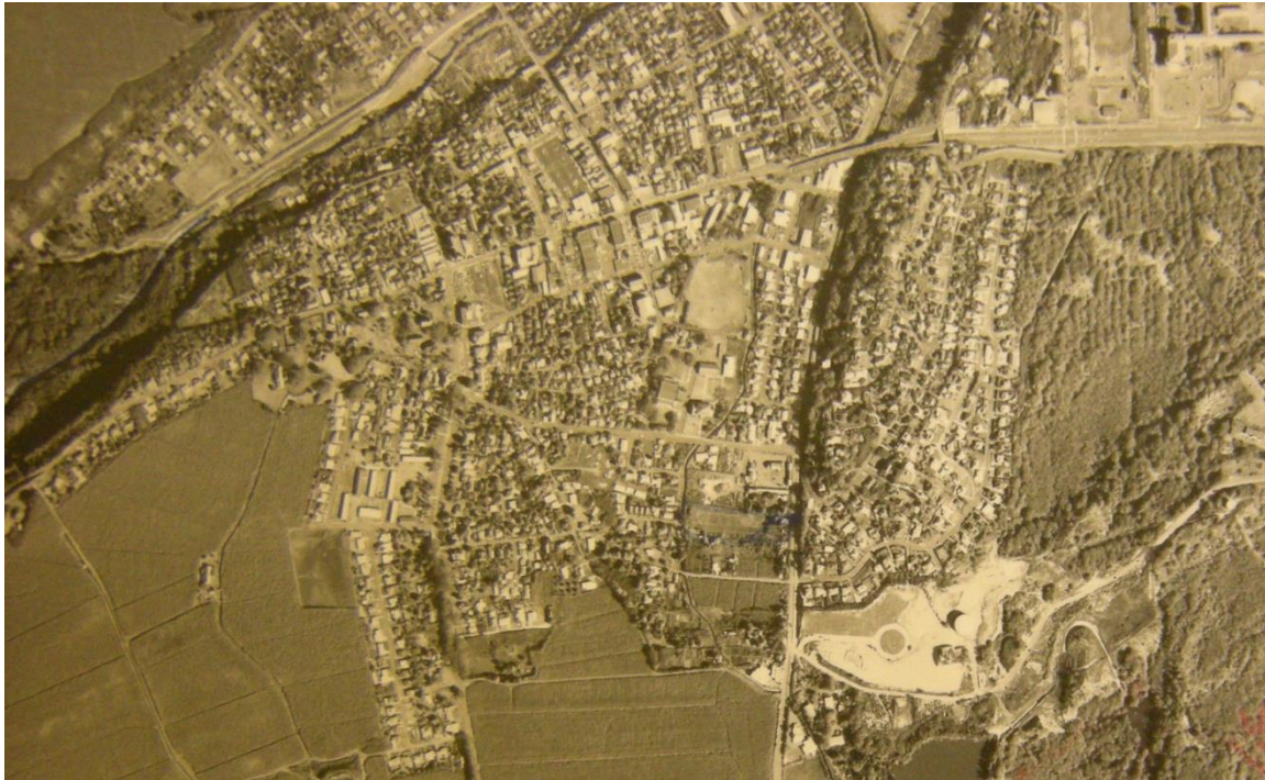
Figure 42: 1965 aerial photograph showing further development of Wailuku, as well as Sand Hills.
