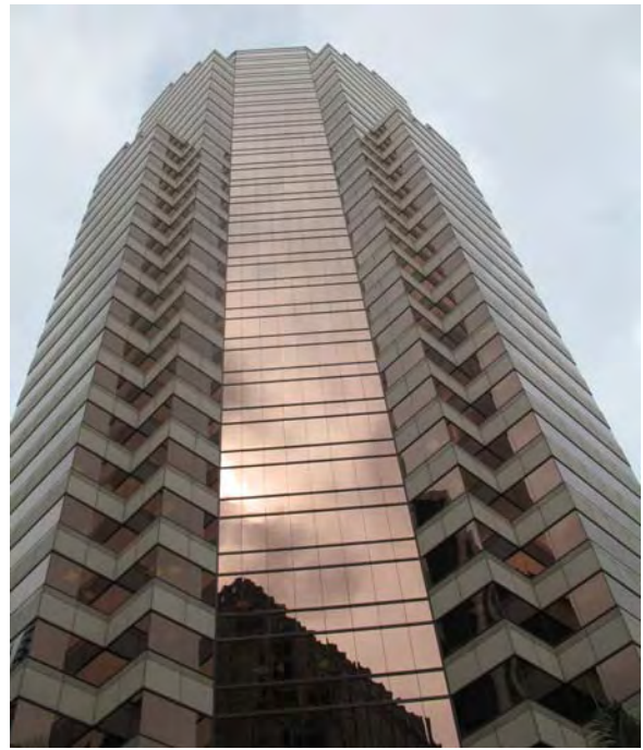
4-132 1100 Alakea David Stringer, 1995, 1100 Alakea St. (2006)
