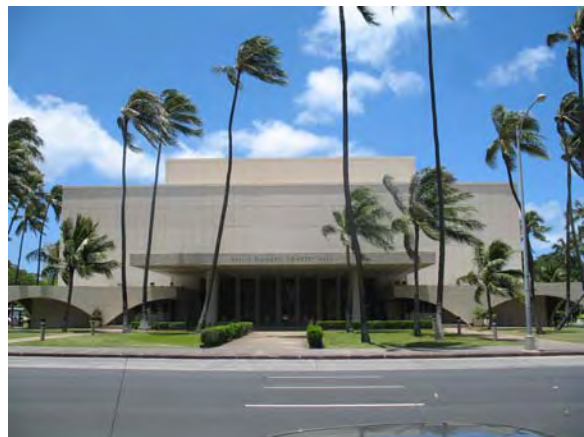
4-126 Neal Blaisdell Center Merrill, Simms, Roehrig, 1964, 777 Ward Ave. (2011)
