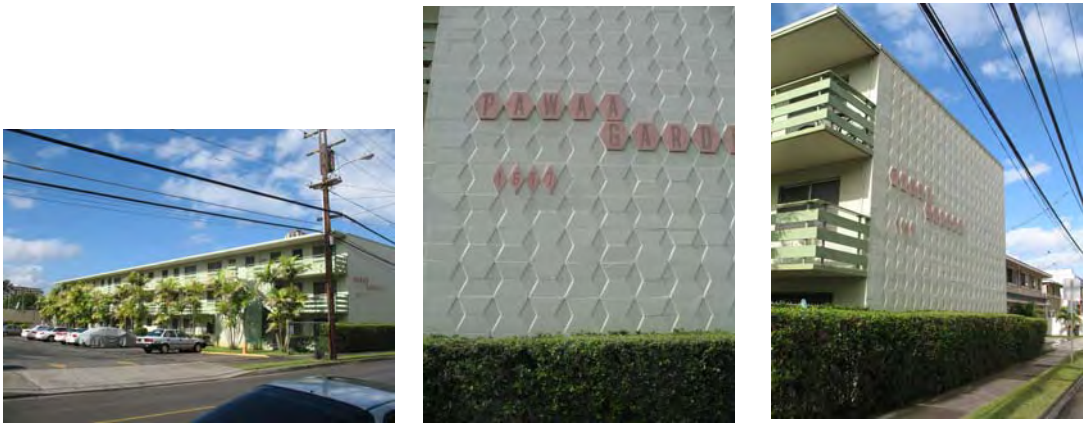
Two buildings echoing each other across a parking lot. Distinctive end wall using an uncommon patterned concrete block. Wood railings affixed to pipes add to the special appearance of the buildings.
