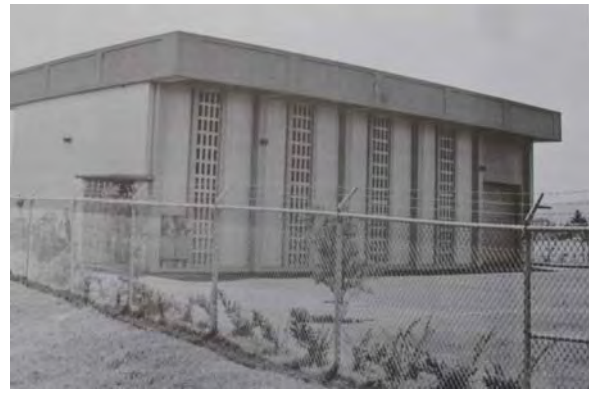
4-103 Waimalu Pump Station (City and County of Honolulu Public Works Annual Report)
