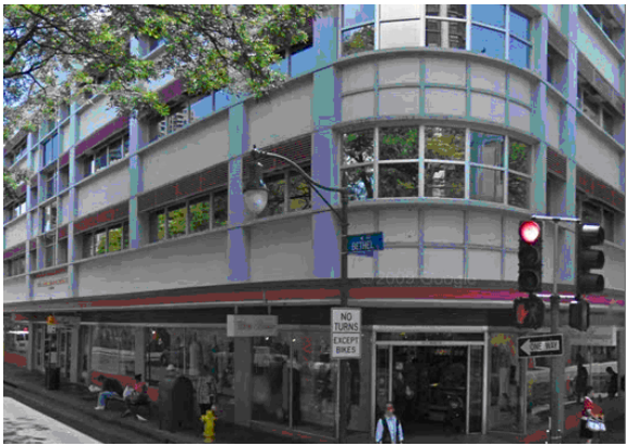
4-11 Plumbers and Fitters Union Building 1955, 1107 Bethel St. http://maps.google.com/maps?q=1109+Bethel+Street,++Honolulu,+HI+96813
