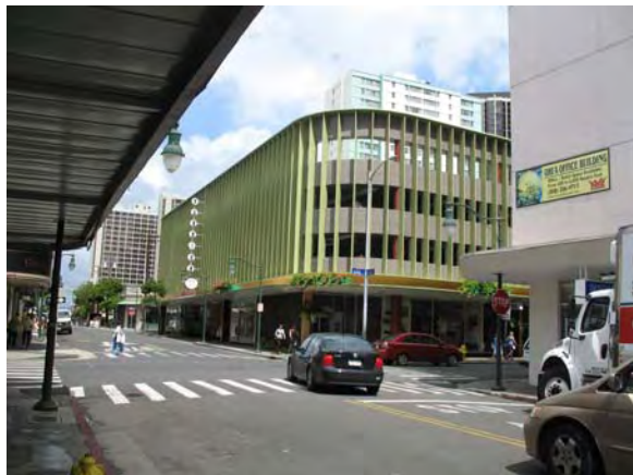
4-100 Marks Garage 1159 Nuuanu Ave. (2011)
