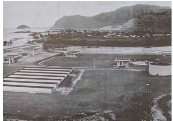
4-104 Wainae Sewage Plant (City and County of Honolulu Public Works Annual Report)
