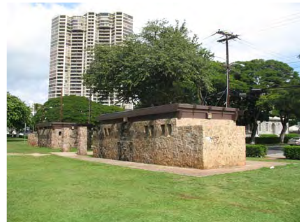
4-113 Thomas Square Comfort Station Tom Wells, 1966, 925 S. Beretania St. (2011)
