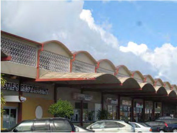
4-36 Waimalu Shopping Center 98-042 Kamehameha Hwy. (2011)
