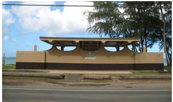
4-117 Punaluu Beach Park Comfort Station Richard Iwanaga, 1968, 3059 Ualena St. (2011)
