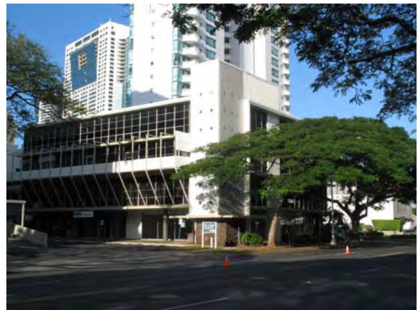
4-5 Seaboard Finance Building Milton Akiyama, 1956, 1349 Kapiolani Blvd. (2011)
