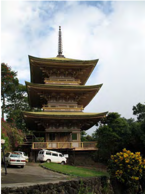
3-12 Concrete Pagoda Robert Katsuyoshi, 1966, 22 Craigsid Pl. (2006)
