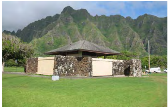
4-115 Kualoa Beach Park Restroom James Sato, 1973, 49-479 Kamehameha Hwy. (2011)
