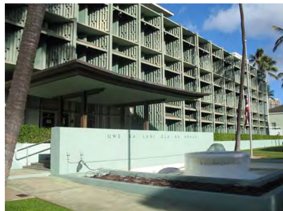
3-5 Board of Water Supply Administration Building Hart Wood, 1958, 630 S. Beretania St. (2006)
