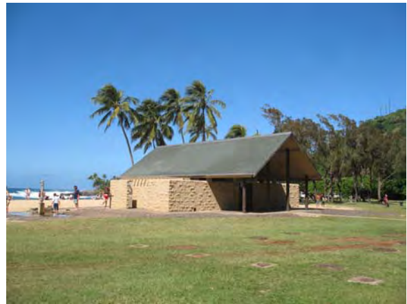
4-67 Waimea Bay Restroom John McAuliffe, 1967, 61-031 Kamehameha Hwy. (2011)
