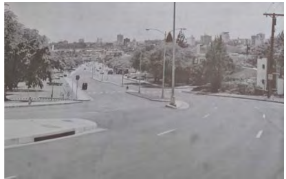
4-97 Newly completed University Ave. (City and County of Honolulu Public Works Annual Report)
