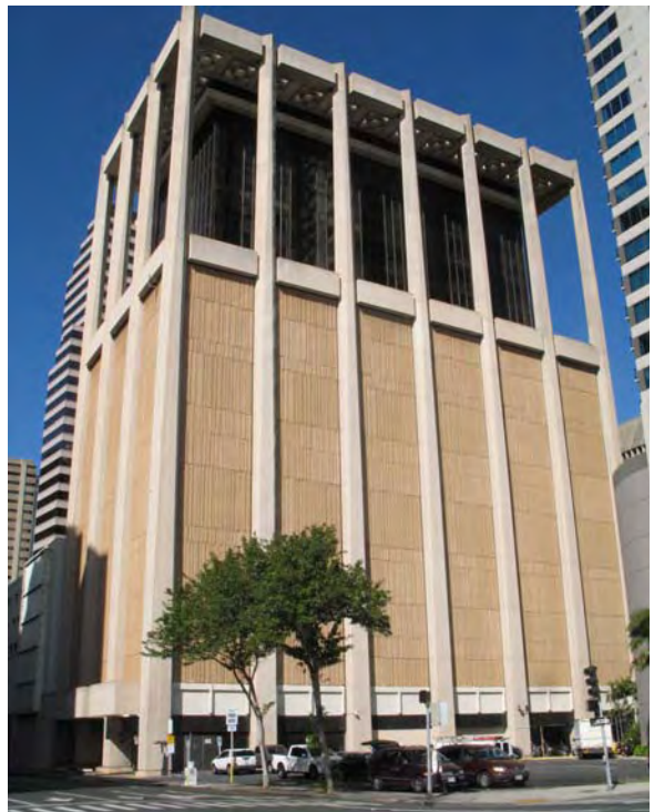
4-124 Hawaiian Telephone Building 1968, Don Chapman, 1177 Bishop Street (2011)
