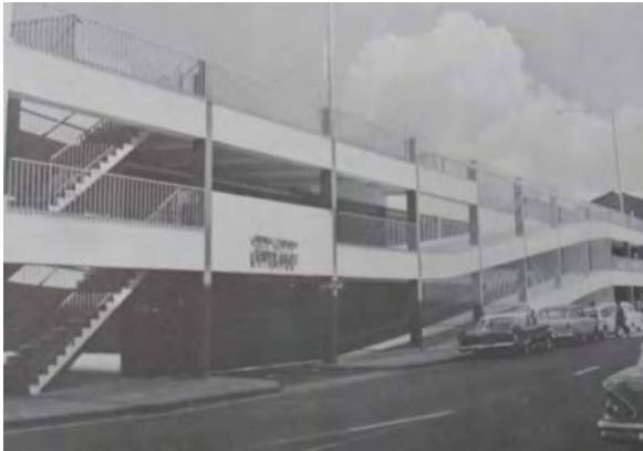
4-99 Double deck Parking Structure, no longer extant (City and County of Honolulu Public Works Annual Report)
