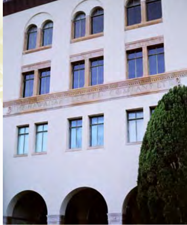
Hawaiian Electric Building
